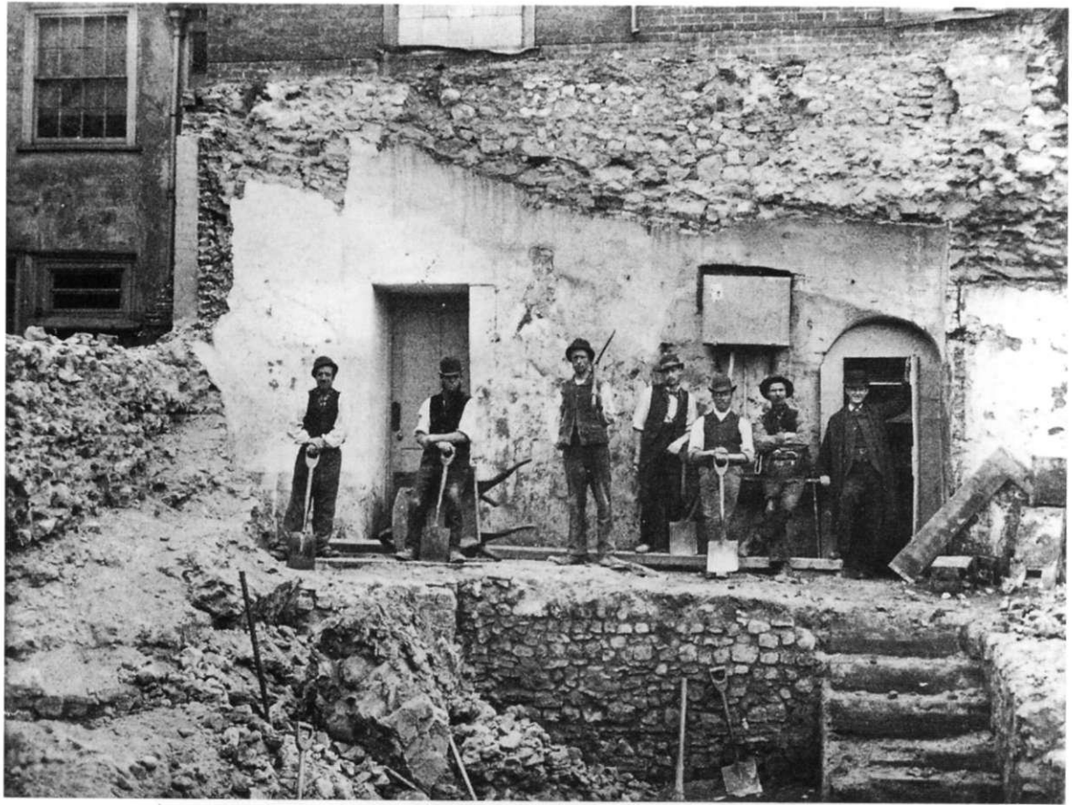
Fig 48 The stone house at Foundry Yard during demolition, looking south from inside basement. Photograph by J C Shenstone
