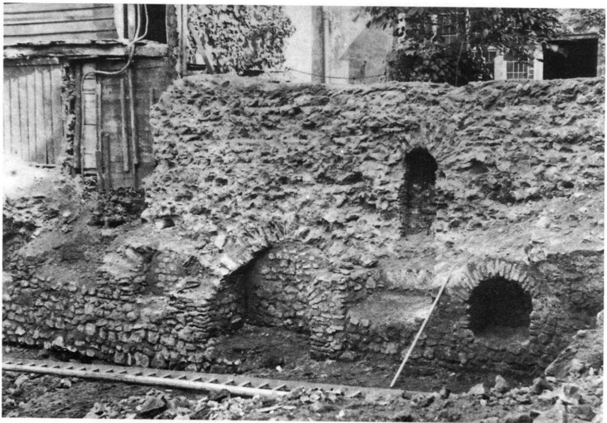
Fig 49 The stone house at Foundry Yard during demolition: eastern wall of basement. Photograph by J C Shenstone
