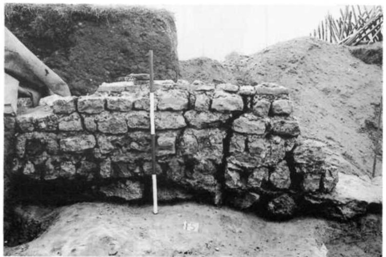
Fig 3.4 Various views of the church walls and foundations. Above left: the south-west corner seen from the south. Note the mortar squeezed out between courses below the original ground level. Above right: the rebuilt west wall seen from the east. Note the subsidence cracks. Below left: the south-west corner seen from the west. Note the severe crack between the original quoin and the rebuilt west wall. Below right: the apse seen from the south-west. [Page 166]
