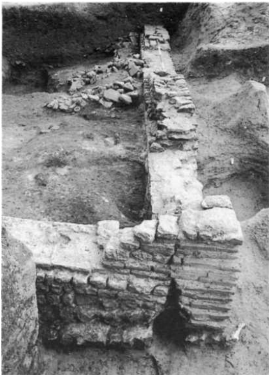
Fig 3.4 Various views of the church walls and foundations. Above left: the south-west corner seen from the south. Note the mortar squeezed out between courses below the original ground level. Above right: the rebuilt west wall seen from the east. Note the subsidence cracks. Below left: the south-west corner seen from the west. Note the severe crack between the original quoin and the rebuilt west wall. Below right: the apse seen from the south-west. [Page 166]
