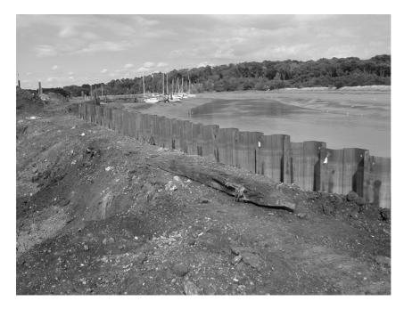
Fig 2 Timber post with new sheet piling to the rear - view north.
