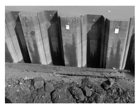
Fig 3 Timber post with new sheet piling behind.
