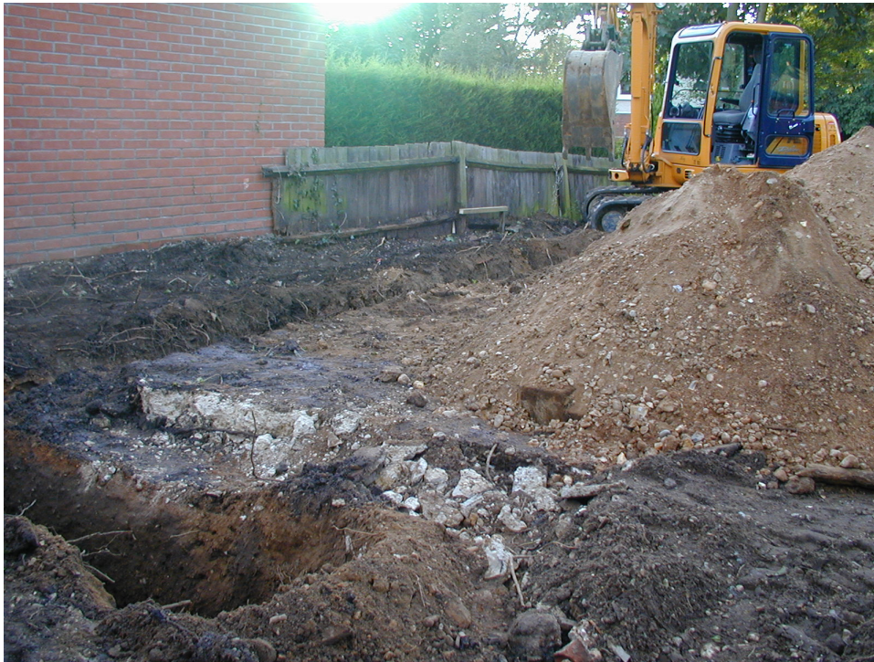
Fig 3 View of foundation trenches looking south-west.
