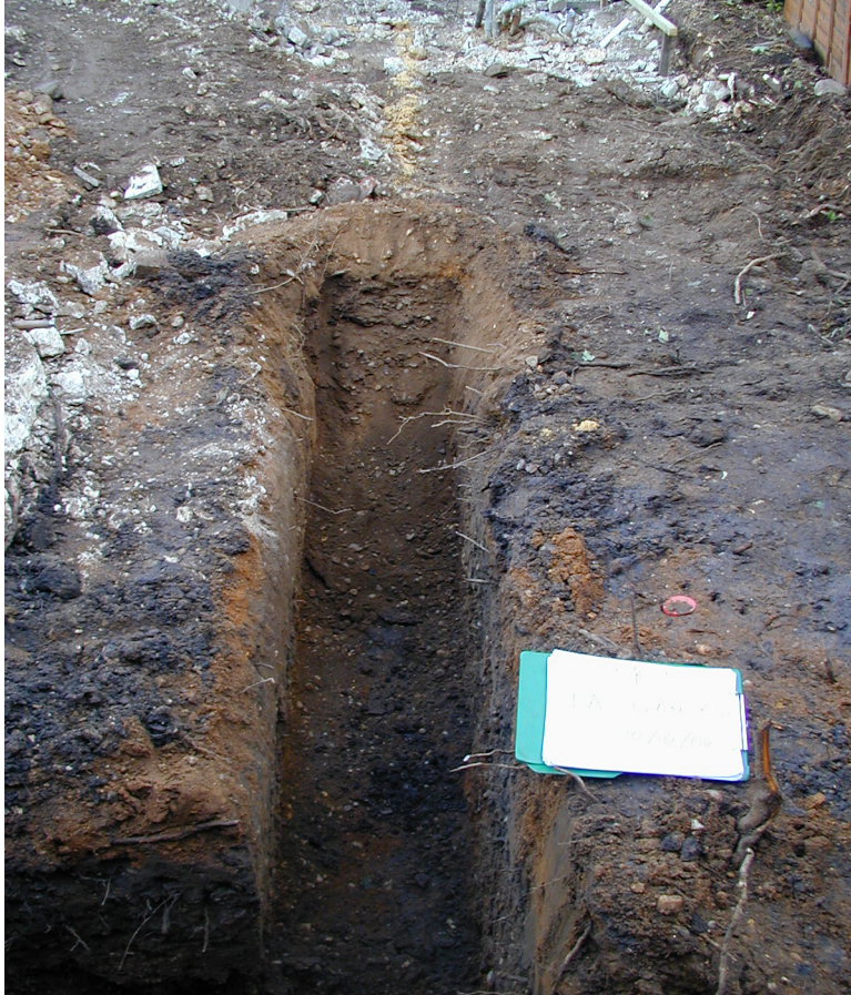
Fig 2 View of foundation trenches looking south.
