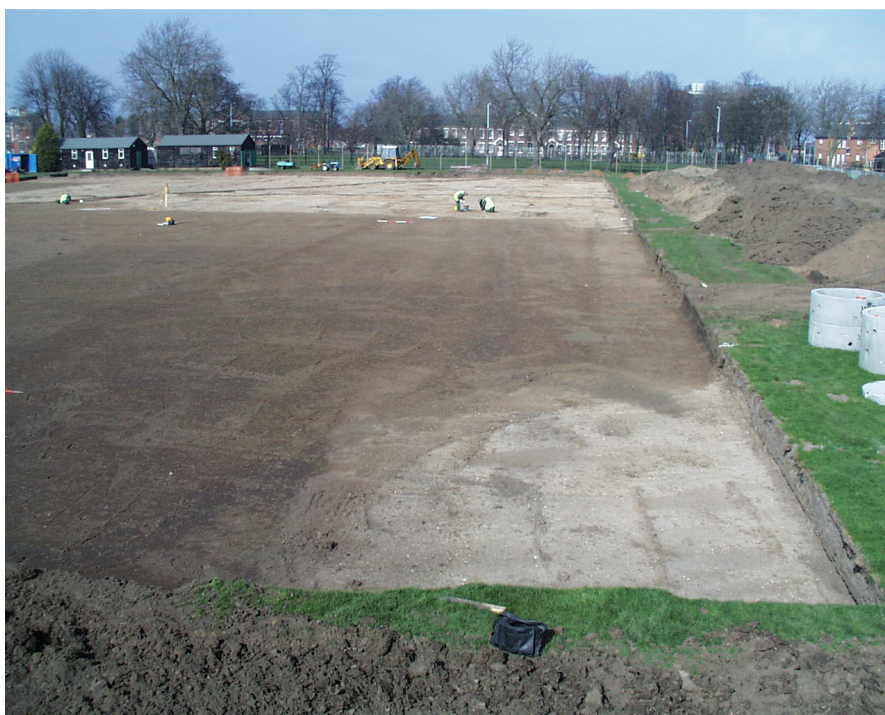
Plate 1 Overall view of the stripped site, view north-west.
