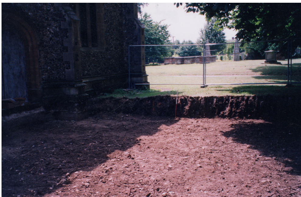
Plate 2 General shot of site after ground-reduction, looking west.
