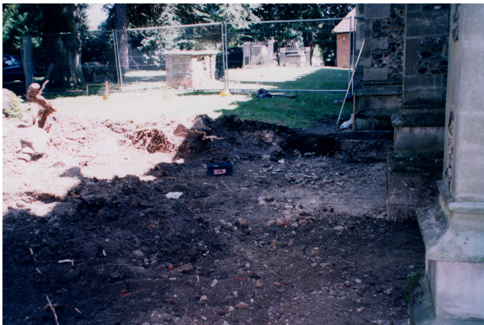
Plate 1 General shot of site during ground-reduction, looking east.
