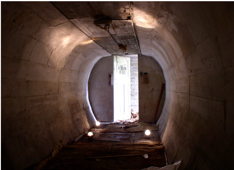
Plate 5 Air-raid shelter 1: internal view, looking north-north-east towards door.
