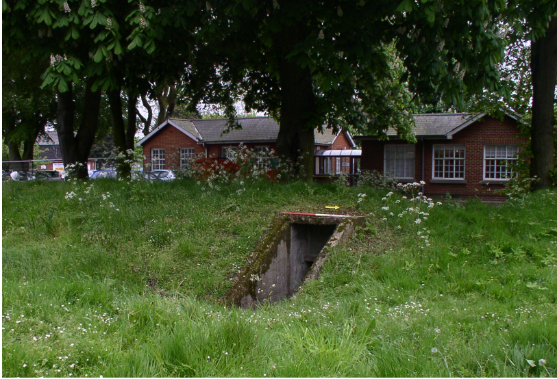
Plate 2 Air-raid shelter 1: north-eastern entrance, looking west, with former Army Radio offices in the background.
