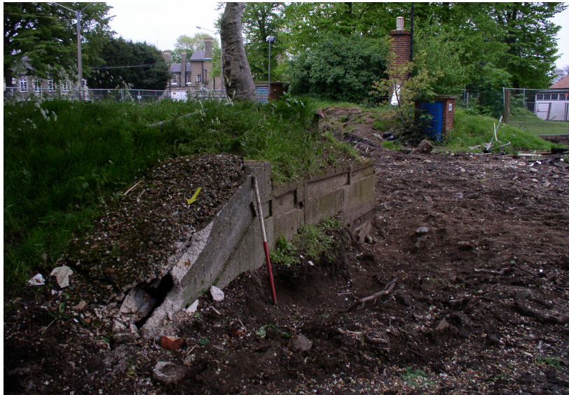
Plate 1 South-western corner of air-raid shelter 1, looking east, with air-raid shelter 2 in the background.
