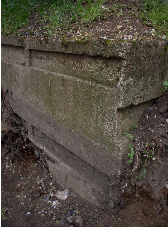
Plate 4 Air-raid shelter 1: shuttering detail at south-western end, looking north.
