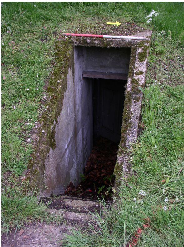
Plate 3 Air-raid shelter 1: north-eastern entrance, looking west.
