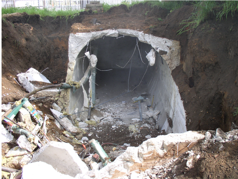
Plate 6 Air-raid shelter 2: south-western end during demolition, looking north-north-east.
