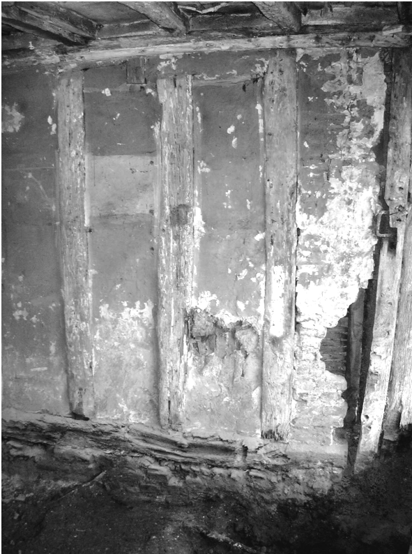
Plate 2 Southern wall of no 3: exposed timber frame, viewed from the north.
