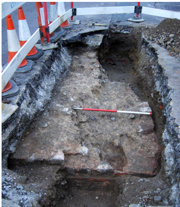
Plate 2 The central pier (F6) of the Roman south-west gate, viewed from the south.
