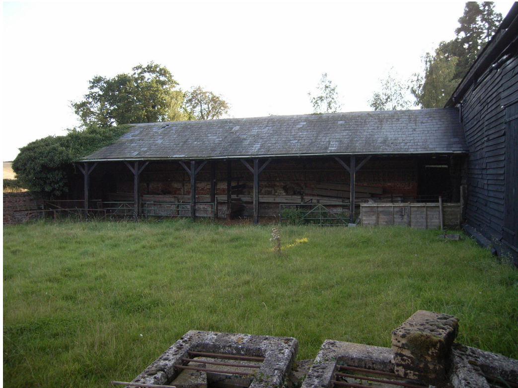
A1.17 Shelter 4: exterior from yard to east with old sack drying frames in foreground.
