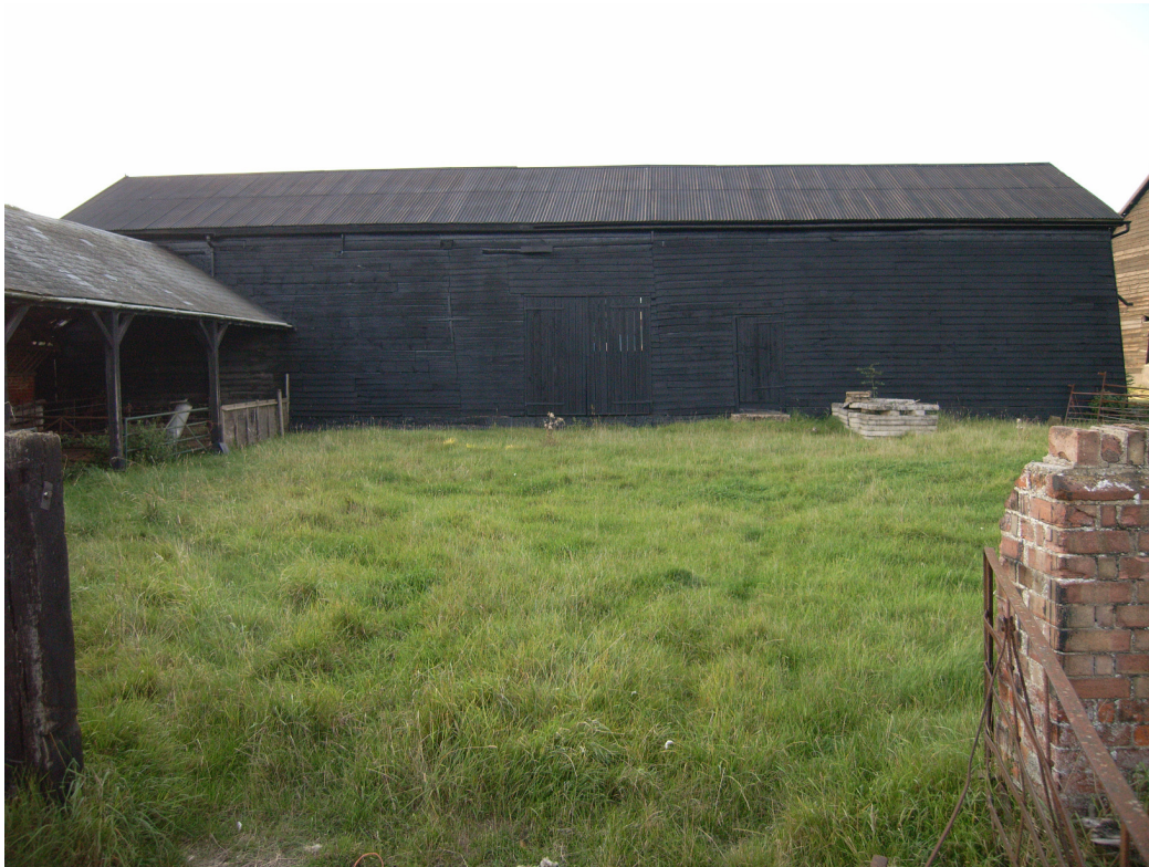
A1.1 Barn 1: exterior from south, showing elevation Q-V.
