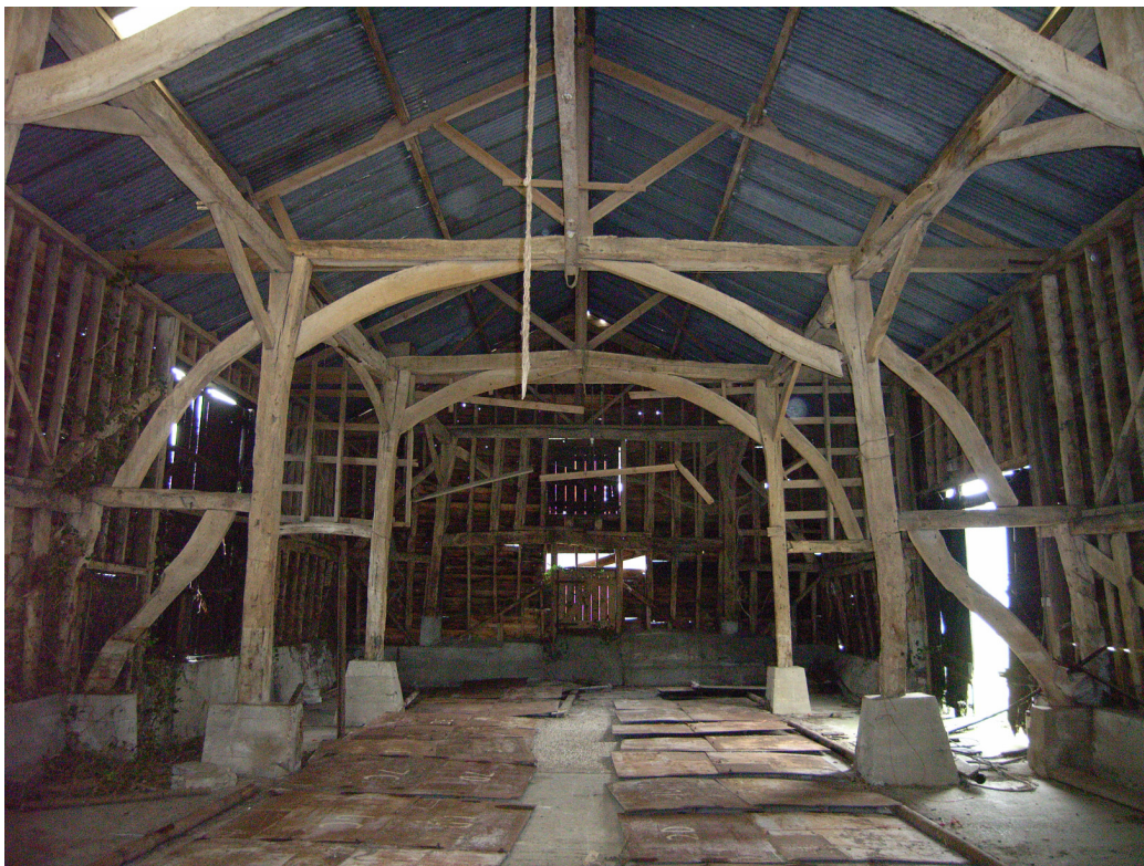
A1.8 Barn 2: general view of interior from east.
