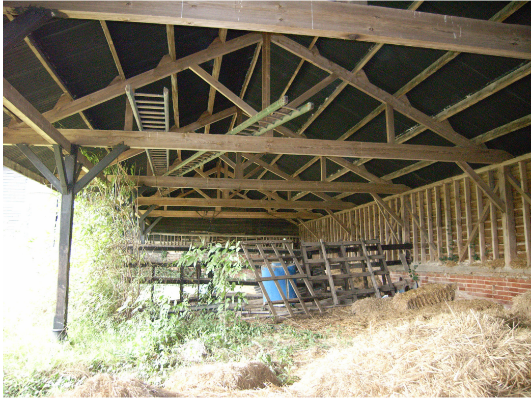
A1.15 Shelter 3: interior from south, looking towards hay-rack attached to barn 2.
