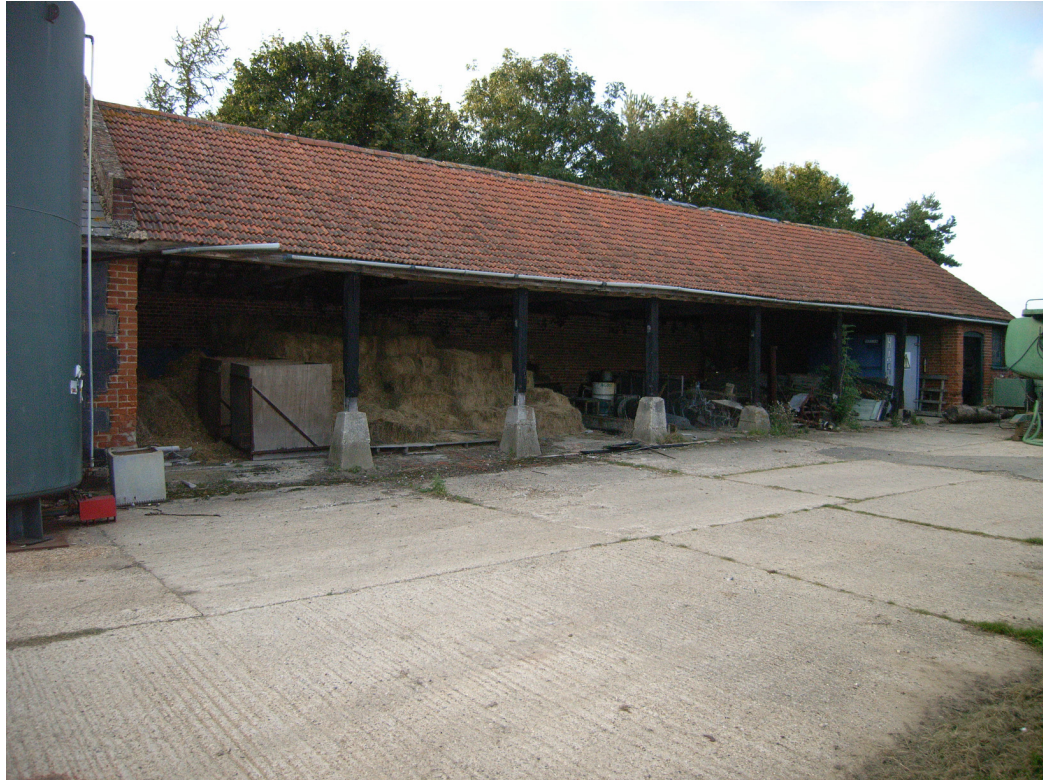
A1.21 Shelter 6: exterior from south, with later enclosed shed (7) to left.
