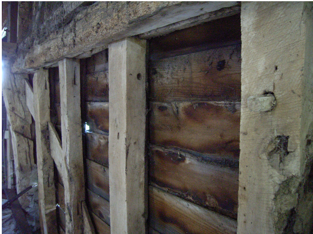
A1.12 Barn 2: detail of original studwork in bay C-D showing infill notches, external brace and passing brace trench in re-used post C to left.
