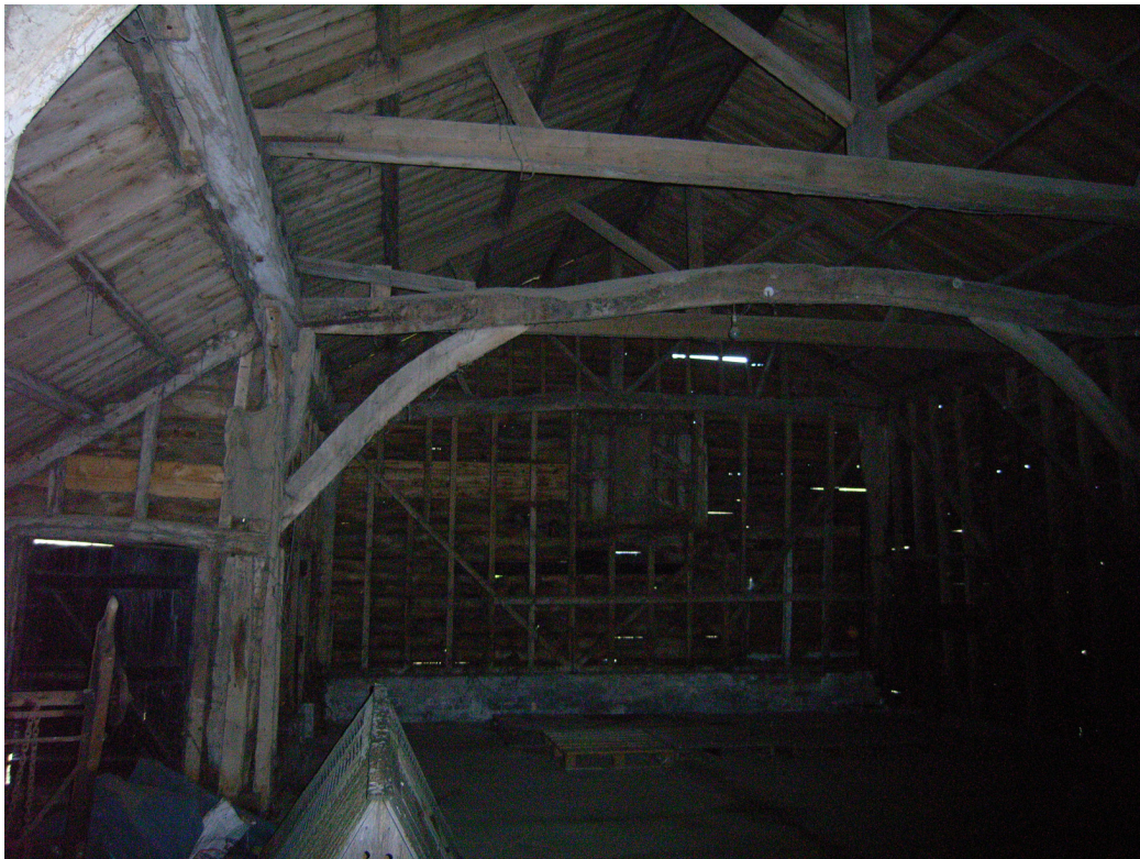
A1.4 Barn 1: general internal view from north-west, showing 1801 lean-to left.
