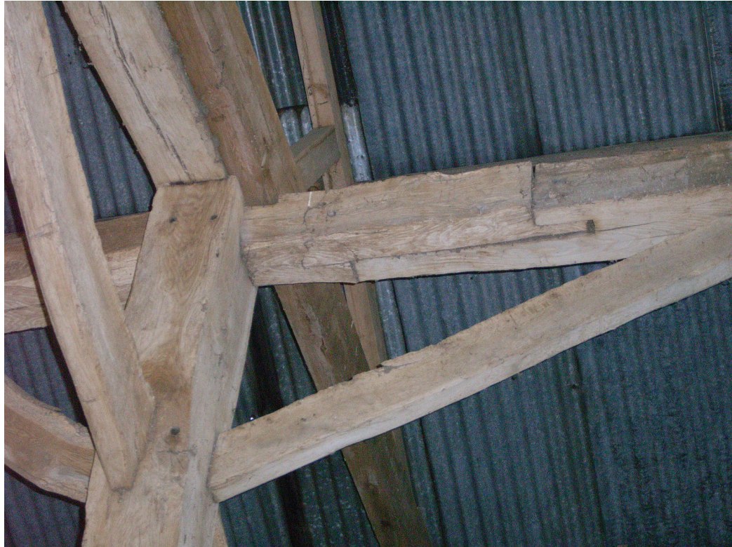
A1.11 Barn 2: detail of face-halved scarf with housed blades in bay I-H.
