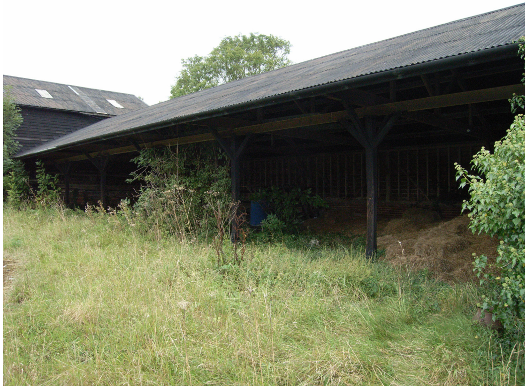
A1.14 Shelter 3: exterior from south-west with barn 2 to left.
