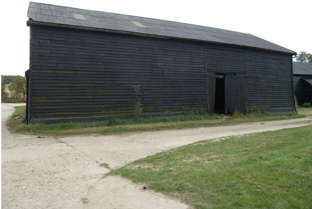
A1.7 Barn 2: exterior from north, showing elevation E-A.
