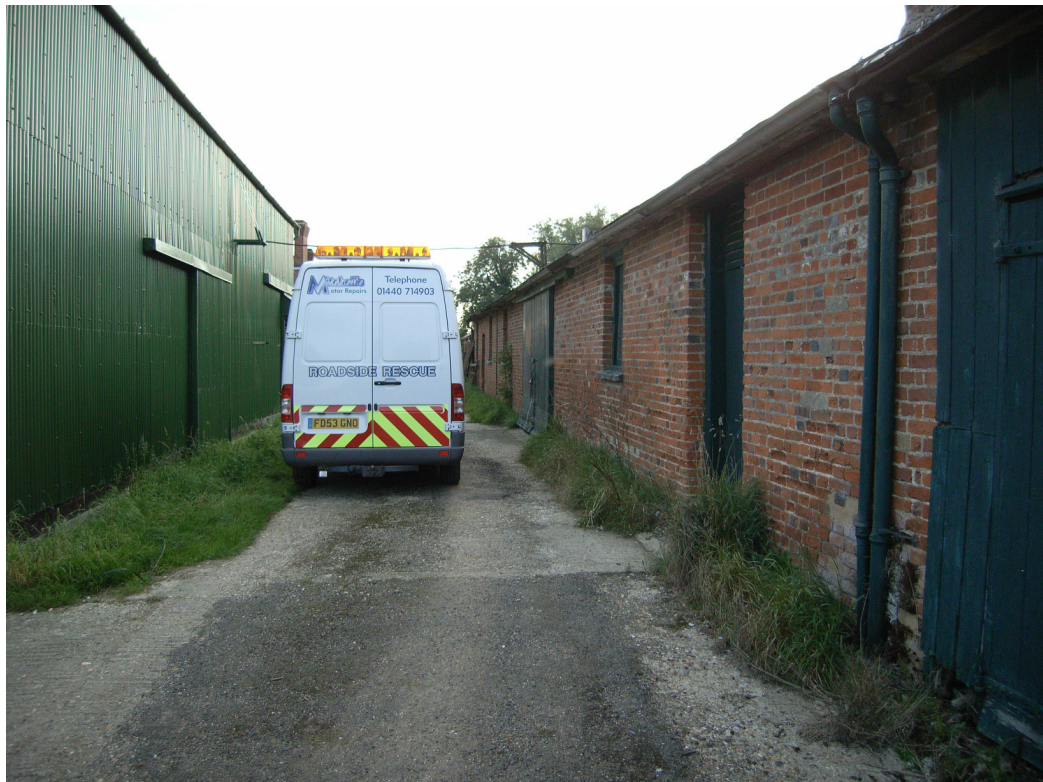
A1.22 Southern exteriors of sheds 9 and 8 from east, showing shed (7) to right.
