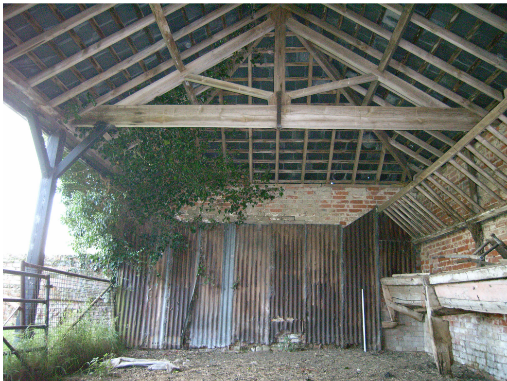
A1.18 Shelter 4: interior of southern gable showing king-post roof, manger and hay-rack.
