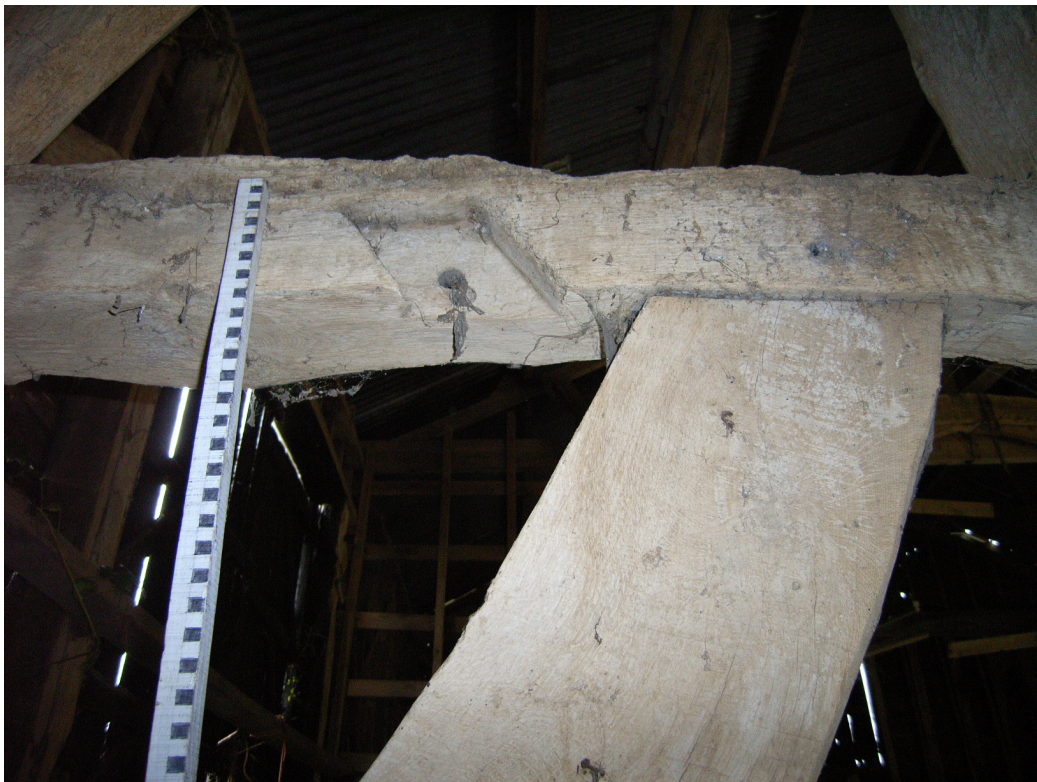
A1.10 Barn 2: detail of empty lap joint in re-used aisle tie to post I.
