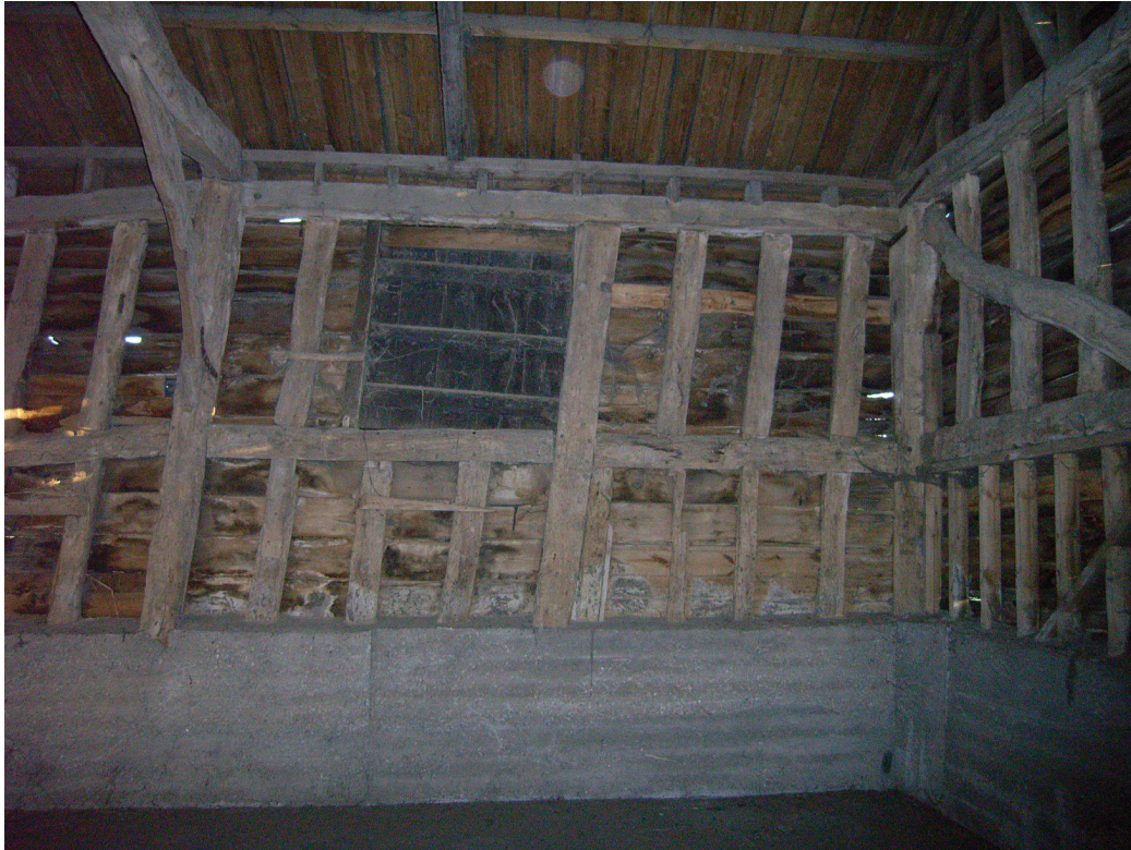
A1.5 Barn 1: internal bay R-Q showing largely original framing and later door above mid-rail (western gable to right).
