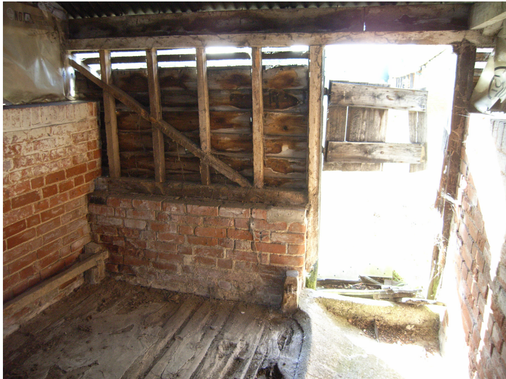
A1.20 Piggery 5: front internal wall of sty in eastern wing, with sow bed to left.
