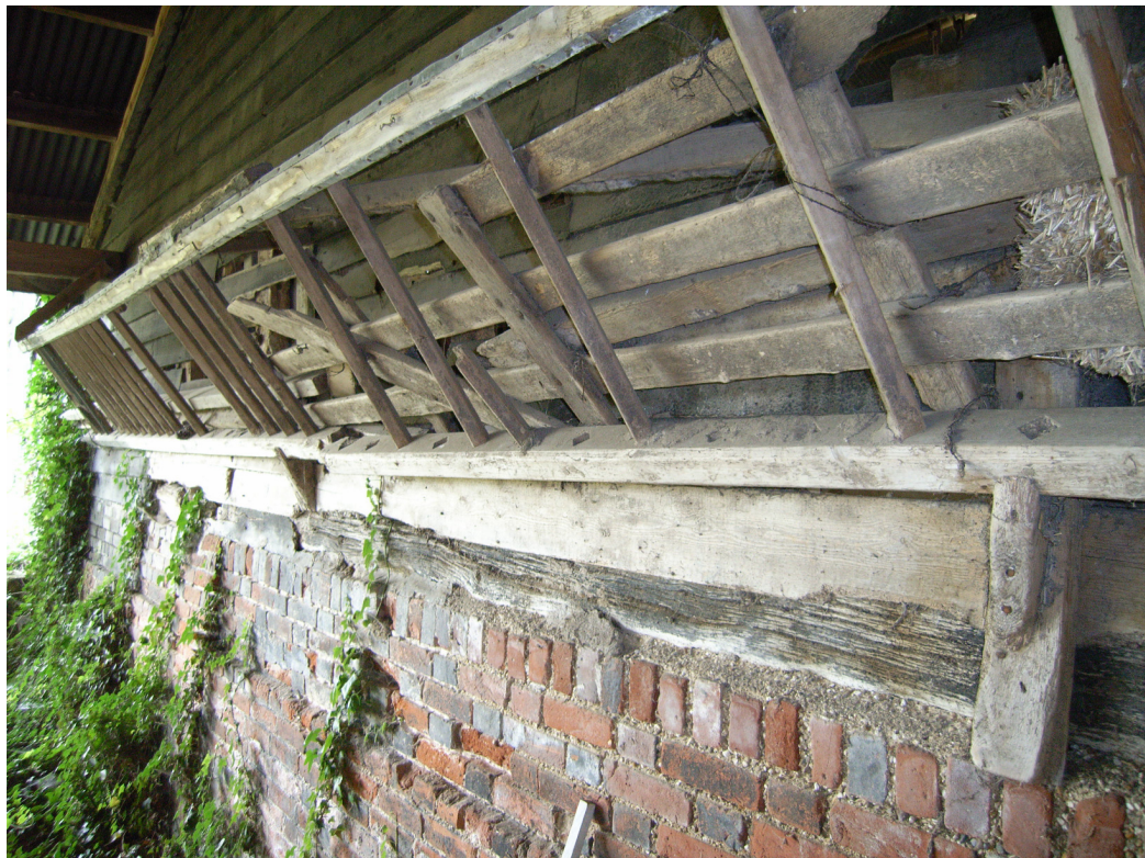
A1.16 Shelter 3: detail of hay-rack from south-east showing secondary rack within.
