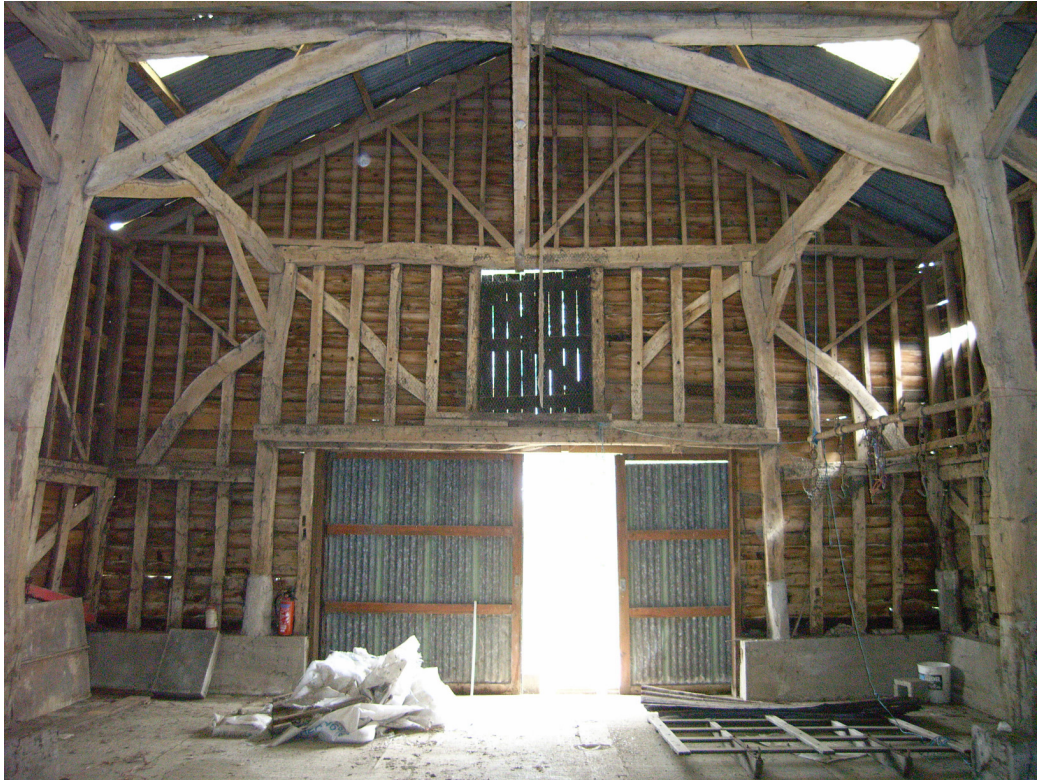
A1.9 Barn 2: interior of gable E-I showing late 20th-century sliding doors below mid-rail with early 20th-century door above.
