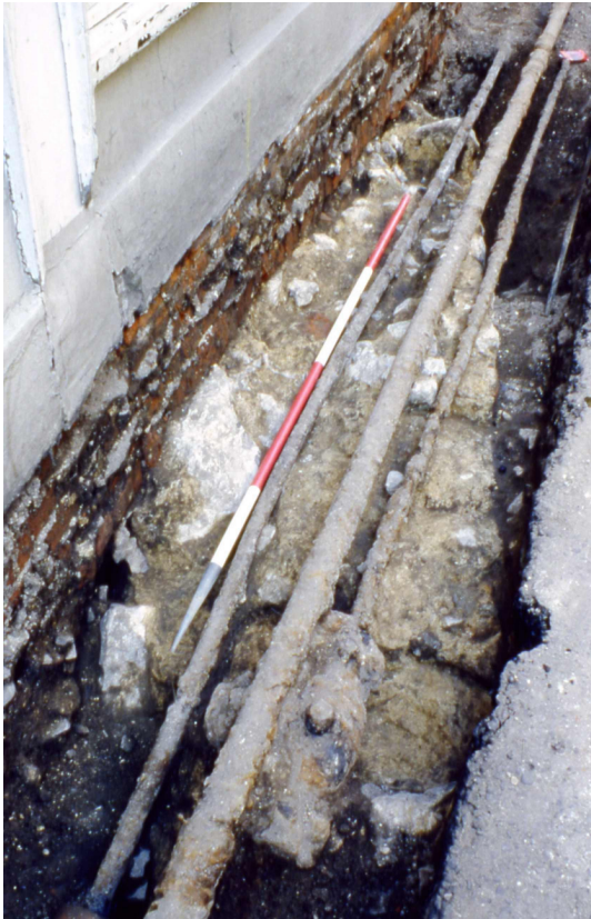
Plate 6 Foundation B, viewed from the south-west. It was crossed by modern services.
