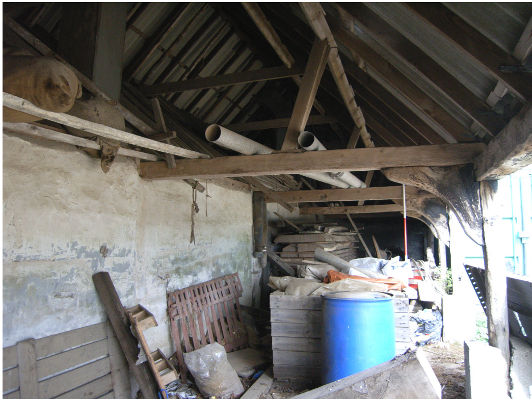
A2.10 Interior of cart lodge (8a) from south showing original bolted knee-braces to right and inserted milking parlour to left.
