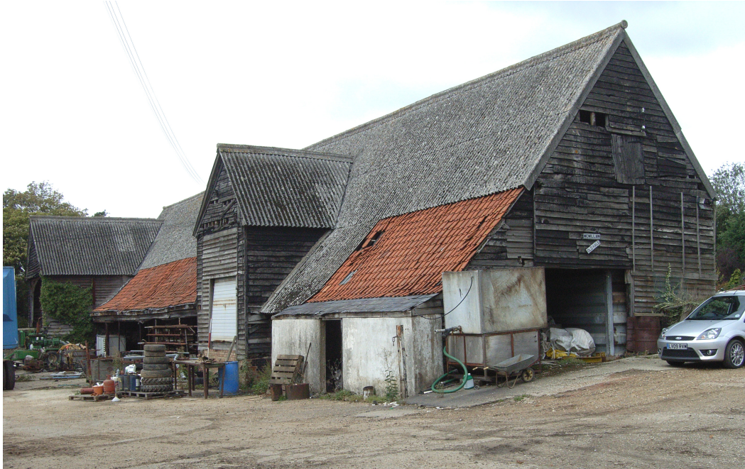
A2.3 Exterior of barn from south-east showing 17th-century western porch (2) to left and 19th-century eastern porch (4) to right with continuous lean-to sheds (2, 5 & 6) to southern yard elevation. The corrugated asbestos replaced thatch, but the pantiles and slate to the sheds survive from the 19th century.
