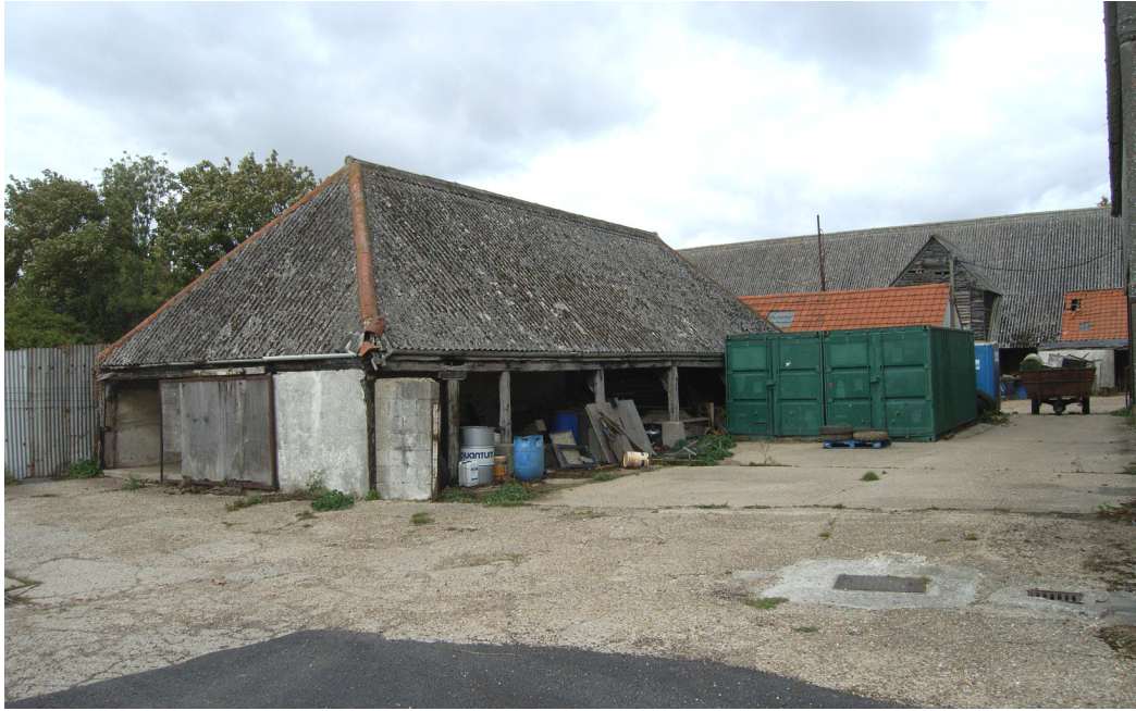
A2.9 Exterior of cart lodge (8) from south-east showing barn in rear to right.
