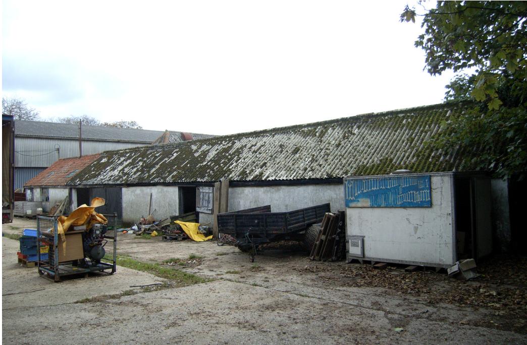
A2.7 Northern exterior of single-storied milking parlour (7) from north-west.
