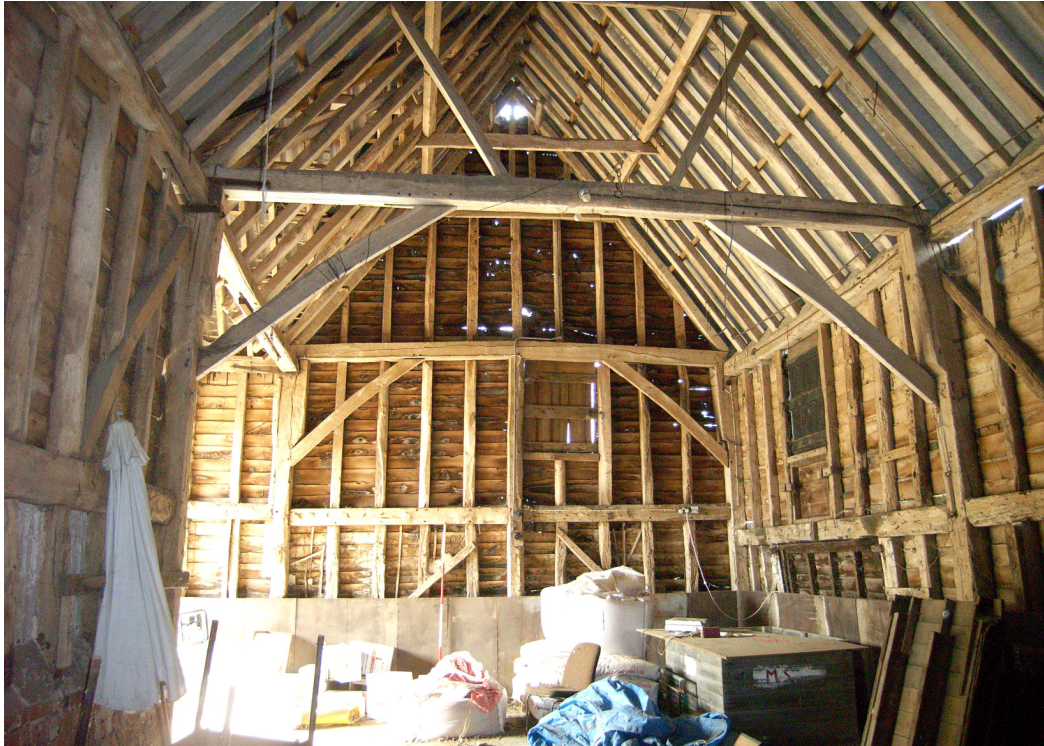
A2.5 Western interior of barn showing open frame of truncated gable and arch-braces flanking threshing bay (A).
