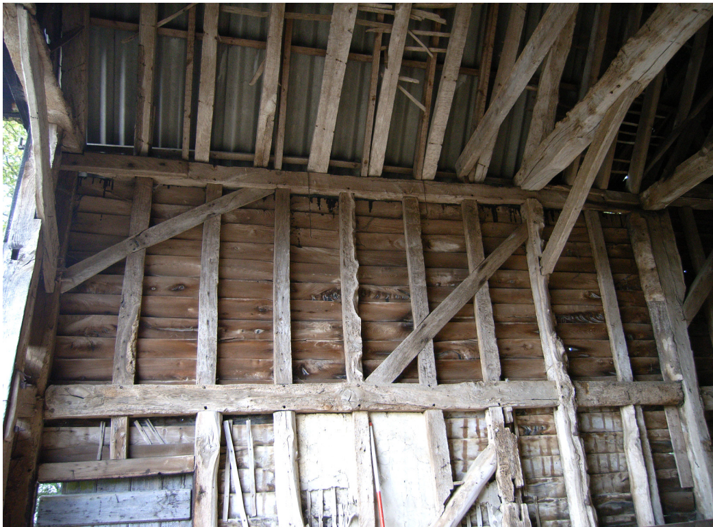
A2.4 Western internal elevation of 17th-century porch (2) showing trenched stud braces and arch-braced open frame to right (the studs below the mid-rail have been replaced).
