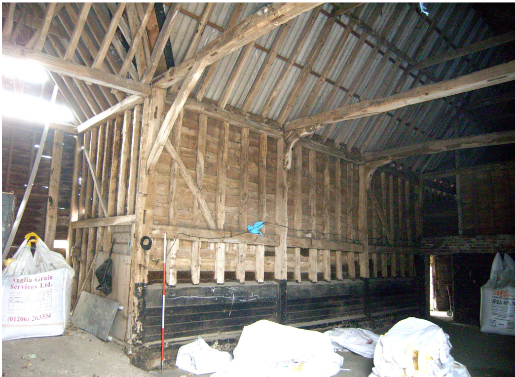
A2.6 Internal southern elevation of central bays G-F showing the eastern porch (4) to left and the brick granary in bay D to right. Note the re-used timber, primary stud braces and bolted knee-braces of the 19th-century walls.
