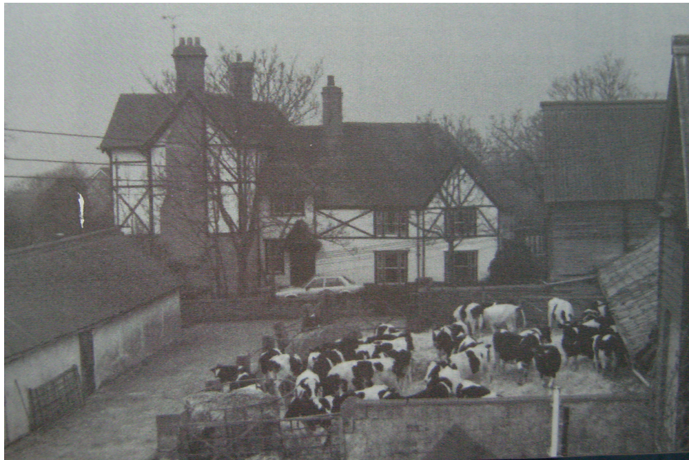
Fig 4 The farm yard from the east in circa 1975. Showing the farmhouse in centre (with its jettied late-medieval range to the right and later additions to left), the milking parlour (7) to the left and the barn to the right. Illustration from 'Boreham: History, Tales and Memories of an Essex Village', ed. Eleanor Burgess, n.d. (1980s).
