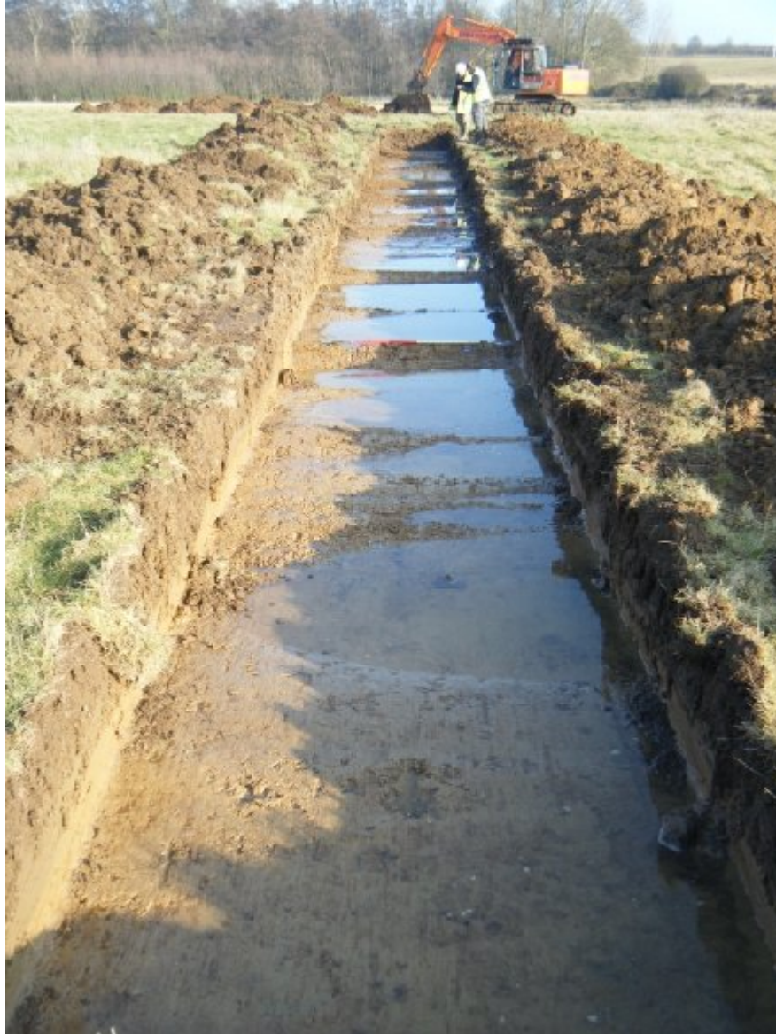
Plate 1: Trench 4, view east, showing typical ground conditions
