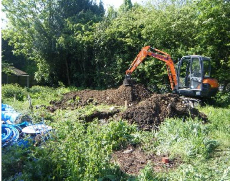
Plate 1: excavating T1, view N
