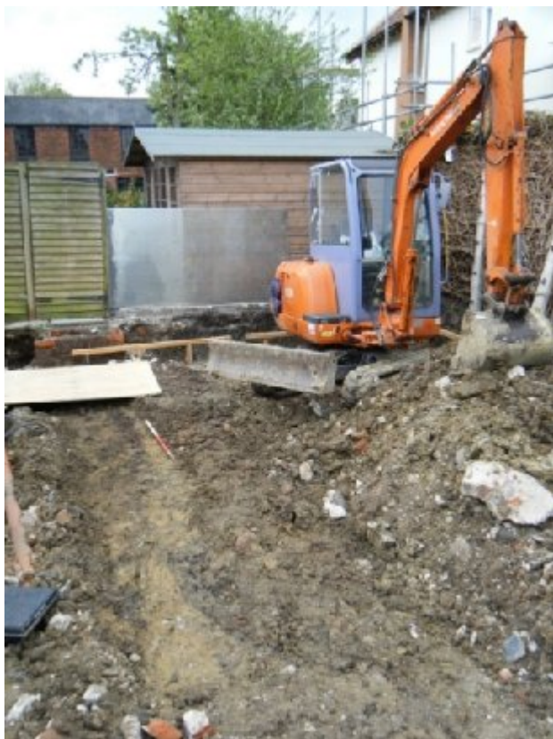
Plate 1: general view of site looking SW
