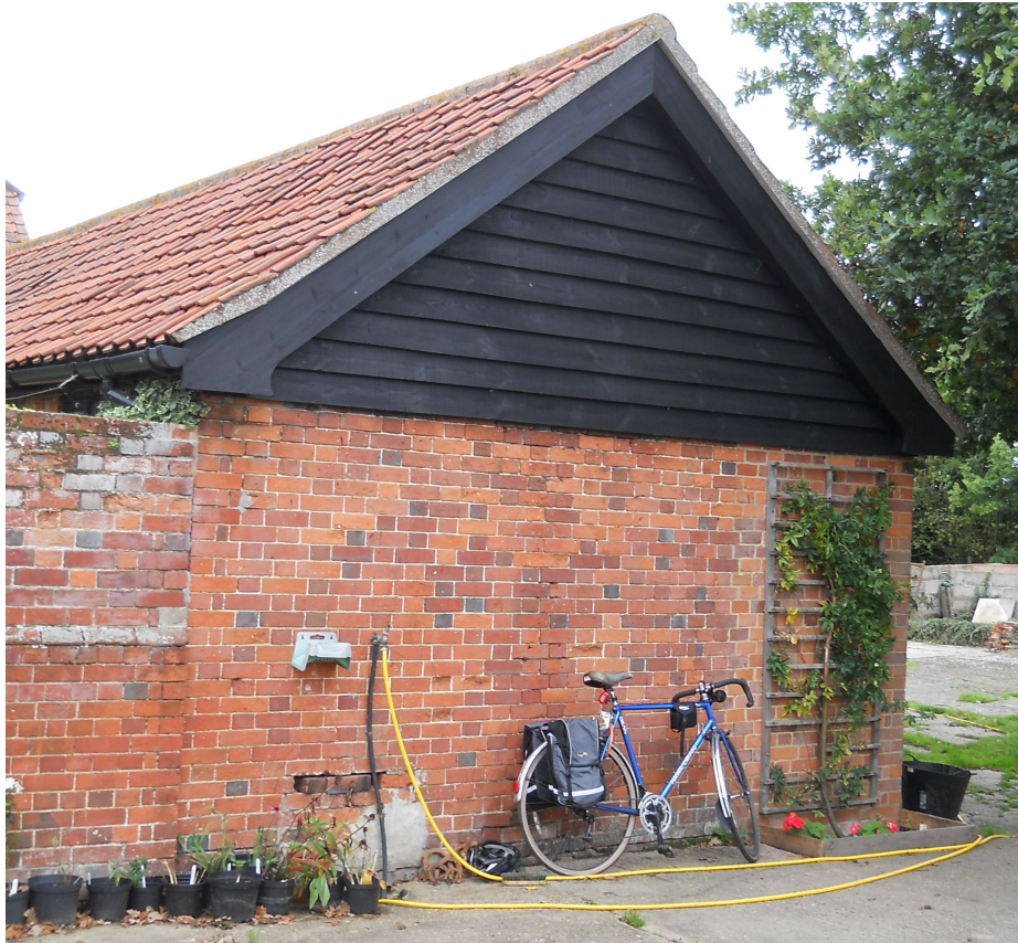
Plate 7 19th-century brick building (P) north-west of cart lodge/ granary (M), viewed from the east.
