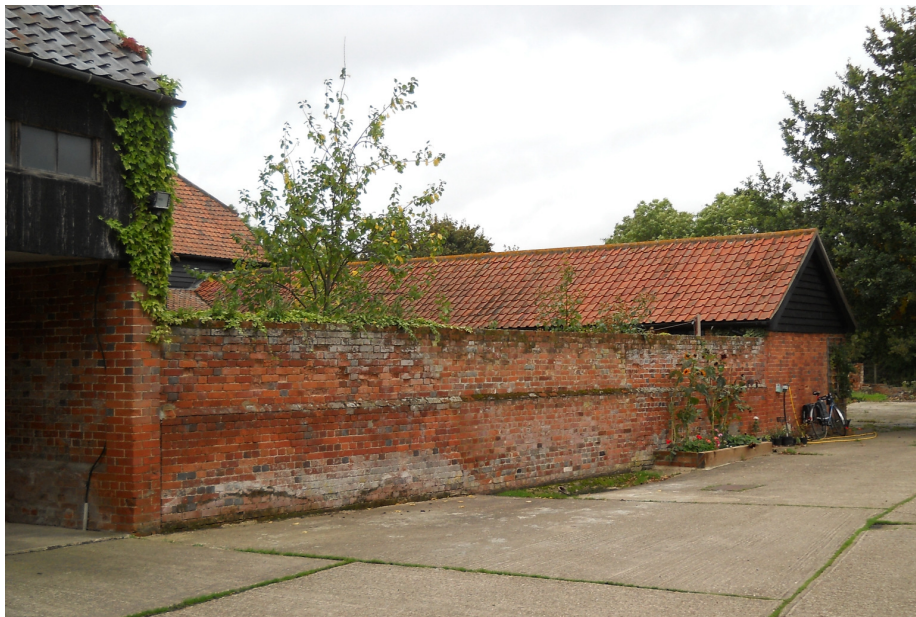
Plate 6 19th-century brick wall attached to northern corner of cart lodge/granary (M), viewed from the south-east.
