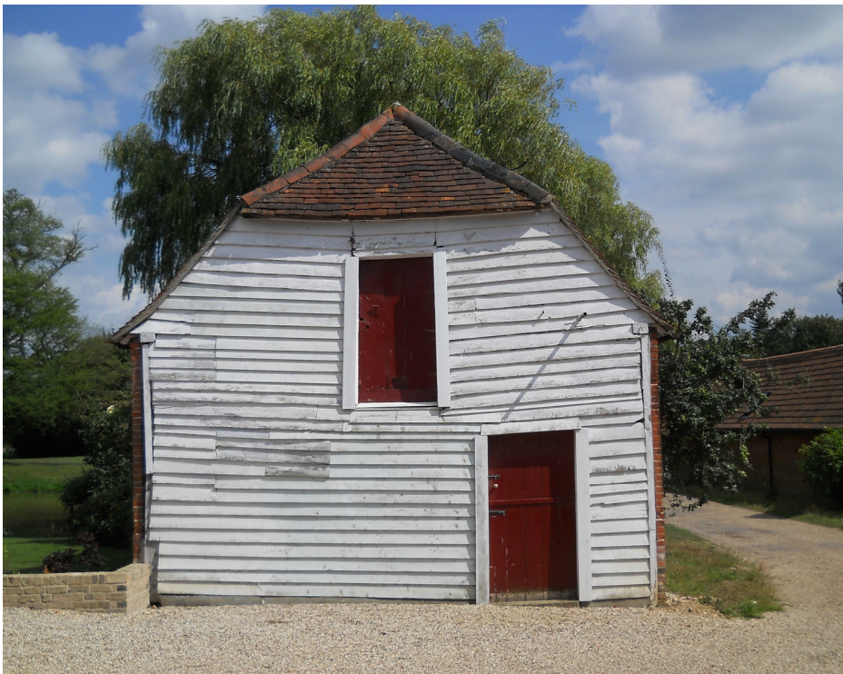
Plate A2 Granary (A): half-hipped roof, weatherboarding, doors, view from west.
