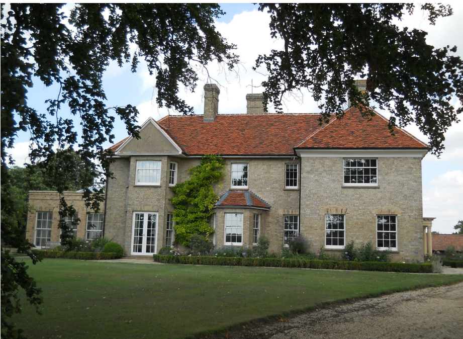
Plate A6 Clees Hall (B): view from south. (The building on the left is modern, built in last 10 years.)
