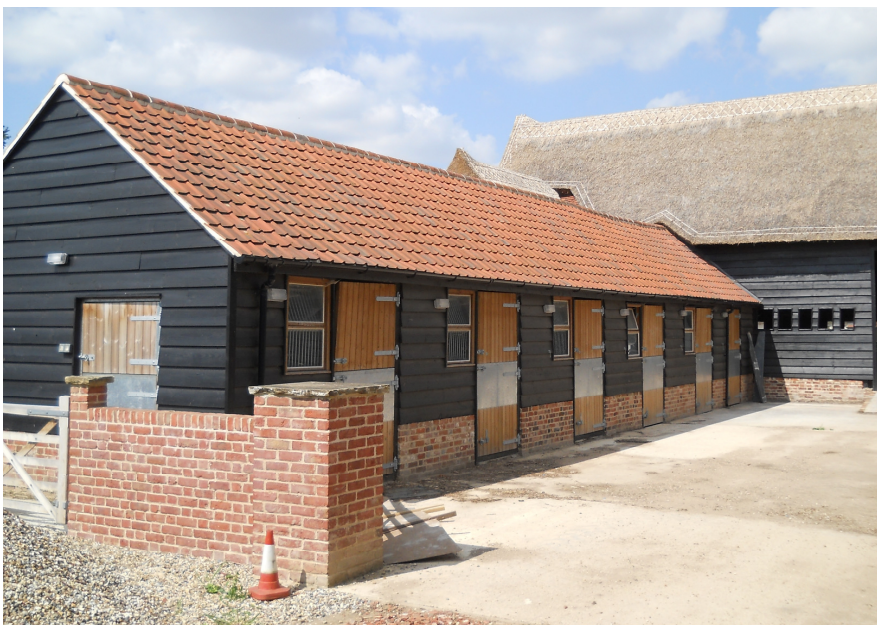
Plate A14 Modern stables (H) attached to medieval barn (E), view from south-east.
