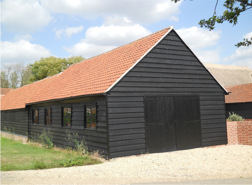
Plate A9 Former cart lodge (J), view from south-west.
