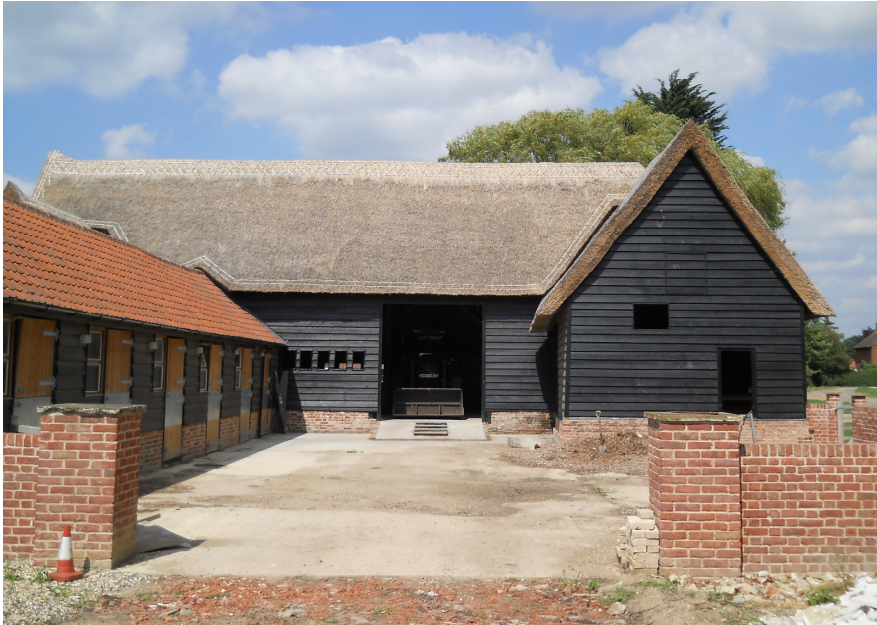
Plate A13 Medieval barn (E) and extension, showing modern stables (H) to left, view from south.
