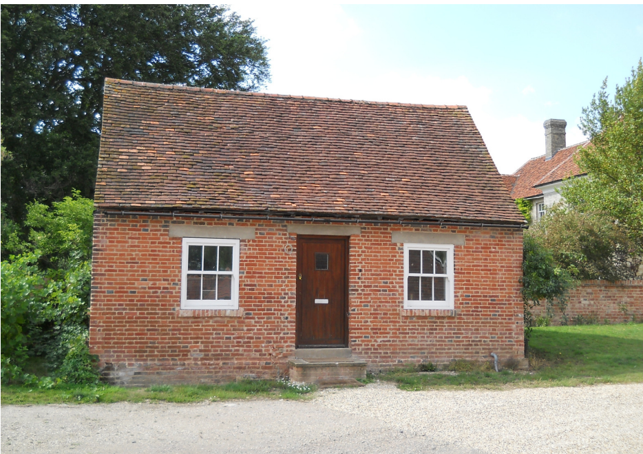
Plate A4 Farm office (D): brick building with clay-tile roof, view from east.
