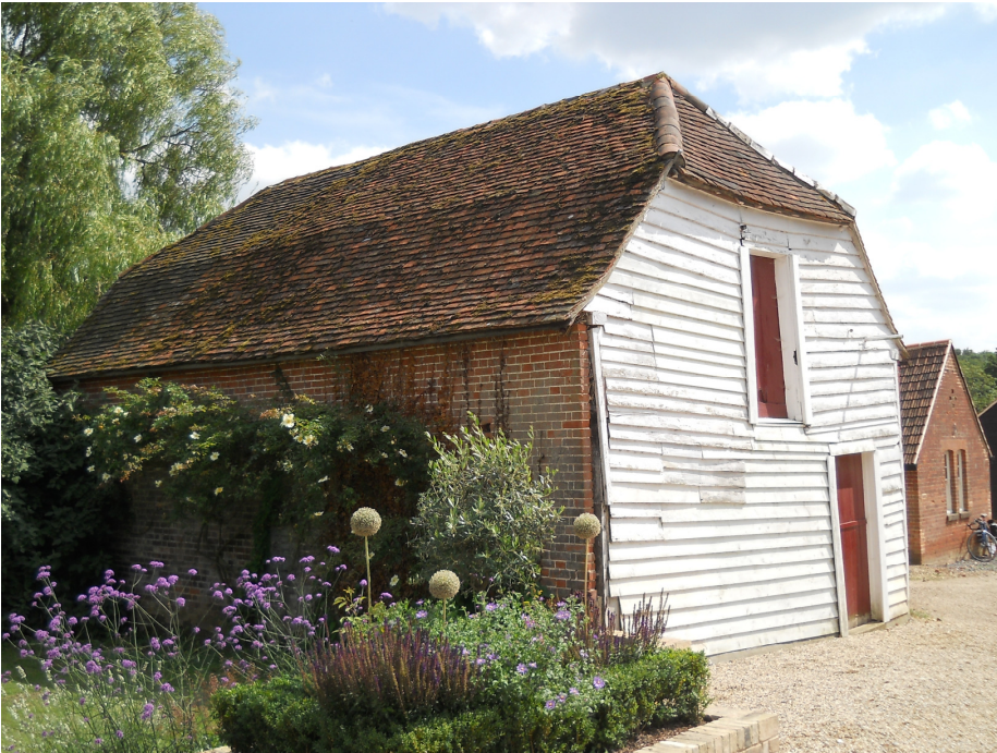
Plate A3 Granary (A): clay-tile roof, brick wall, iron reinforcing plates, view from north-west.
