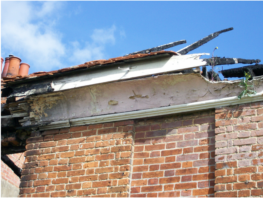
Plate 7: detail of the plaster cornice and eaves.
