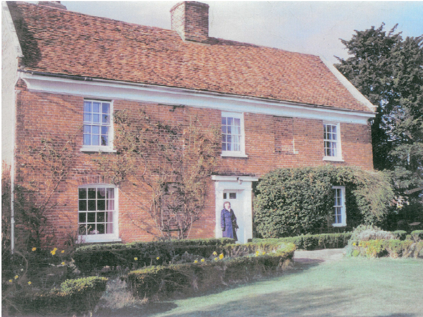
Plate 1: Tubbeswick Farm south elevation prior to the 2009 fire.
