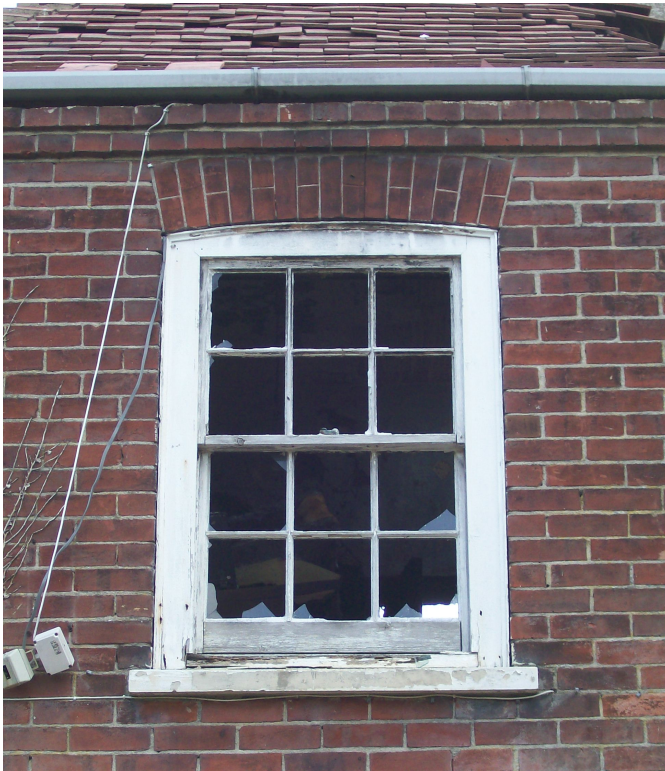
Plate 8: west elevation upper-storey sash window.
