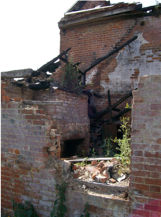
Plate 11: north elevation, showing pantry fireplace.
