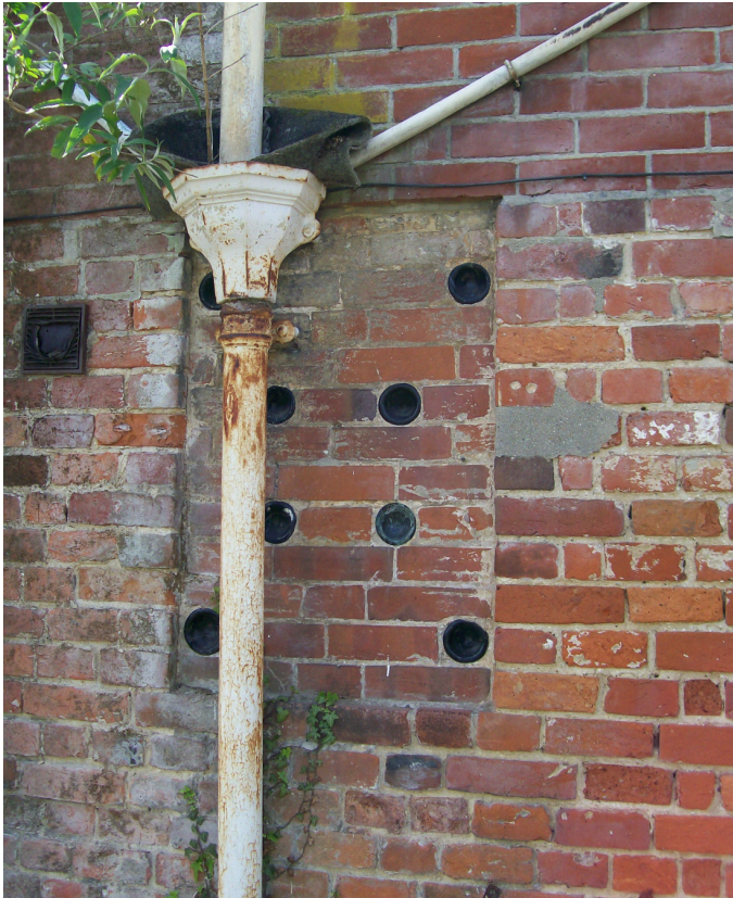
Plate 9: north elevation, detail of bricked-in window and bottle bases.
