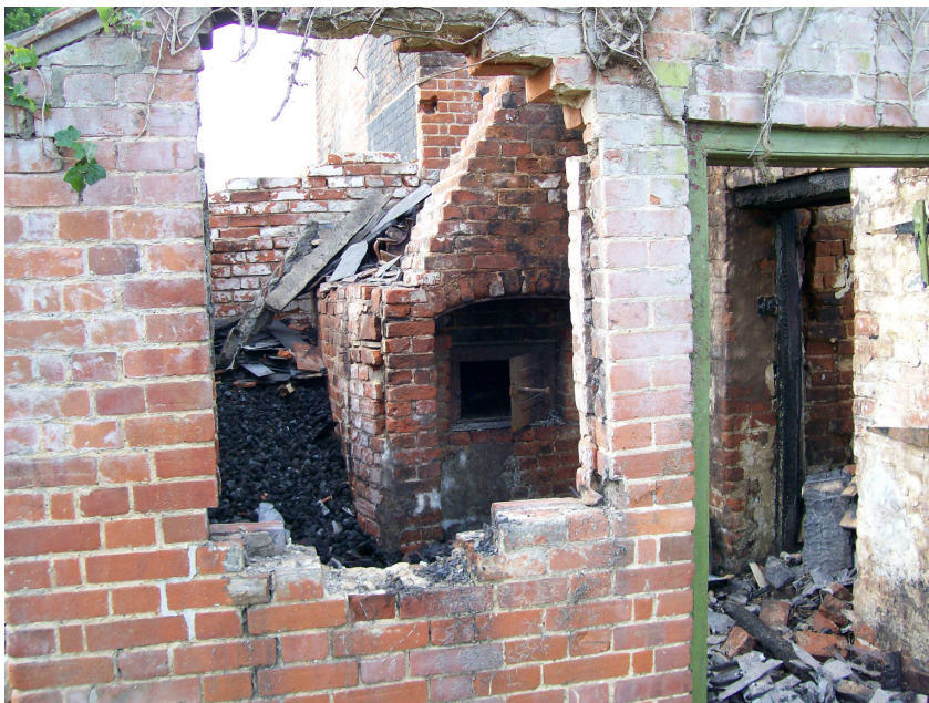
Plate 12: north elevation - boiler room, showing furnace.
