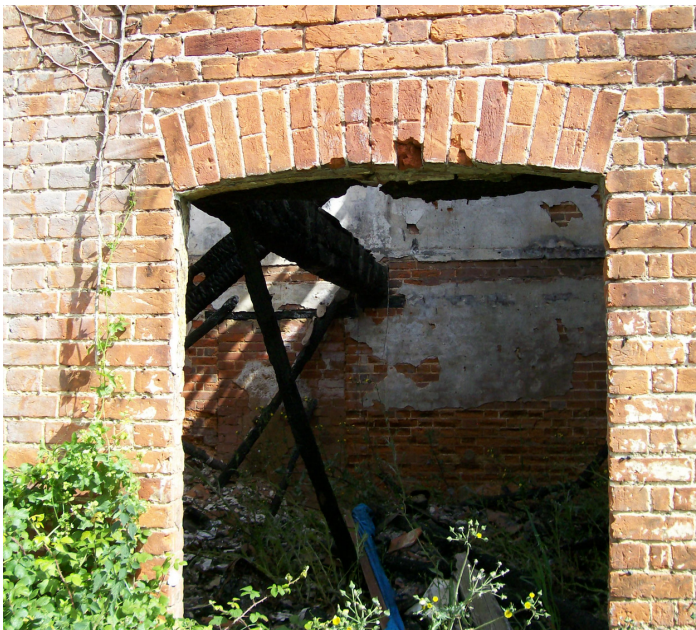
Plate 10: south elevation, east ground-floor room, showing oak bridging beam and blocked-in window.
