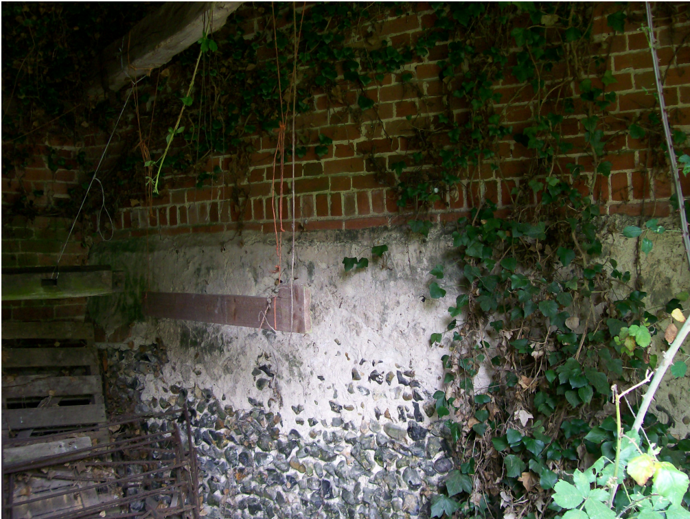
Plate 8 The flint wall separating Buildings 3 and 4 with later brickwork on top.
