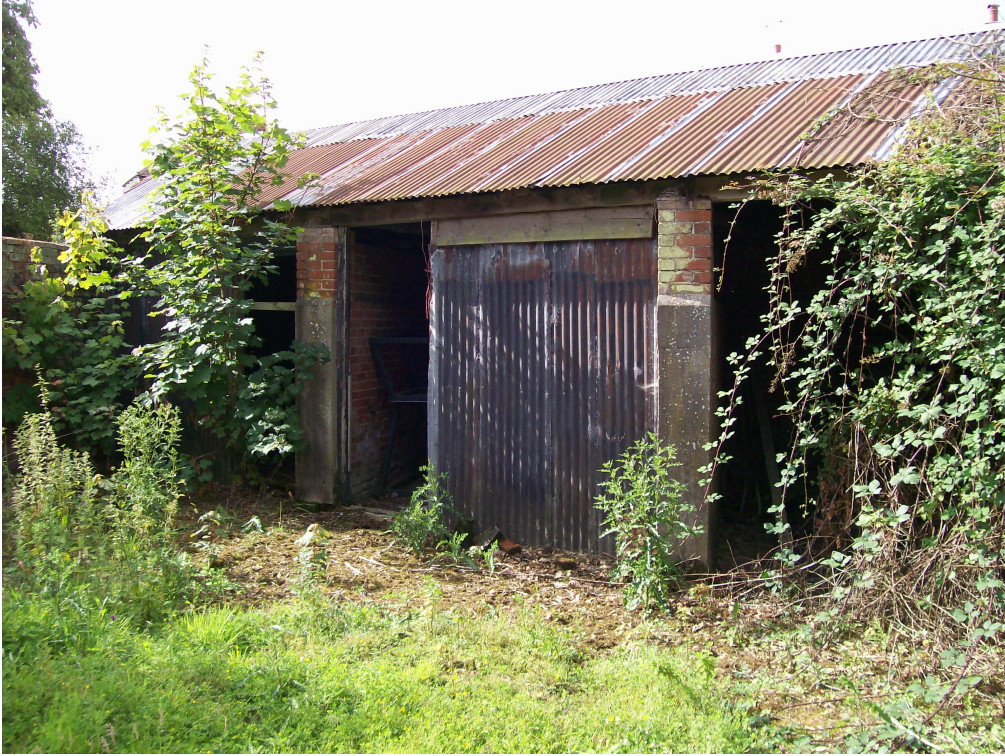
Plate 7 Building 3 showing the open-fronted bays.
