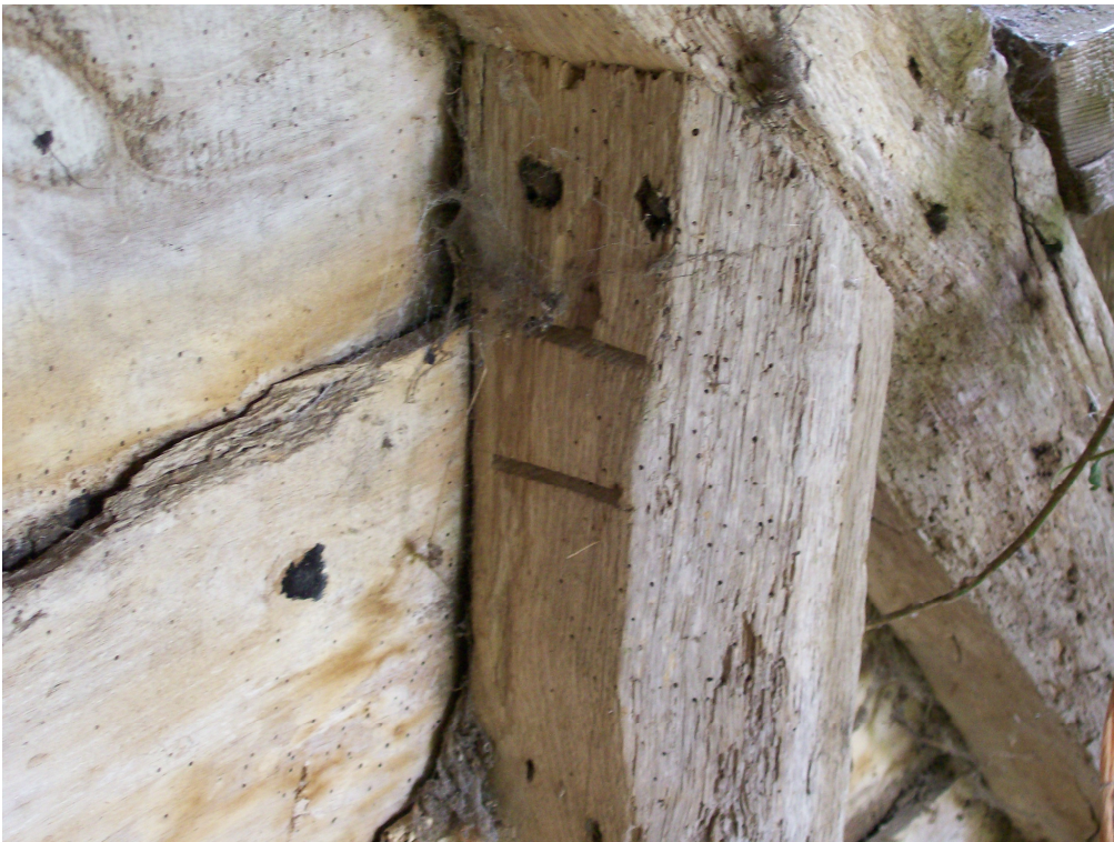
Plate 6 Carpenters' marks and nails holding the frame of Building 2 together.
