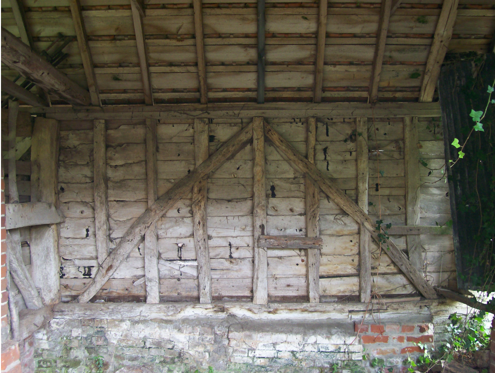
Plate 5 Building 2 original timber-framing of the north wall with scarf joint on sill beam.
