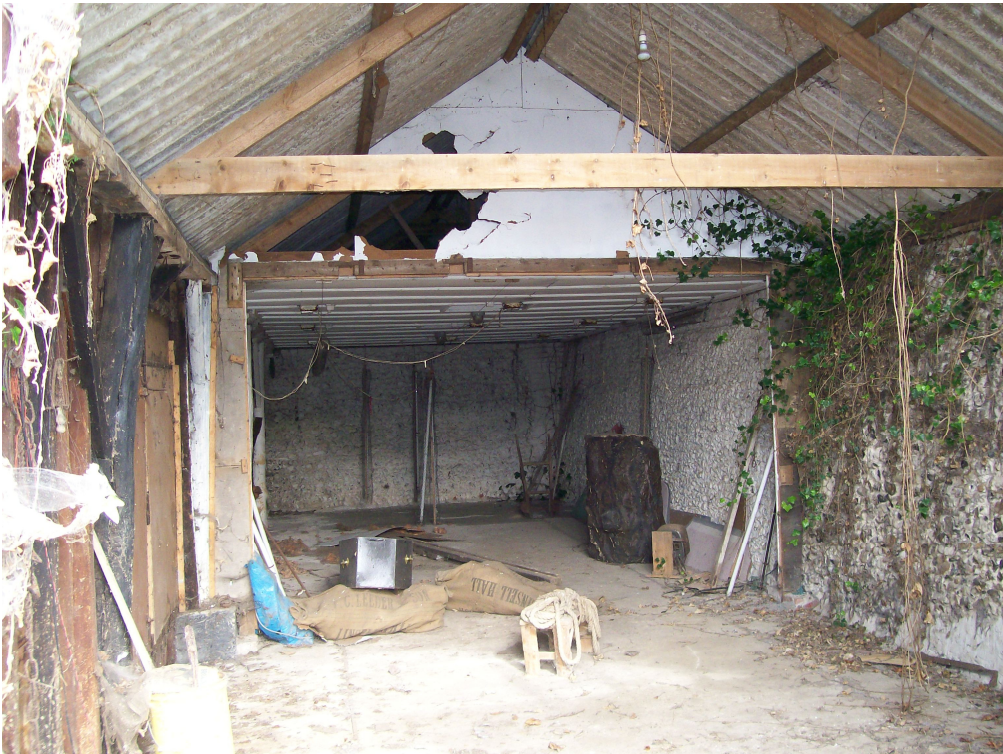
Plate 2 Interior of Building 1 showing flint walls and modern roof.
