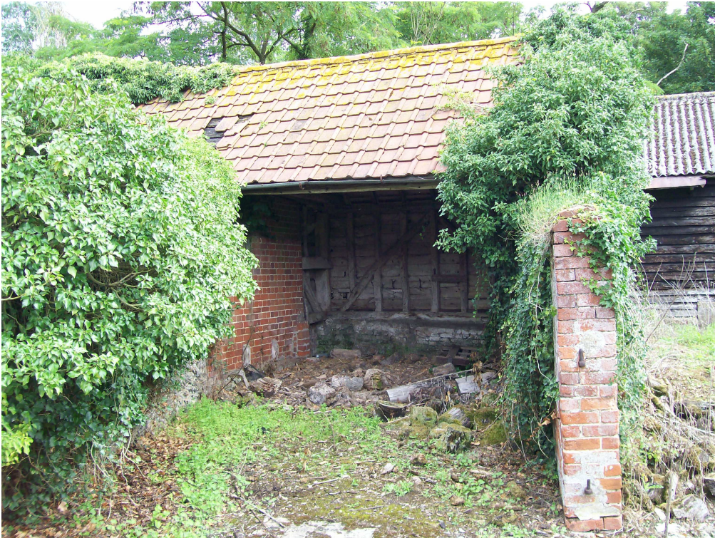
Plate 4 Building 2, bay 1 with the original timber-frame wall to the rear and the later brick cross-walls.
