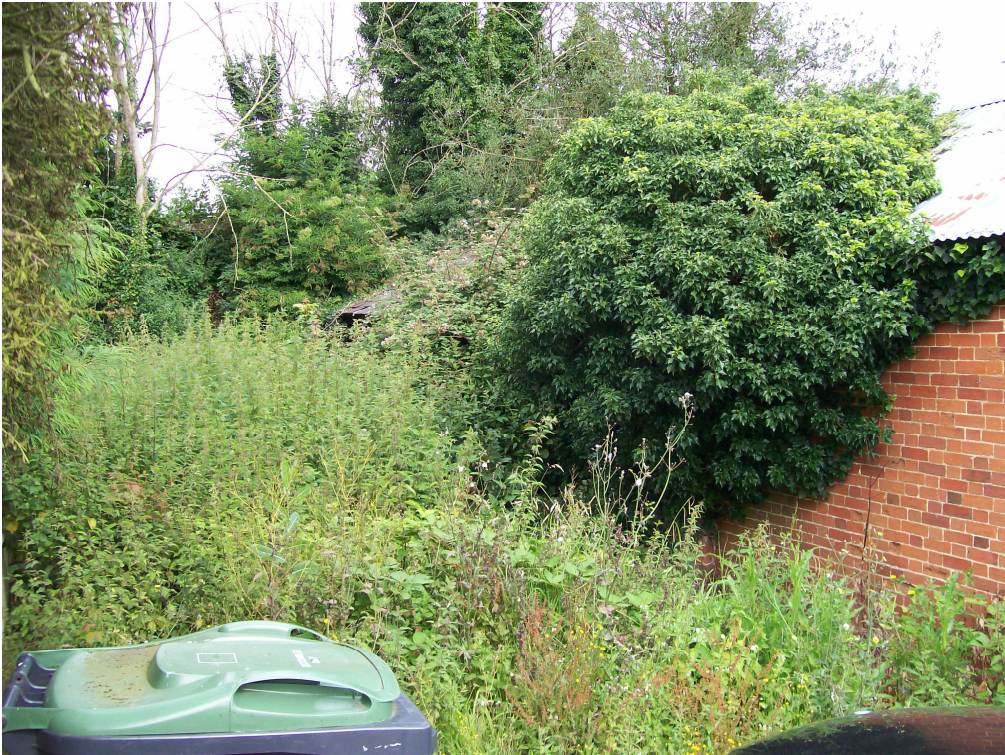
Plate 10 The south side of Building 4, showing the difficulty the vegetation presented.
