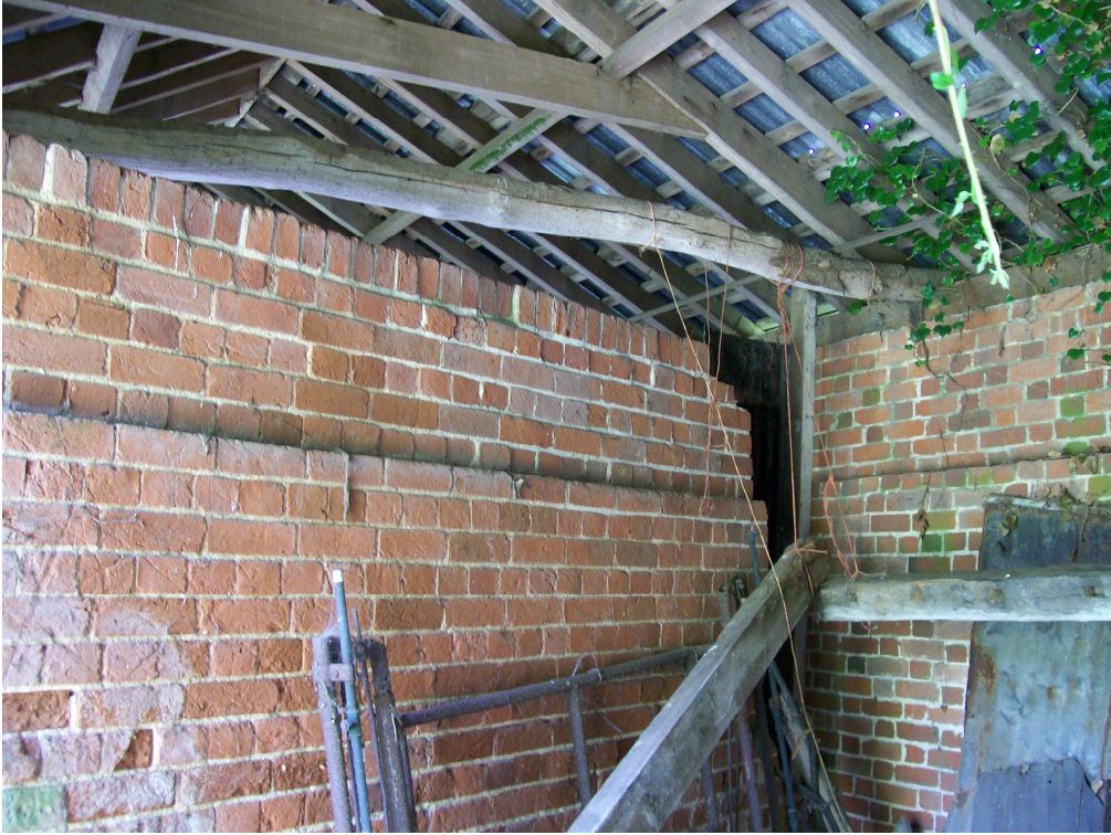
Plate 9 Interior of Building 3 showing the freestanding brick wall and re-used tie beam.
