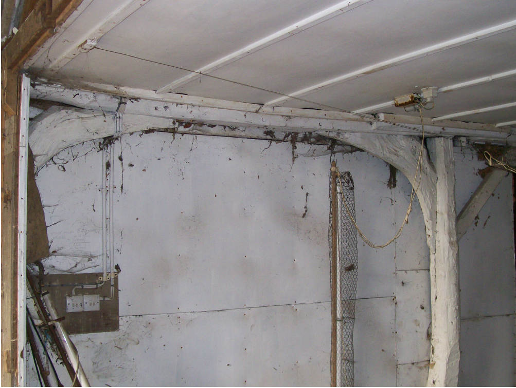
Plate 3 Building 1 re-used knee braces and scarf joint.
