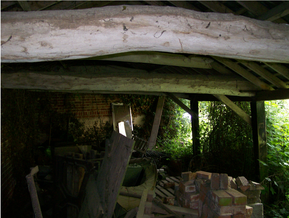
Plate 11 Interior of Building 4 showing the large re-used tie beams and the modern nailed straight bracing.
