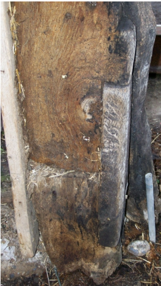
Plate 12 Barn 2, structure 2a; remains of threshold leap in surviving midstrey doorpost.
