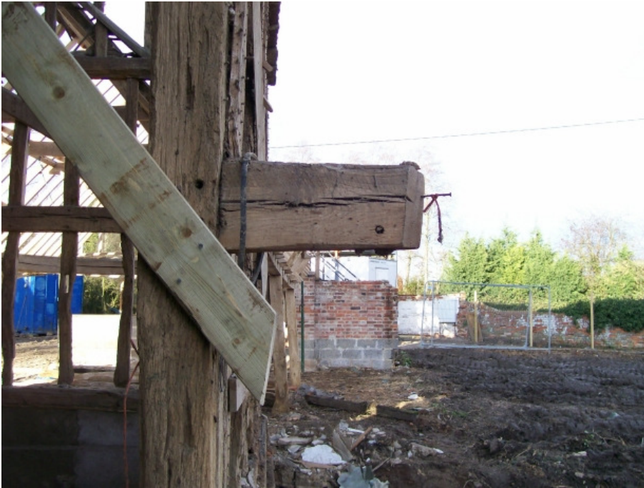
Plate 7 Barn 1, structure 1c; evidence for midstrey to the east of bay 2.
