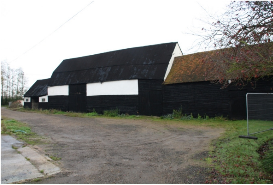
Plate 3 Barn 1, (left to right) structures 1b-d.
