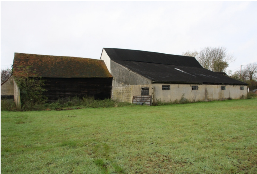
Plate 4 Barn 1 showing (from left to right) structure 1d with lean-to extension and remains of later shelter shed, and structure 1a projecting from the east side of structure 1c.
