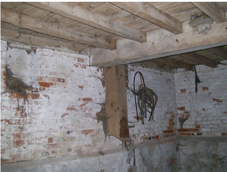
Plate 2 17th-century dovecote, lower storey interior showing blocked window and grain chute.
