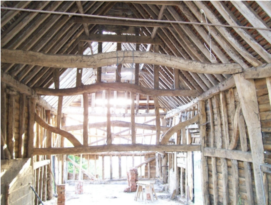
Plate 9 Barn 1, structure 1d; truss C with ogee braces.
