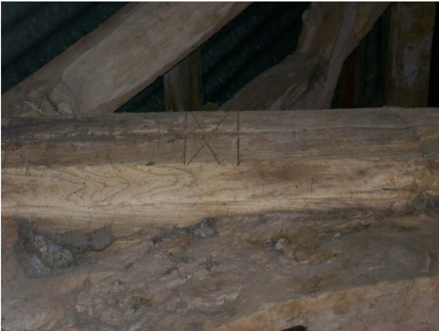
Plate 8 Barn 1, structure 1c; carpenters' marks on truss C above hanging knee brace.
