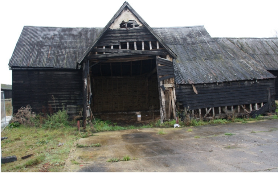
Plate 11 Barn 2, structure 2a; threshing barn with lean-to 2d to the right.
