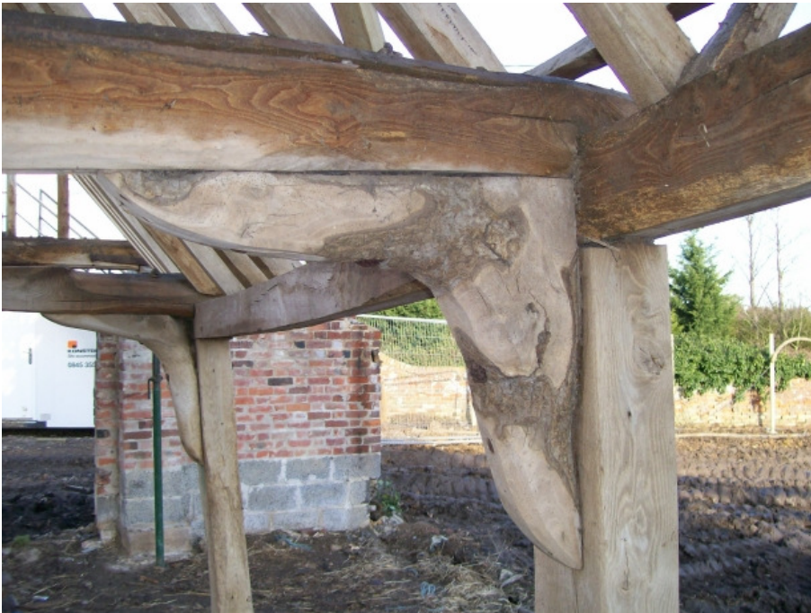
Plate 6 Barn 1, structure 1b; detail of hanging knee brace of truss B, with bark attached.
