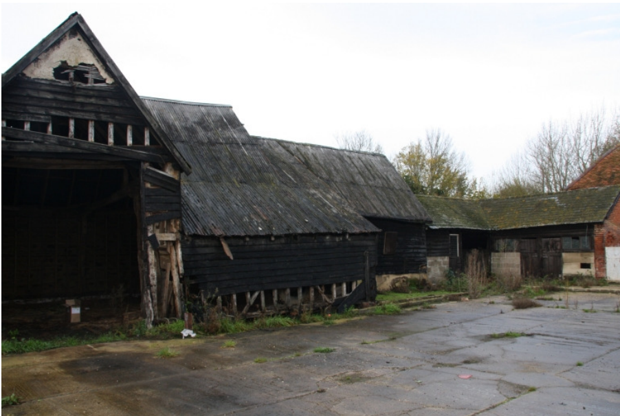
Plate 10 Barn 2, (left to right) structures 2a-c, with structure 2d in the foreground .
