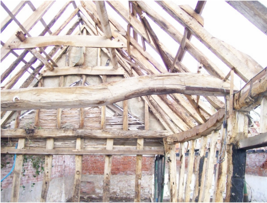
Plate 13 Barn 2, structure 2b; exposed timber frame showing curved and chamfered tie beam.
