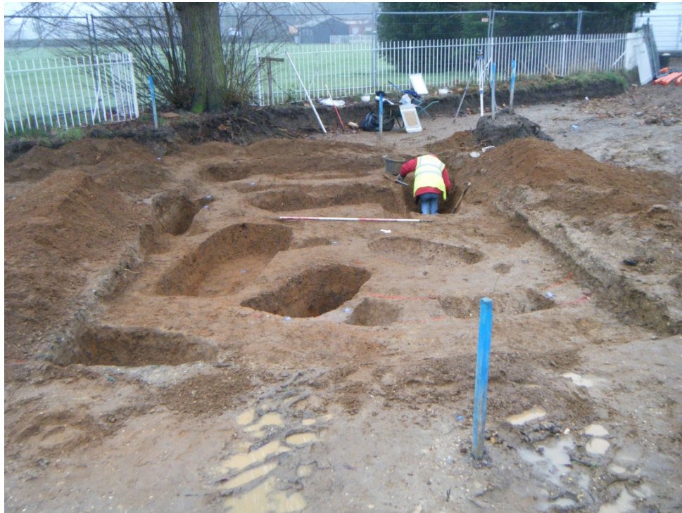
Plate 4 Excavation on the area of the attenuation tank (view south-west)
