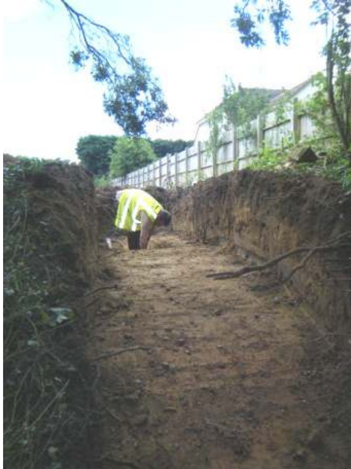
Plate 1: T1, excavating ditch F2 (view SW, up bank)
