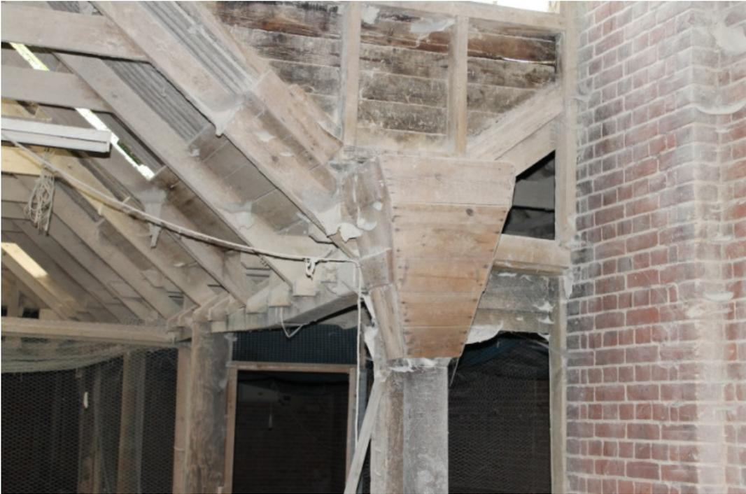
**Plate 9** Wooden rainwater trap for valley formed by shelter shed 4 and later covered yard of shelter shed 4
