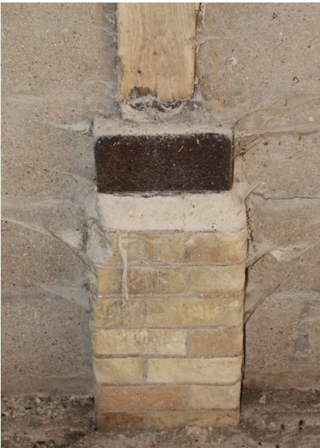
**Plate 14** Detail of brick and iron plinth for timber post of shelter shed 8
