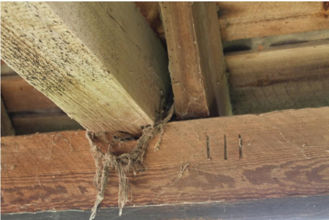
**Plate 12** Cart shed 7, carpenter's mark (III) on eaves plate
