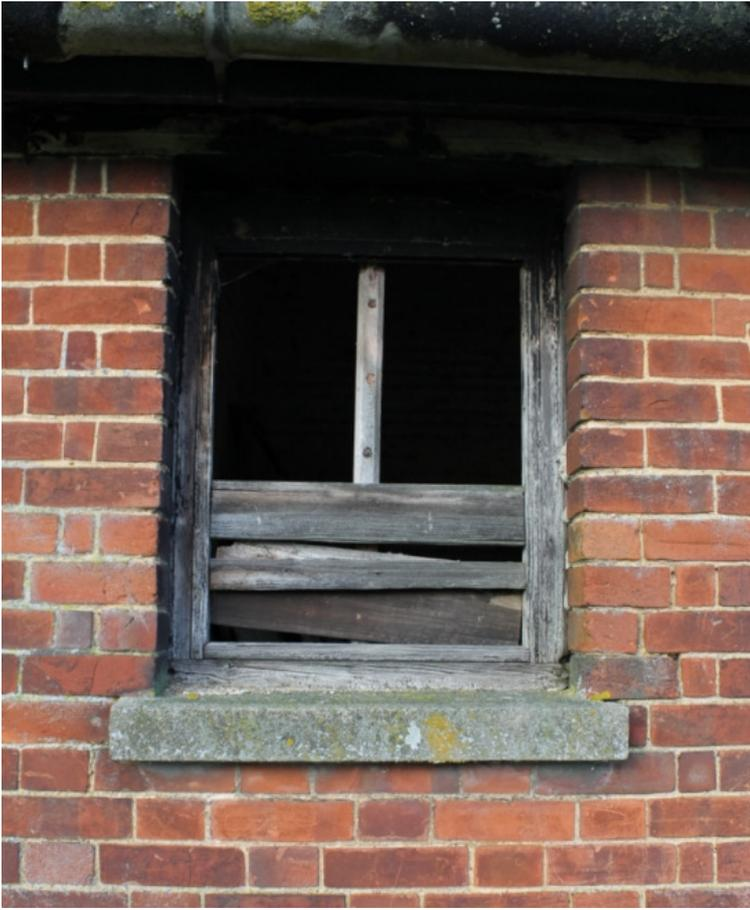
**Plate 7** Stable block 3, detail of window with chamfered mullion - view north-west
