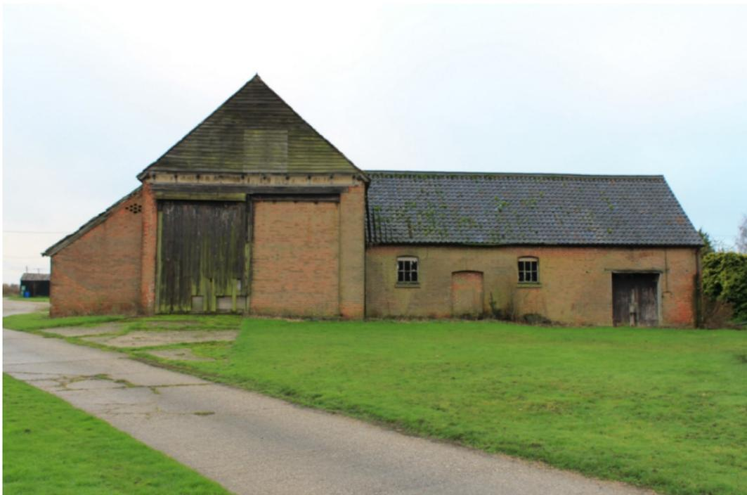
**Plate 4** Straw barn 2, note the sliding door and ornate cornice (with shed 1 to the right)
