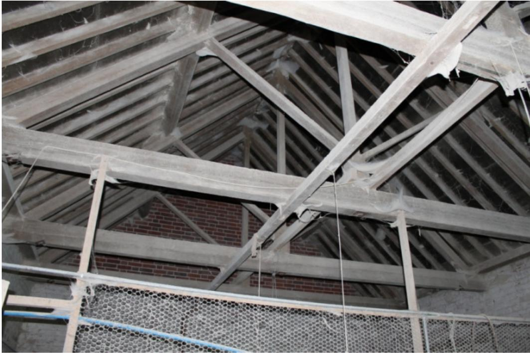
**Plate 3** Shed 1, detail of roof construction
