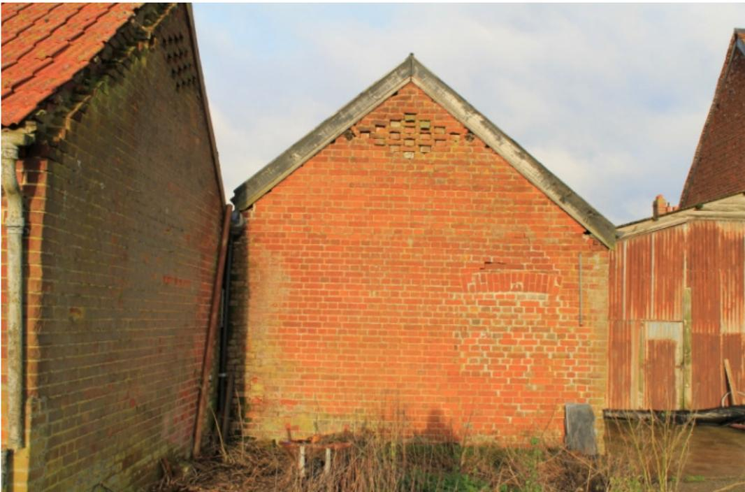
**Plate 10** South-east elevation of shed 6 showing diamond-pattern ventilation and blocked entrance - view north-west
