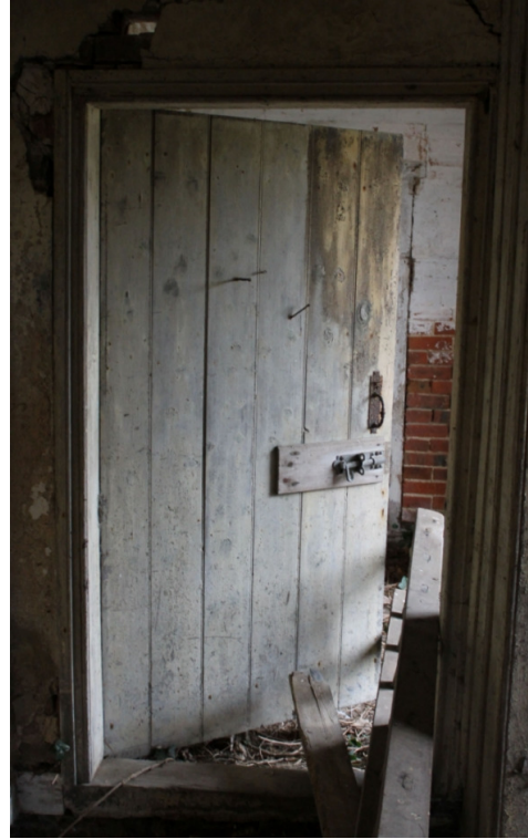
Plate 11 Original door to scullery - view south
