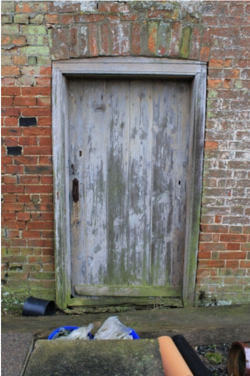
Plate 5 North elevation, original doorway - view south
