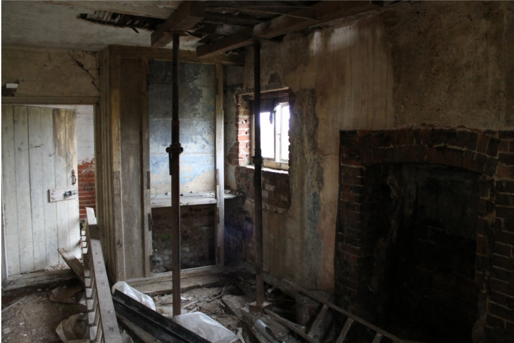
Plate 8 Kitchen, with scullery through door - view south
