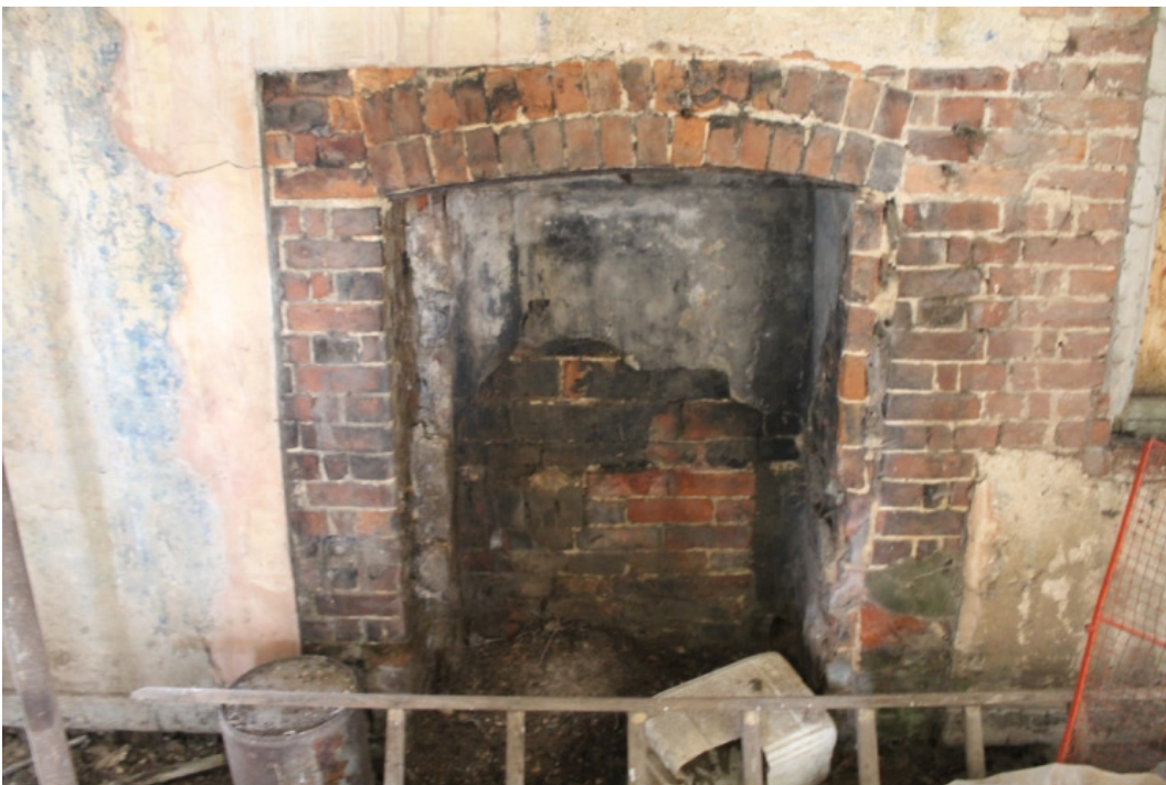
Plate 9 Kitchen fireplace – view west
