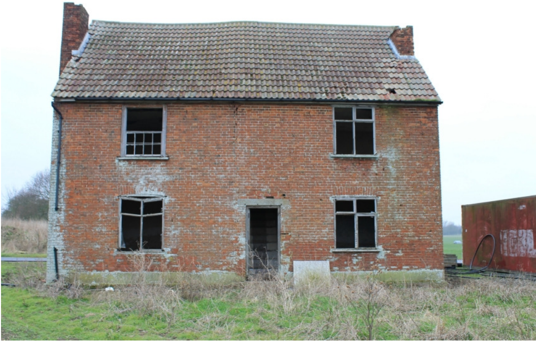
Plate 3 East elevation – view west
