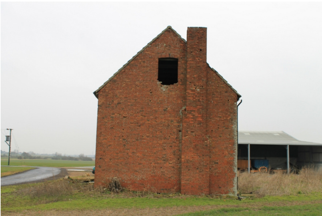
Plate 7 South elevation - view north
