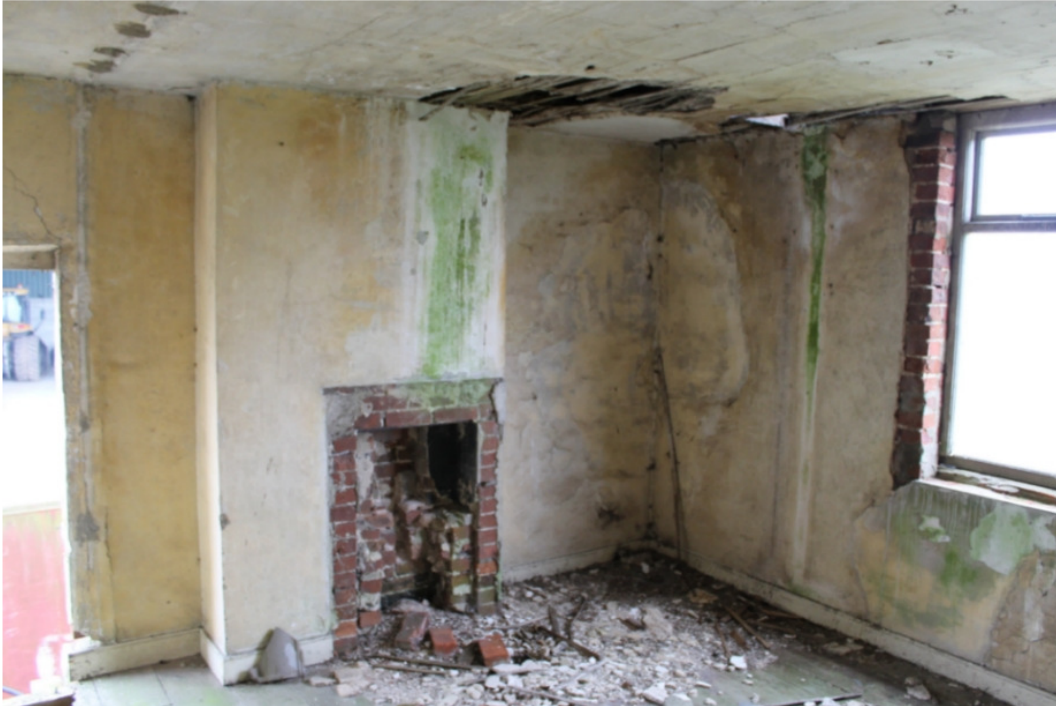
Plate 20 Bedroom 1 with remains of fireplace and inserted doorway to outbuilding – view north-east
