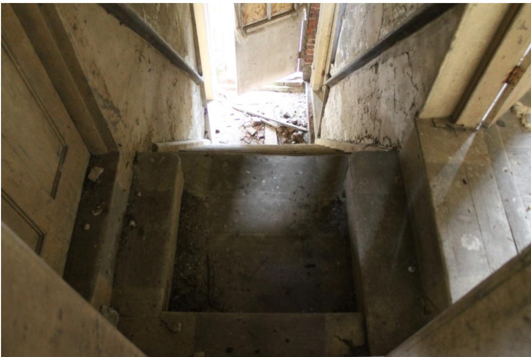
Plate 19 First floor landing with bedroom 1 to the left and bedroom 2 to the right
