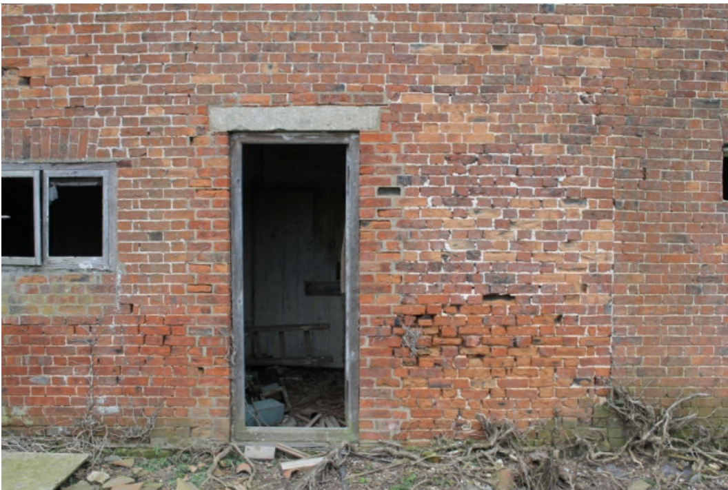
Plate 15 Scullery exterior showing relocated doorway - view east
