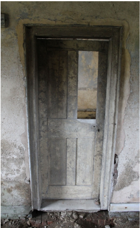
Plate 12 Original door to dining room – view east
