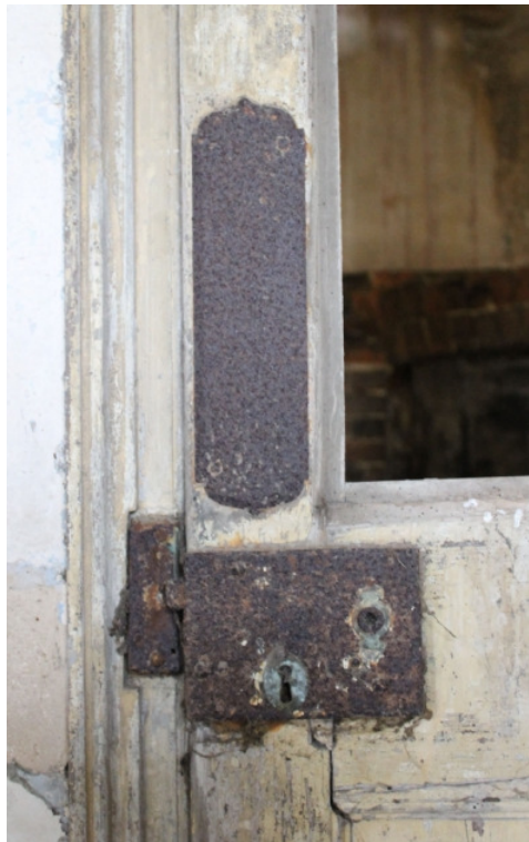
Plate 13 Detail of original door furniture - view west
