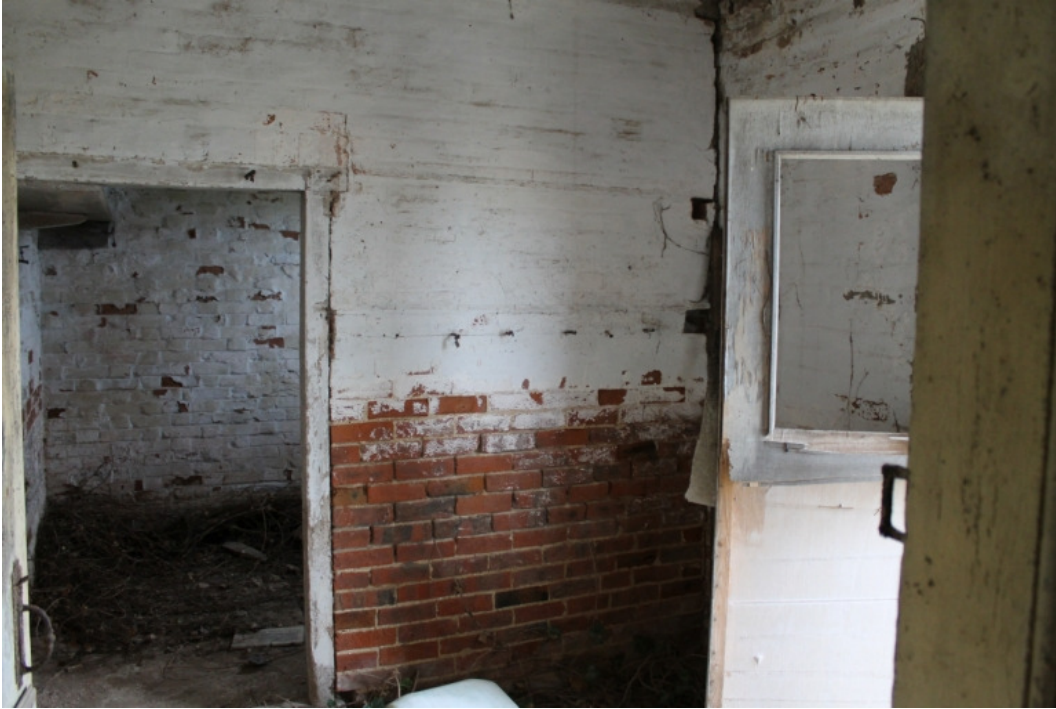
Plate 14 Scullery, with inserted dividing wall and relocated doorway – view south
