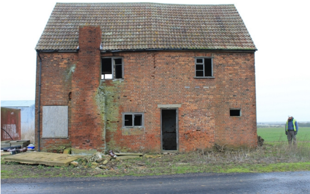
Plate 2 West elevation – view east
