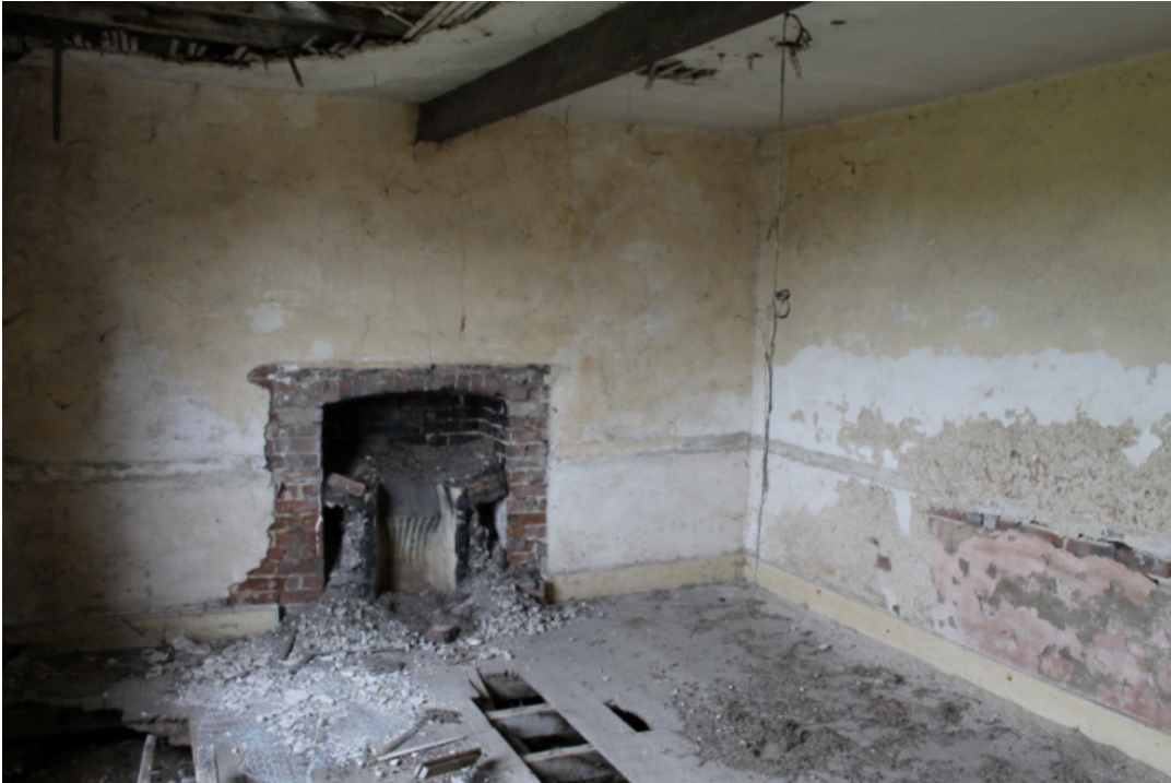
Plate 18 Parlour with remains of fireplace and bridging beam – view south-west
