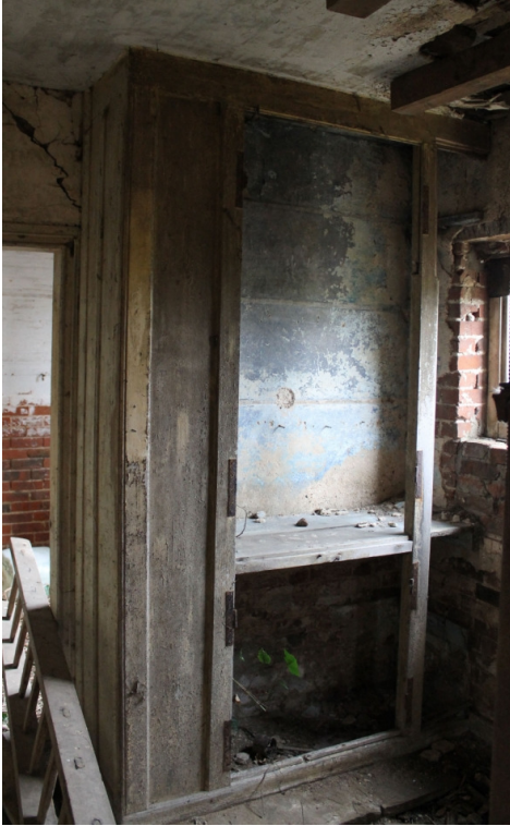
Plate 10 Original kitchen cupboard - view south-west
