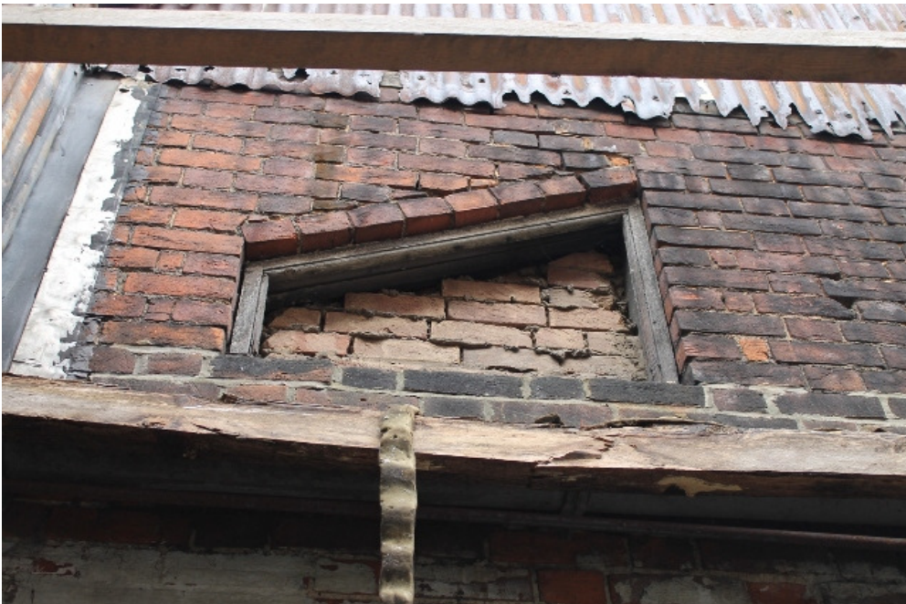
Plate 4 The rebuilt first floor wall of the converted 1830 house, showing the irregular-shaped window – view north
