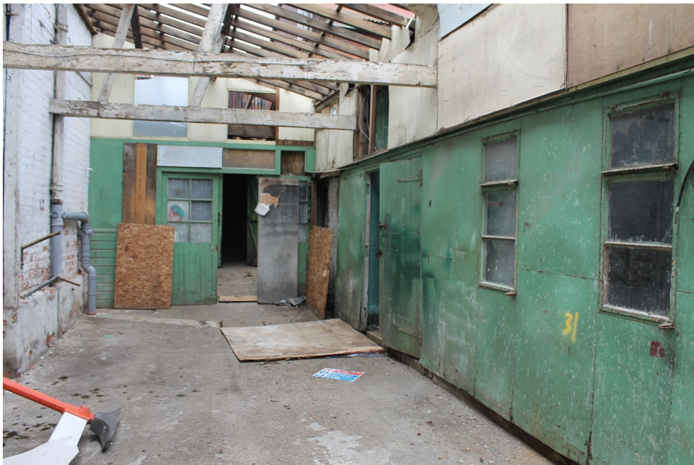
Plate 13 Inserted metal-framed windows in the south wall of the wooden shed – view west
