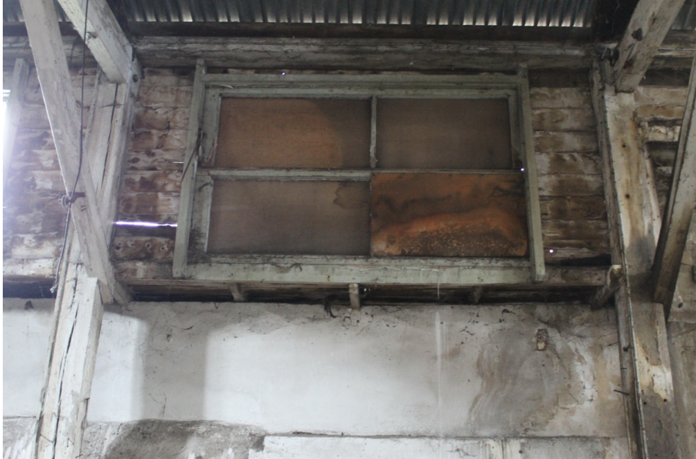
Plate 10 North wall of the workshop, showing the structure built on the adjoining property wall - view north
