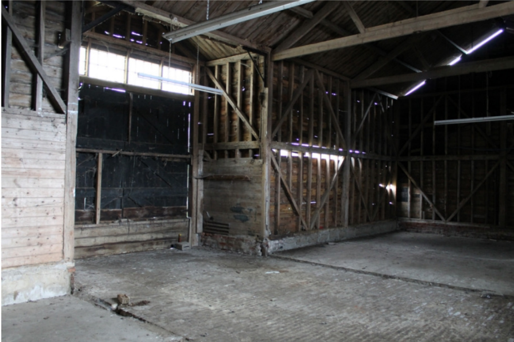
Plate 5 Interior of the barn showing the midstreay threshold leap and brick threshing floor – view east
