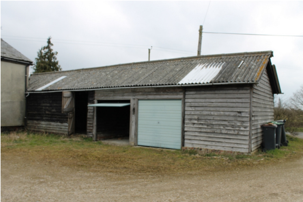
Plate 9 Stable block with converted two-bayed horse shed to the right and carhorse stable to the left of the Henderson garage doors
