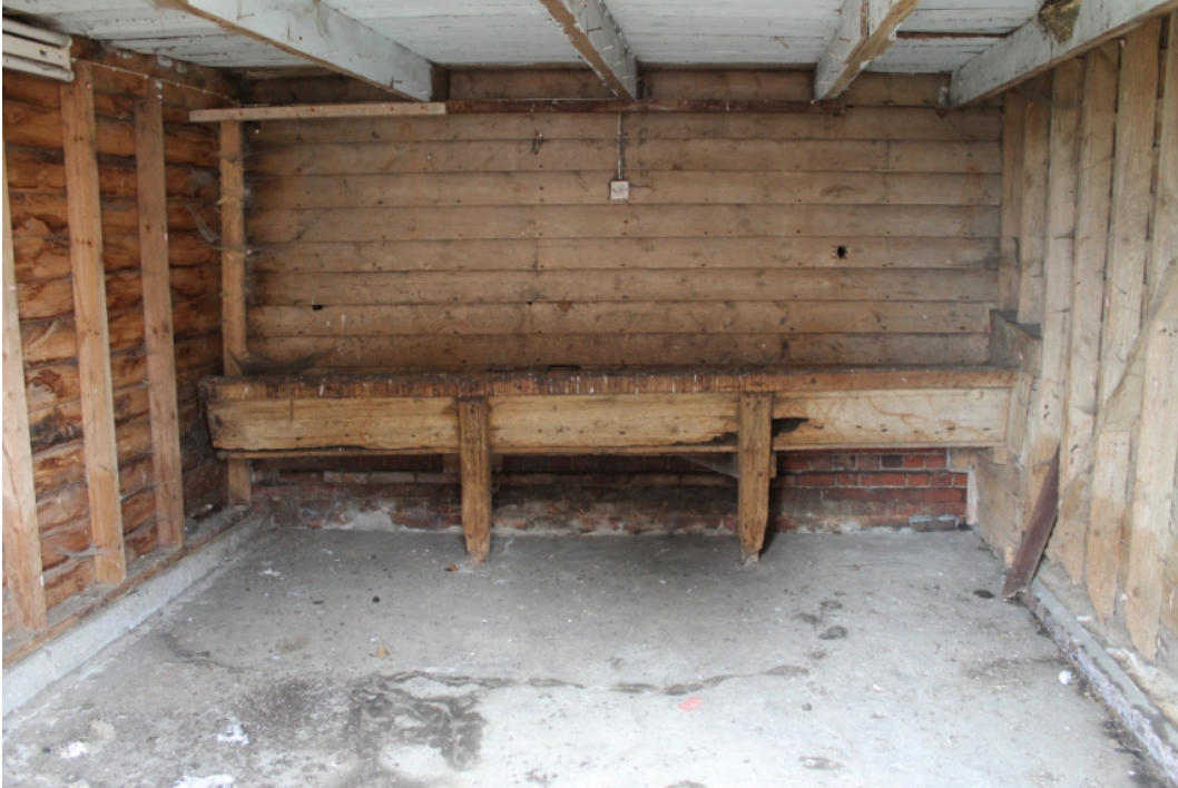
Plate 24 Lean-to cattle shed showing manger with chaff loft above – view north-west
