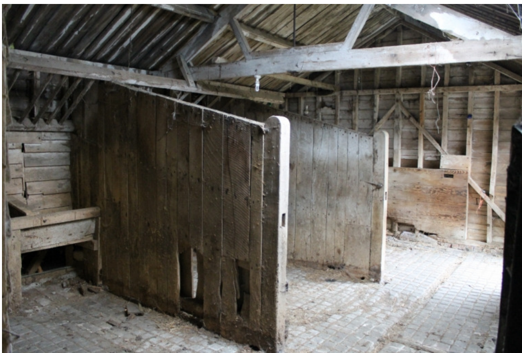
Plate 11 Stable block showing interior of carthorse stable – view south-east
