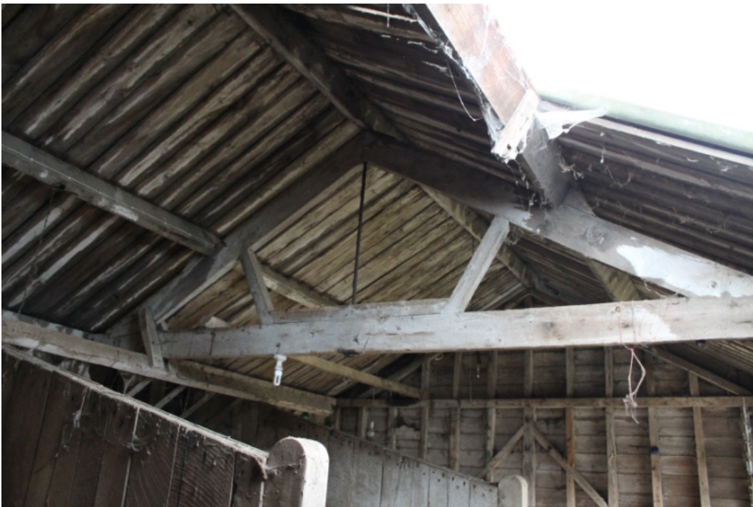
Plate 13 Carthorse stable, truss A - view south-east
