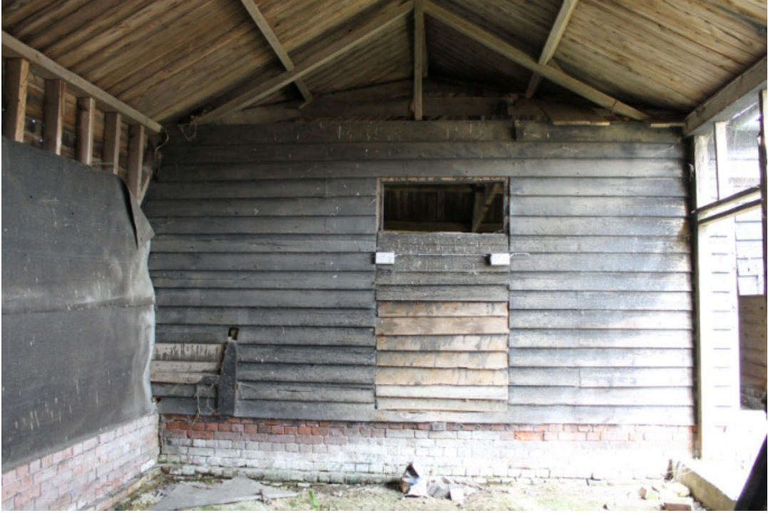
Plate 22 Interior of the 'four-bayed' cattle shed showing the original short king post truss and remains of the manger – view north-west
