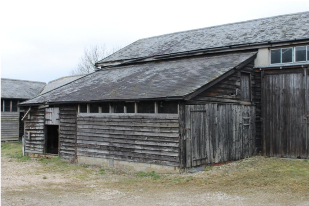
Plate 23 Lean-to cattle shed showing blocked open front and door to chaff loft - view north-west
