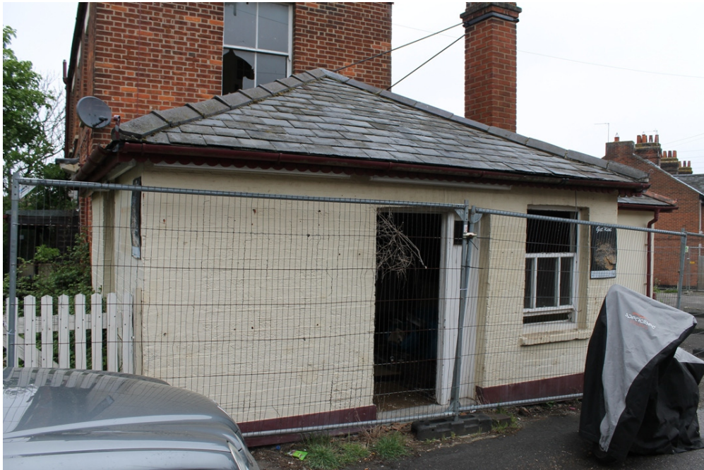
Plate 15 Phase 2 extension - view north
