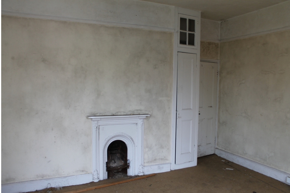
Plate 12 Bedroom with register grate, picture rail, later fitted cupboard and original door – view north-east
