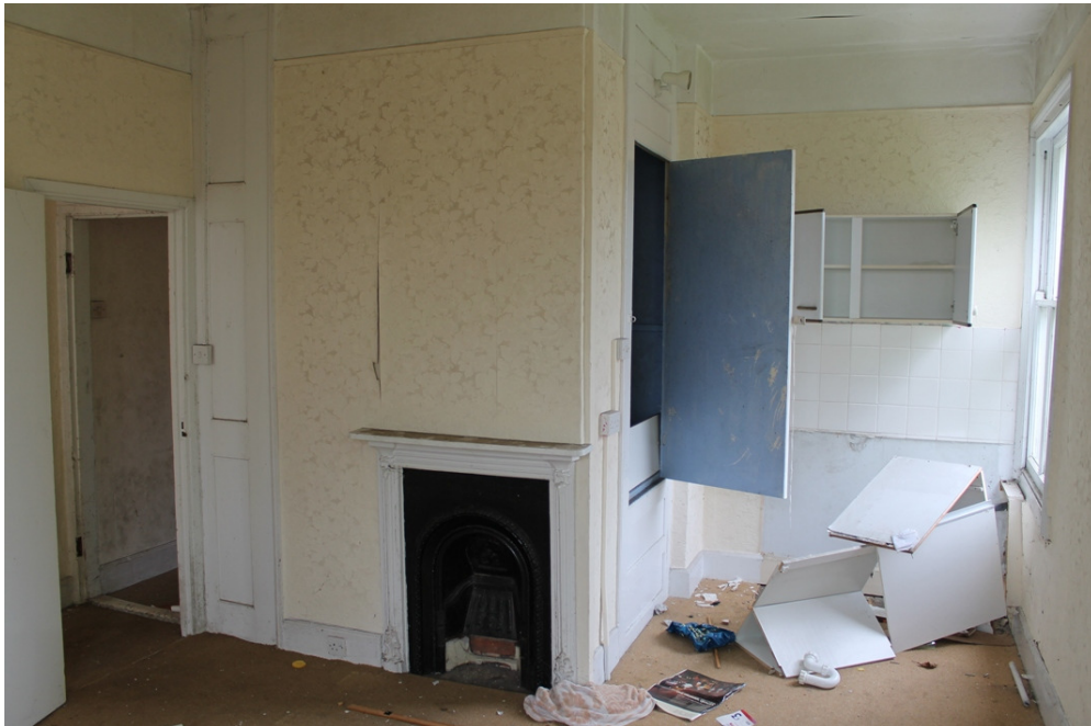
Plate 13 Living room, with the inserted stud wall to the left, the register grate and the cupboard above the stairs - view south-east
