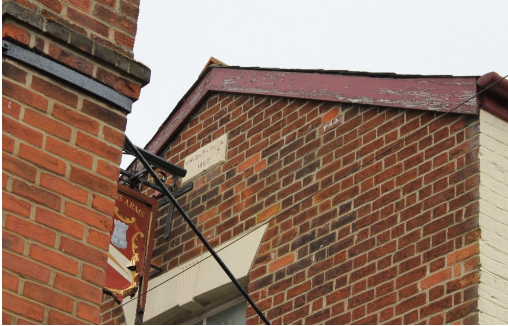
Plate 3 South elevation showing date stone – view north-west
