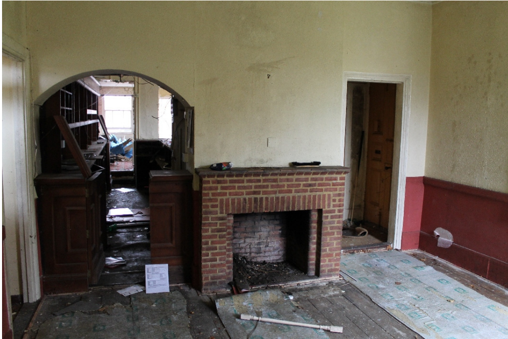
Plate 7 The back bar, with rebuilt fireplace and exposed original floorboards – view south
