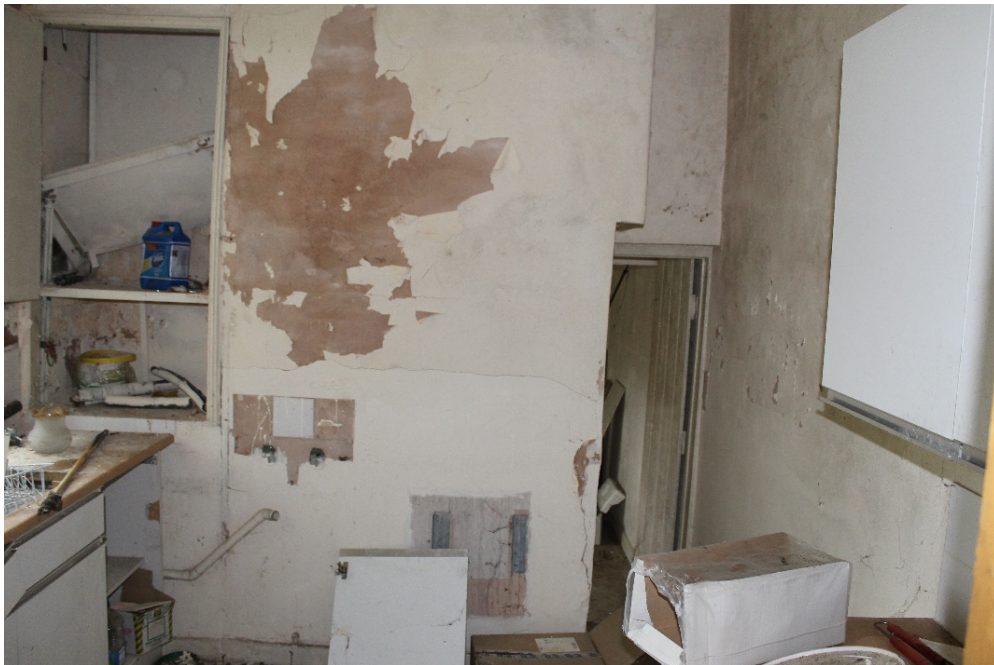
Plate 8 The service wing, showing the kitchen with its blocked fireplace and the inserted phase 3 doorway – view north-west
