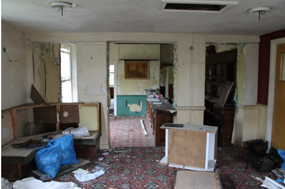
Plate 5 Interior of the bar, seen from the phase 2 extension looking into Wright Villa – view north-west
