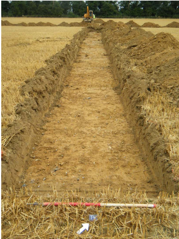
Plate 5: T4, view NW. T3 and T2 behind.
