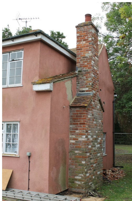
Plate 14 Phase 2 single-storey extension with the Phase 3 second storey extension above – view south-west
