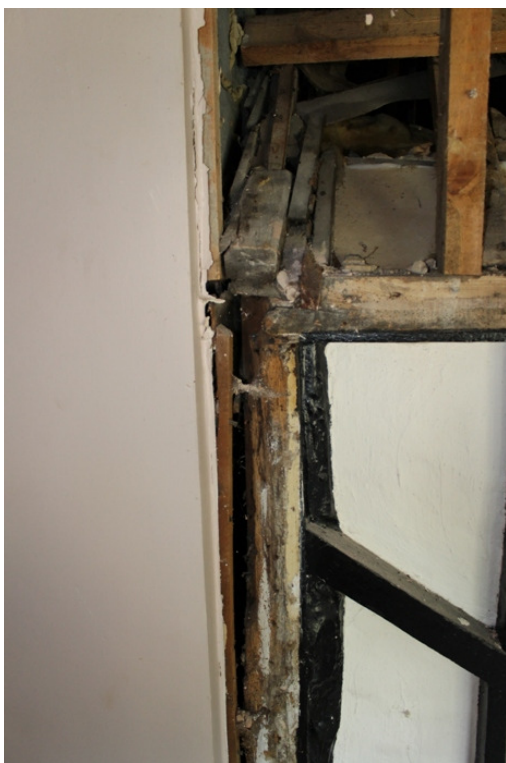
Plate 13 The south gable with 1979 extension to the left – view west
