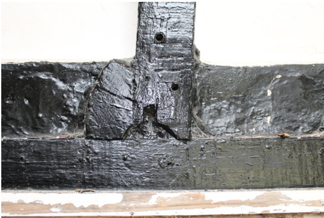
Plate 12 Example of a carpenter's mark (III) on the base of a stud in the east wall of the first floor frame, with the butt end of a floor joist carried on the girt - view west
