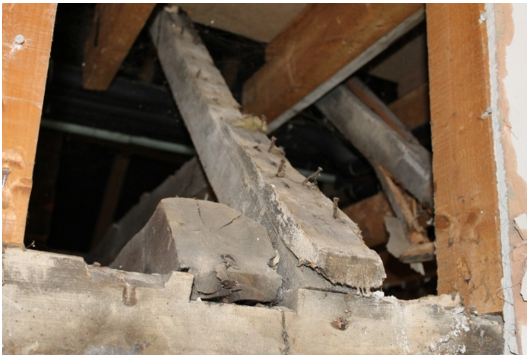
Plate 10 Original rafter with firing piece nailed to it and end of relocated tie beam – view north-west
