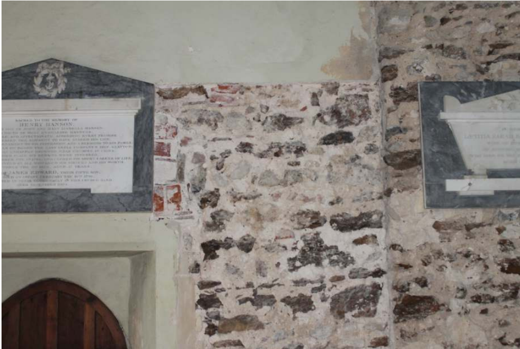
This photograph is farther along the south aisle wall than the previous two. It appears to show two different building styles (ie, periods) near this small door. To the right is older work (original south aisle?) and to the left is more recent work with the external door (extension to south aisle).
