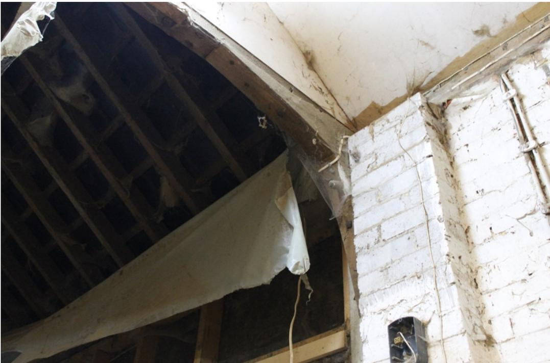
**Plate 8** Bolted knee brace to truss B of bay 2 and brick pier of the wall – view north-east
