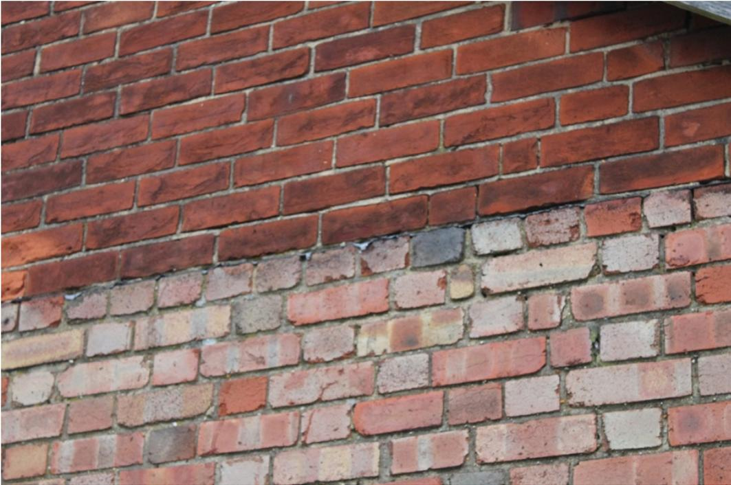
**Plate 5** Remains of lead flashing between the Fletton bricks and soft reds of the gable on the south-east elevation of the brick barn, indicative of a mono-pitch lean-to - view north
