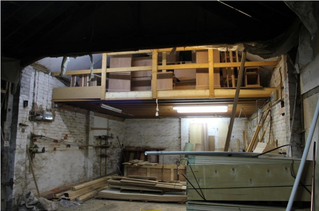
**Plate 7** The interior of the brick barn, showing the modern mezzanine blocking the pitching door – view north-west
