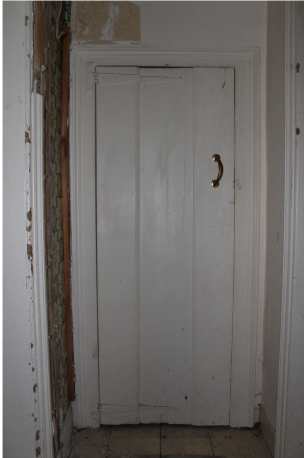
Plate 21 Cupboard at head of Phase 3 staircase with original plank door – view west
