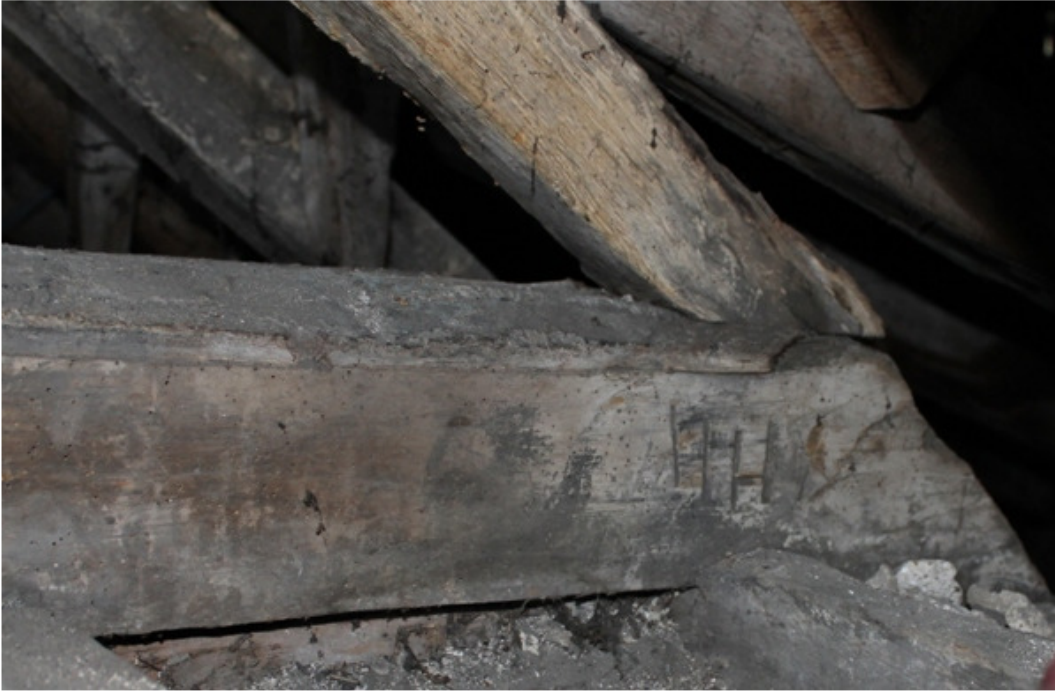
Plate 23 Chiselled carpenter's mark on the end of an attic tie beam – view north-west.
