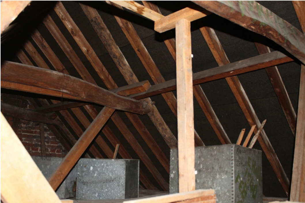
Plate 22 Detail of the roof timbers, showing original Phase 1 principal rafter and collar and modern inclined queen post, purlin and common rafters – view south-east
