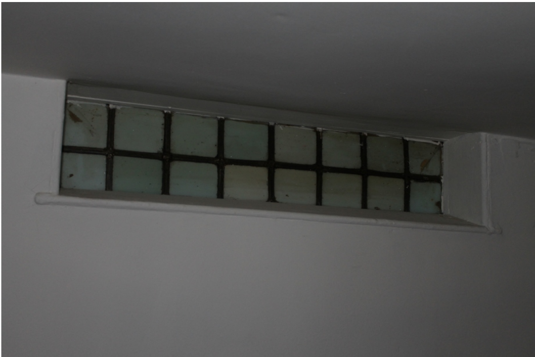
Plate 20 Leaded light window in dividing wall between bedrooms 3 and 5 – view south-west
