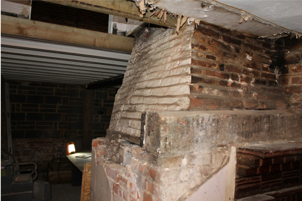
Plate 9 The original Phase 1 chimney between the dining area and the bar, with the stepped brickwork of the stack and the cambered timber mantel - view north-west.
