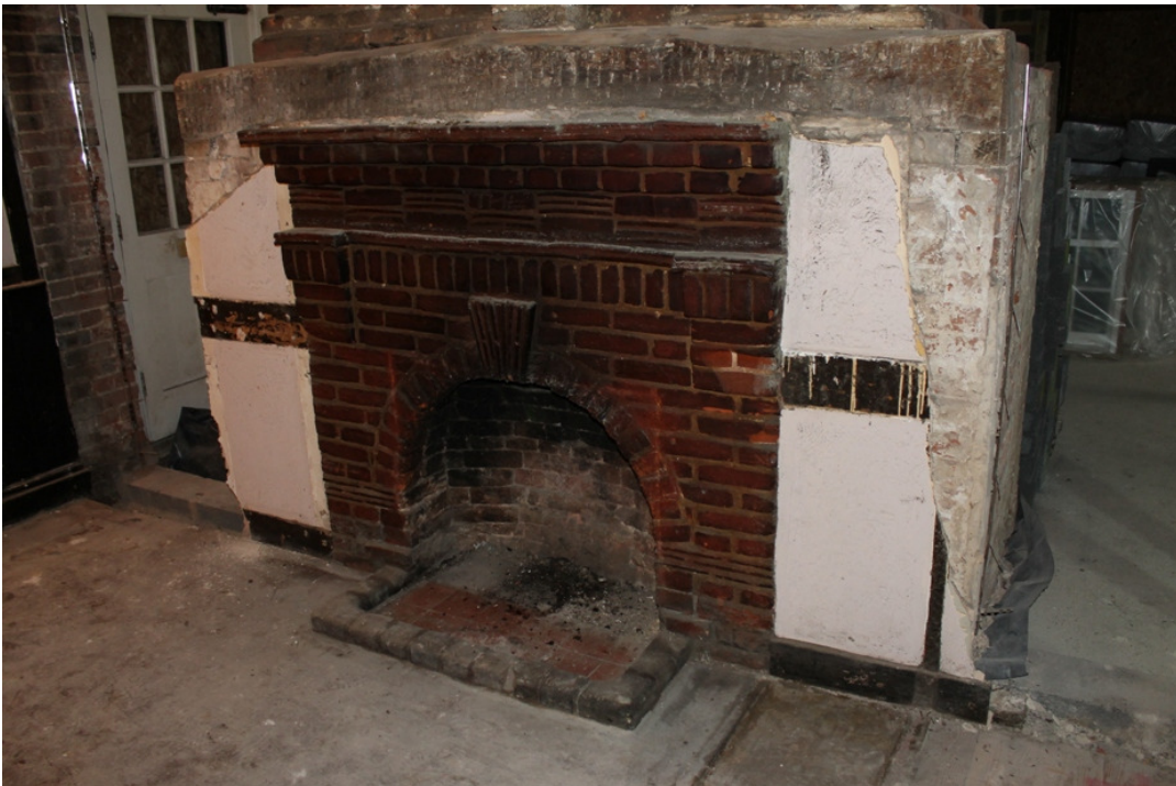
Plate 10 Art Deco fireplace inserted to the Phase 1 chimney, with Phase 5 render and mock timber framing – view south-west
