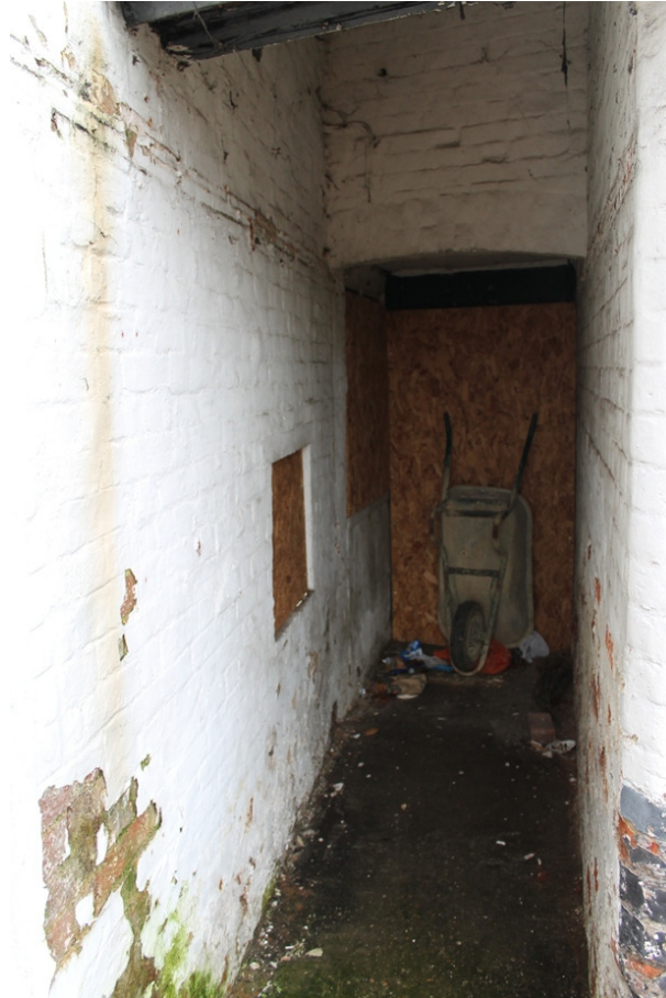
Plate 13 Phase 4 passage way leading from yard into Phase 3 extension, showing the arch for the original doorway to the extension – view south-east
