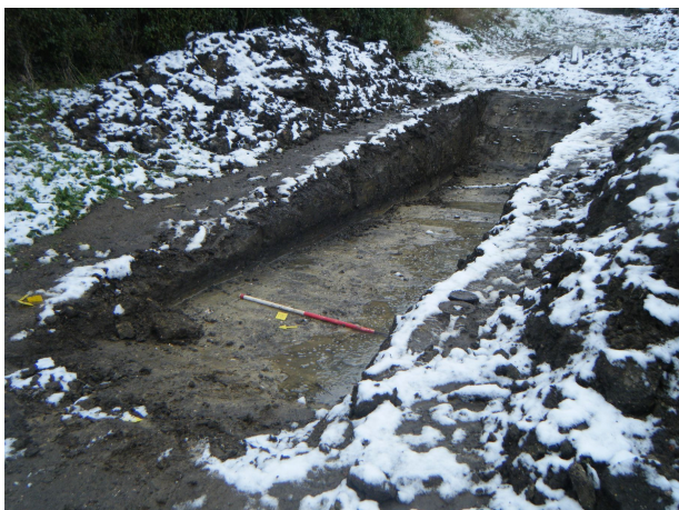
Photograph 1 Trench T3, looking SE
