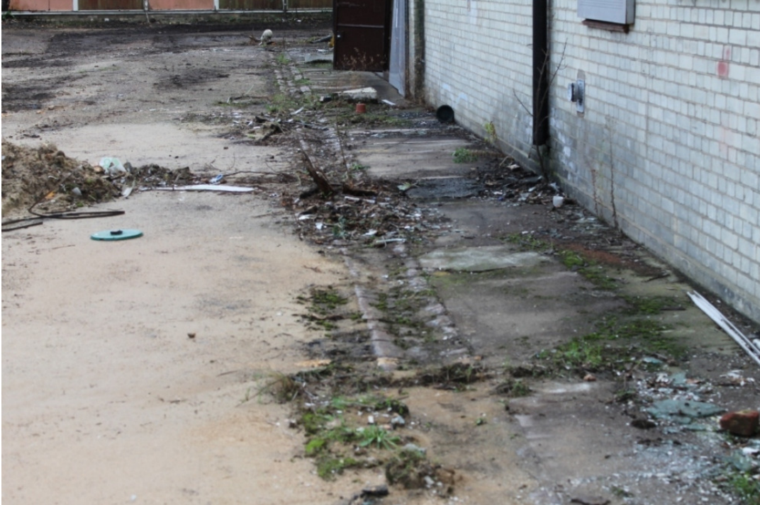
Plate 21 Original granite-lined drainage gully extending the full length of FLG 10/11 - view south
