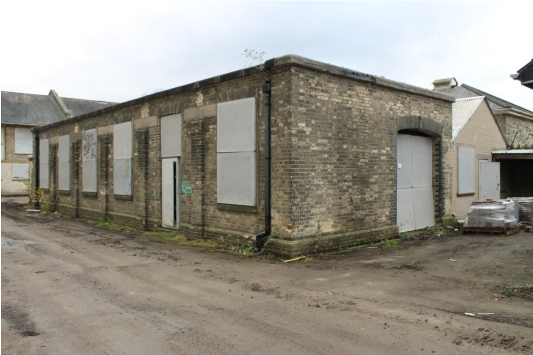
Plate 11 Building 3, flat-roofed brick shed with building 3a to the right – view south-east
