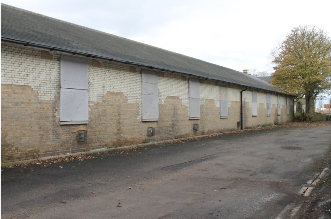
Plate 19 West elevation of FLG 10/11 showing the increased height of the brickwork and the windows which were inserted to the elevation at the same time - view south-east
