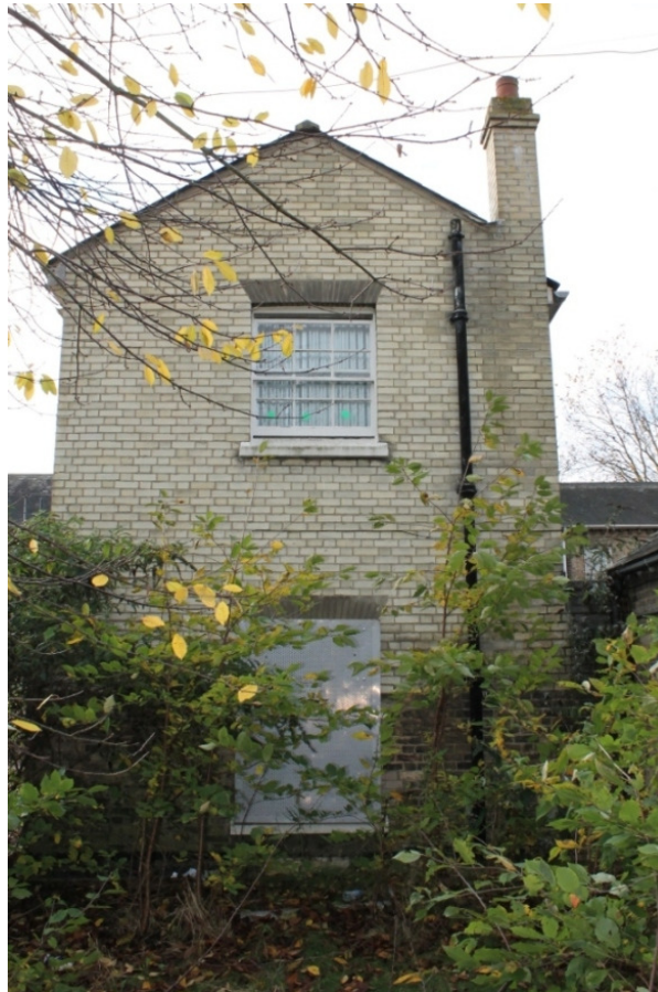
Plate 2 East elevation of the Annexe showing the Phase 4 extension constructed on top of an earlier wall – view west
