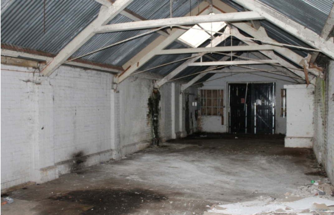
Plate 15 Interior of Building 3a showing the timber roof trusses supported on the south wall of Building 3 and the boundary wall to the right – view north-east
