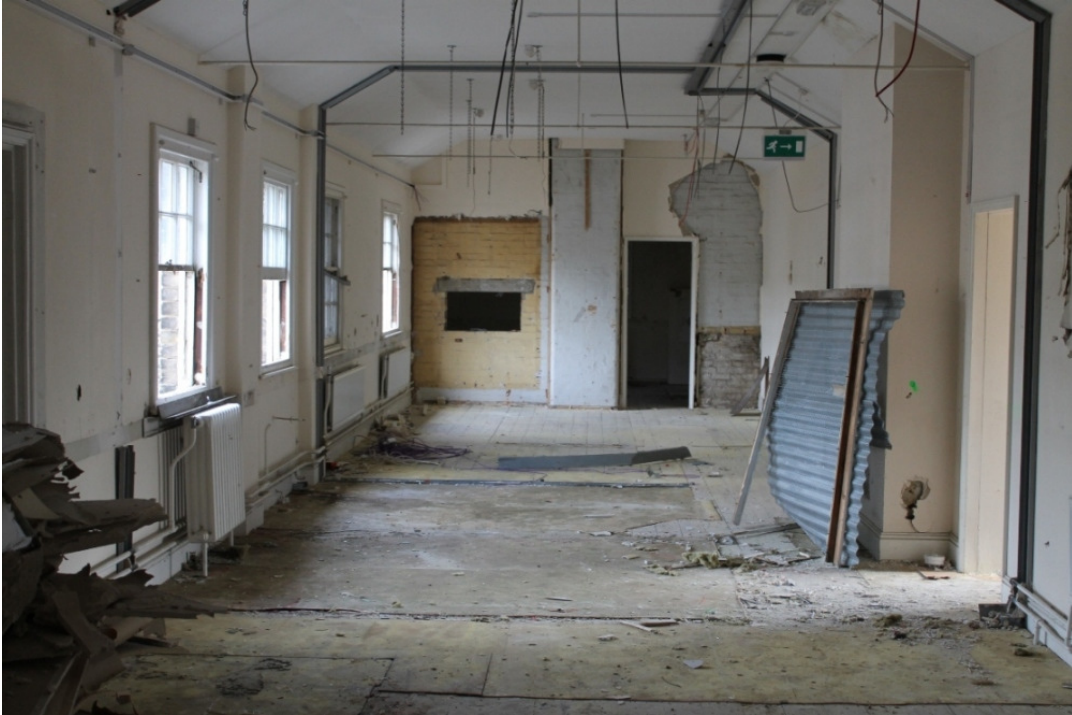
Plate 7 First floor of the Annexe with the Phase 4 extension to the rear - view east
