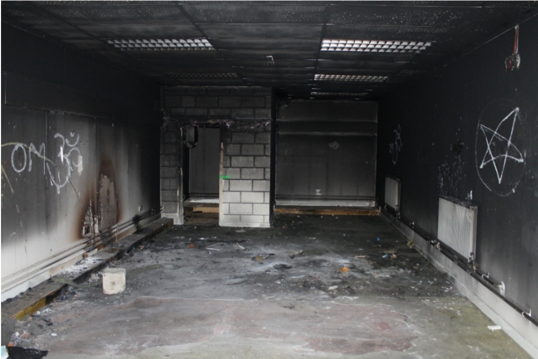
Plate 29 Interior of FLG 12 Room 1, possibly used as a foyer for the cinema next door - view east
