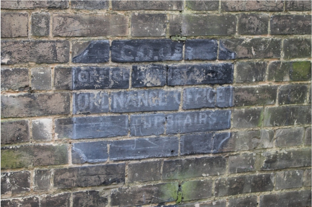
Plate 3 Painted sign on the east elevation of the Annexe
