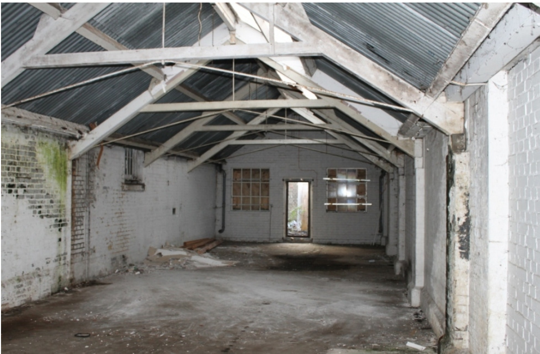
Plate 16 Interior of Building 3a showing the timber roof trusses and the blocked window to FLG 17 on the left – view south-west
