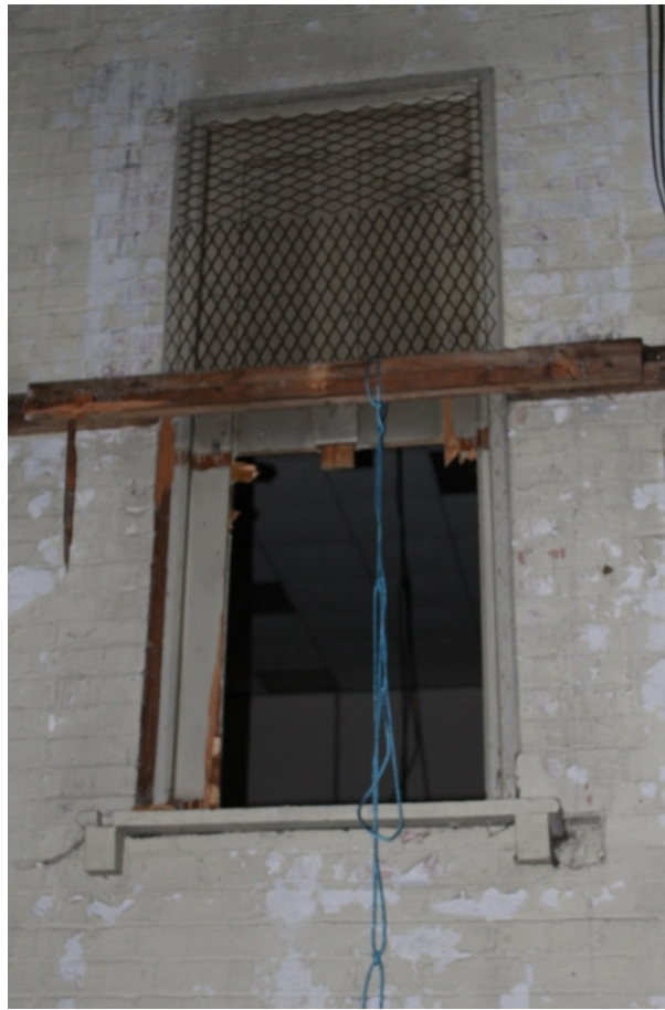
Plate 24 Doorway in the dividing wall between FLG 10 and the building to the north - view north
