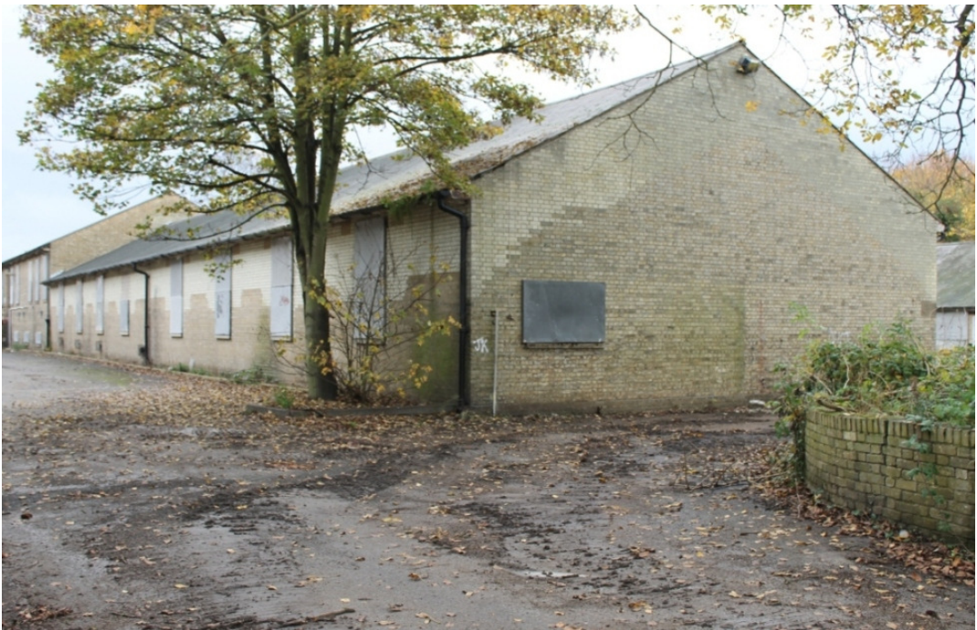
Plate 20 South elevation of FLG 10/11 showing the increased height of the brickwork and a later inserted window - view north-east
