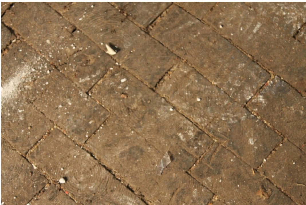
Plate 17 Detail of wooden parquet floor to Building 3a
