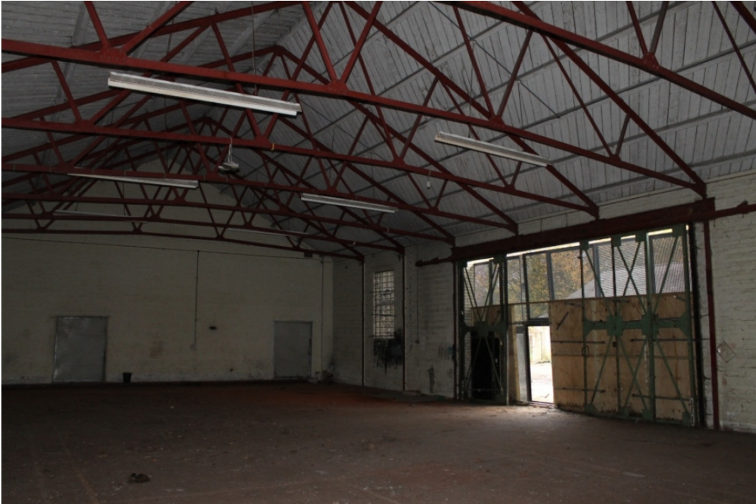
Plate 23 The interior of FLG 11 showing the original steel roof trusses supporting the diagonal sarking boards of the roof and the badminton court painted on the floor - view north-east
