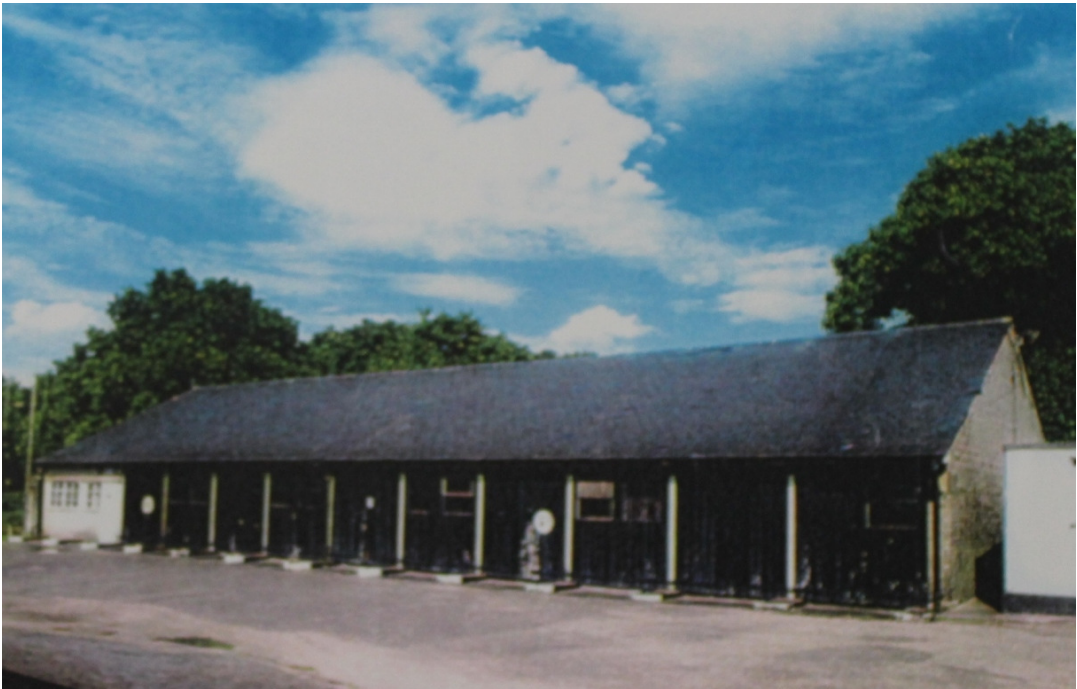
Plate 26 West elevation of FLG 12/13 photographed in 2000 showing the original wagon doors extending along the length of the façade - view north-east (copyright Ingrams, 2000)
