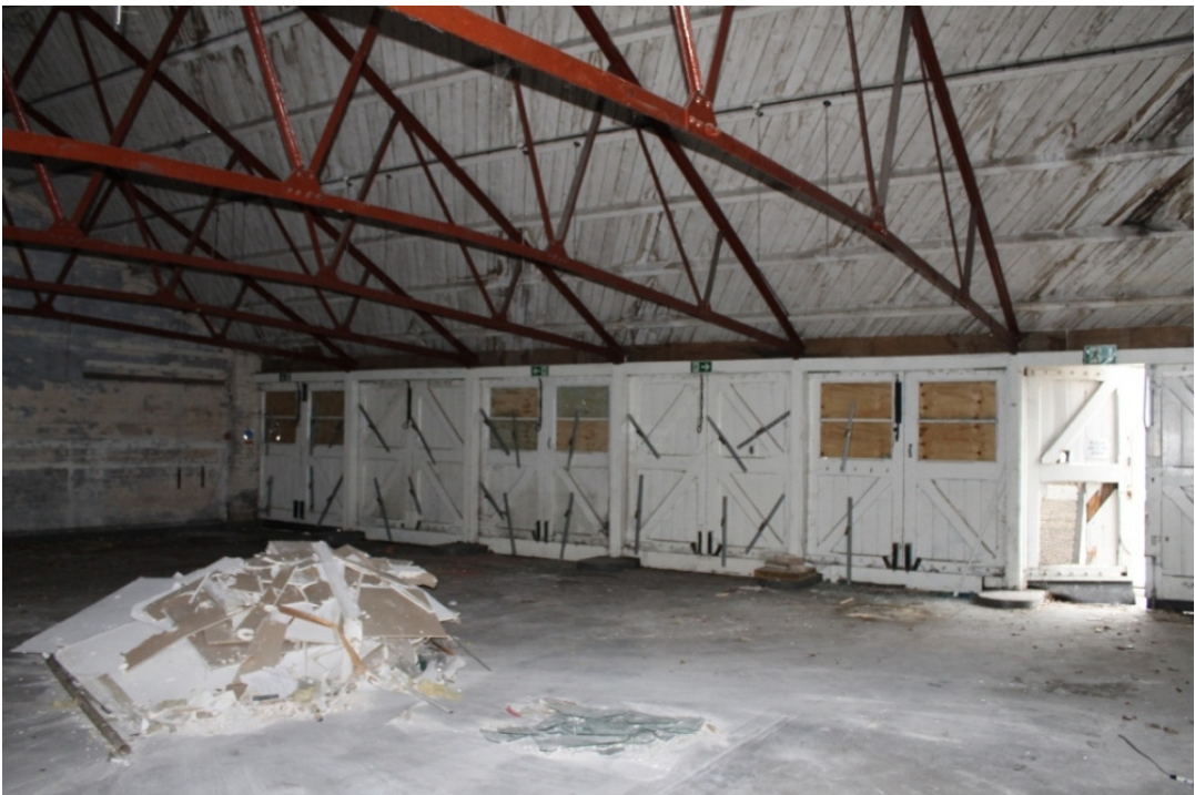
Plate 28 Interior of FLG 13 showing original wagon doors, steel roof trusses and diagonal sarking boards - view south-west
