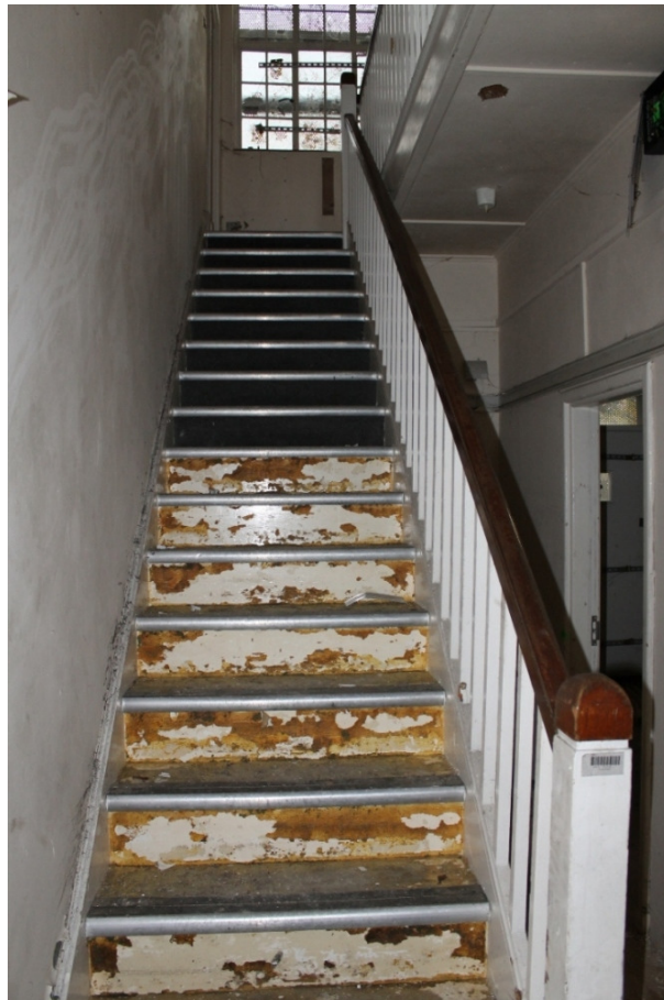
Plate 10 FLG 2 stairs to the first floor – view south
