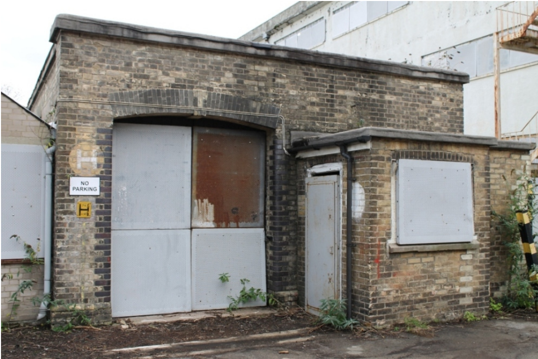
Plate 13 East elevation of Building 3 showing the wagon doors with jambs constructed from blue bricks with rounded edges - view west
