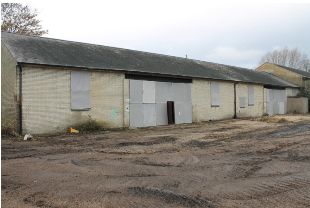
Plate 18 East elevation of FLG 10/11 showing the infilled front and raised roofline - view north-west
