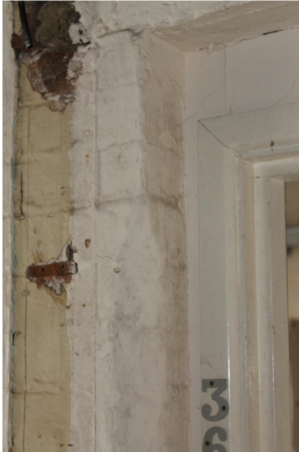
Plate 5 Chamfered brick door jamb in dividing wall of the ground floor to the Annexe - view north-west
