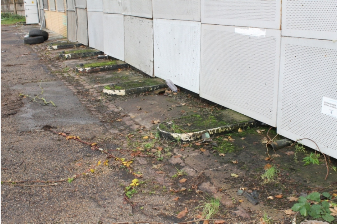
Plate 27 West elevation of FLG 12/13 showing the original granite-lined drainage gully in front of the wagon doors - view north-east
