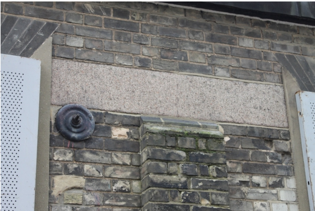
Plate 12 North elevation of Building 3 showing one of the granite pads above a brick buttress which carry the I-beams of the flat roof – view south
