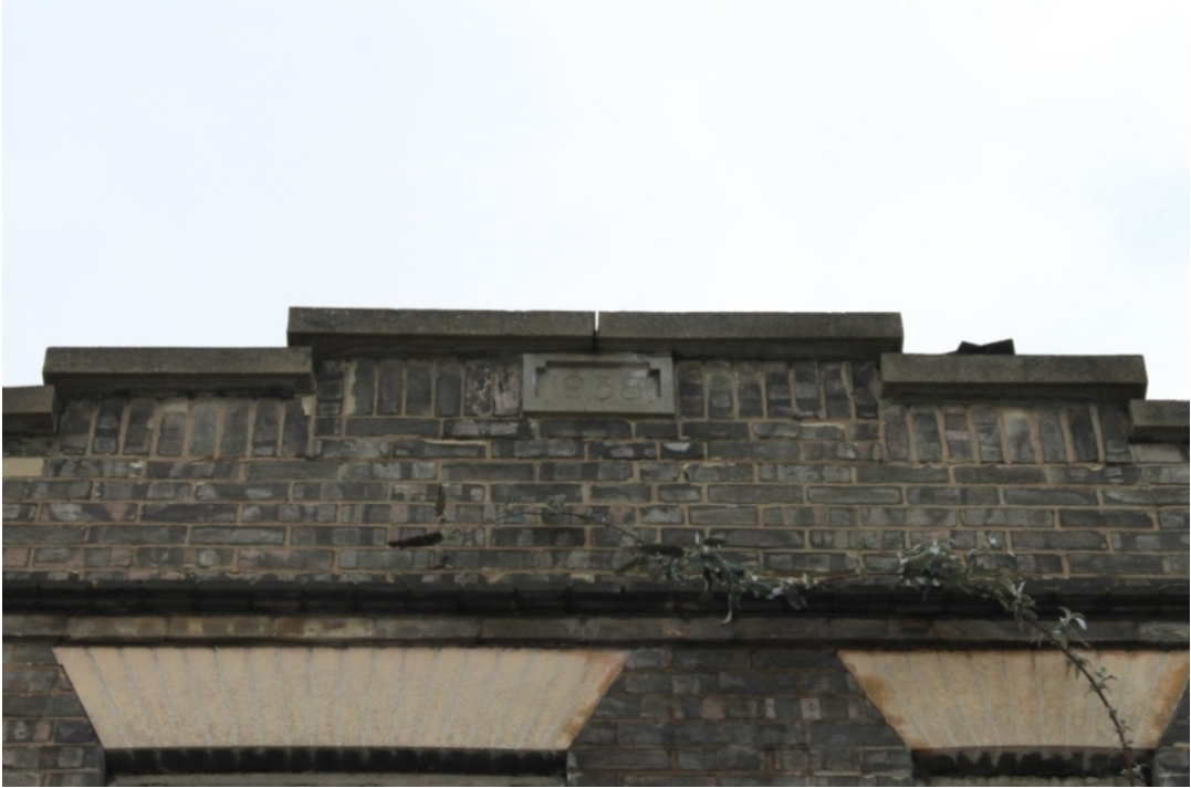
Plate 9 North elevation of FLG 2 showing the date stone marked 1938 below the stepped section of the parapet - view south
