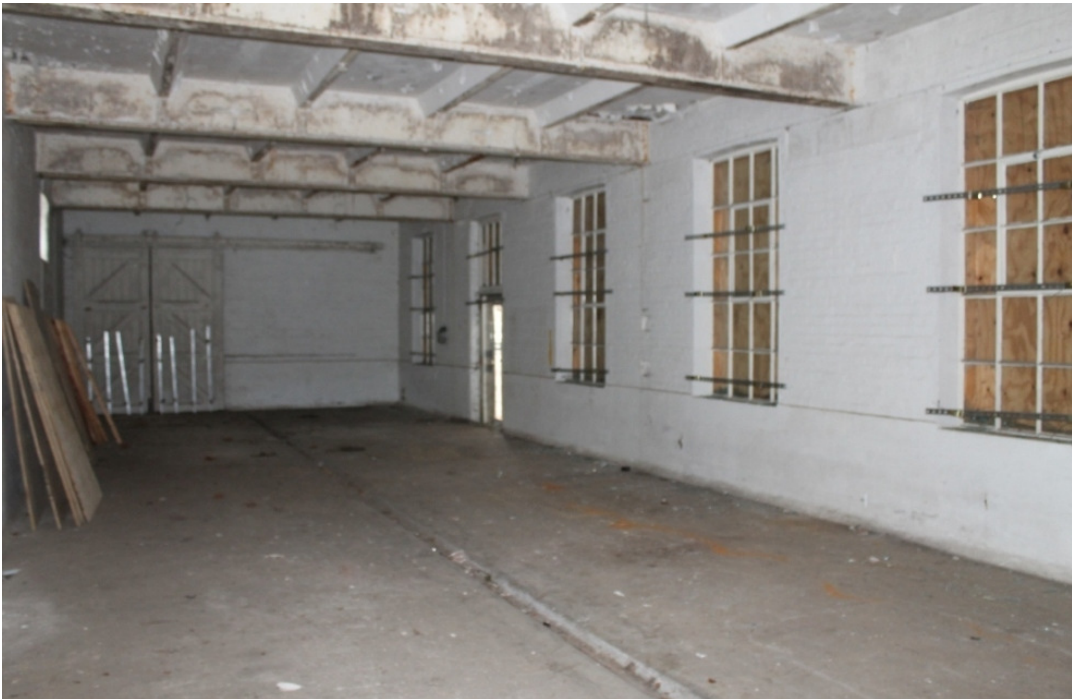
Plate 14 Interior of Building 3 showing the sliding wagon doors, the metal-framed windows, the I-beams carrying the flat roof and the drainage gully in the floor – view north-west
