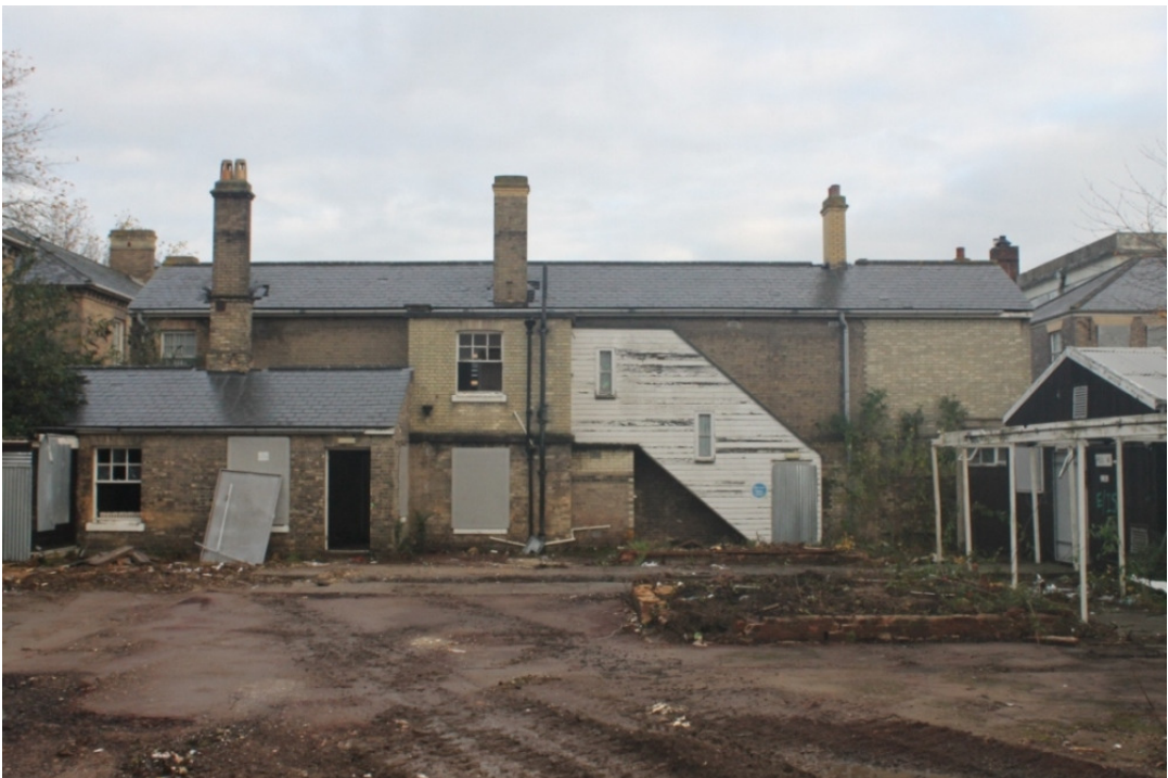
Plate 4 South elevation of the Annexe showing the extensions to the rear of the range - view north
