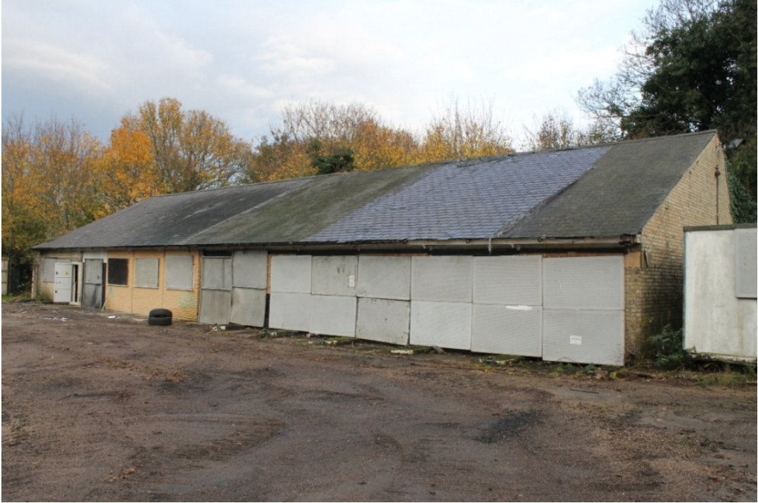
Plate 25 West elevation of FLG 12/13 showing the alterations to the wagon doors - view north-east
