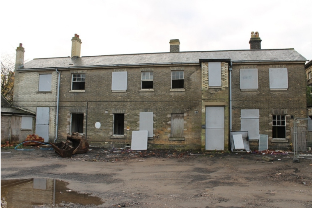
Plate 1 North elevation of the Annexe - view south
