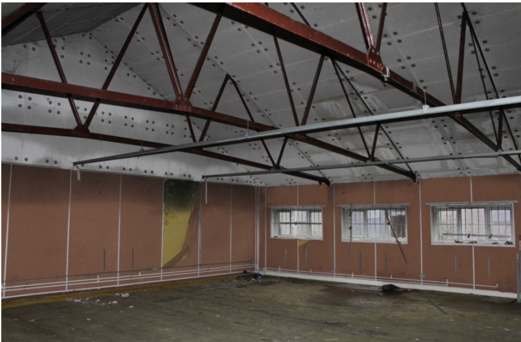
Plate 30 Interior of FLG 12 Room 2, fitted out with sound-proofing for use as a cinema - view south-east
