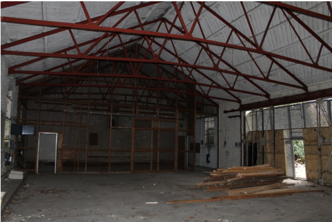
Plate 22 The interior of FLG 10 showing the later caged area to the north and the sliding doors of the modified east elevation. The steel roof trusses supporting the diagonal sarking boards are part of the original building and have been raised to the modified height - view north
