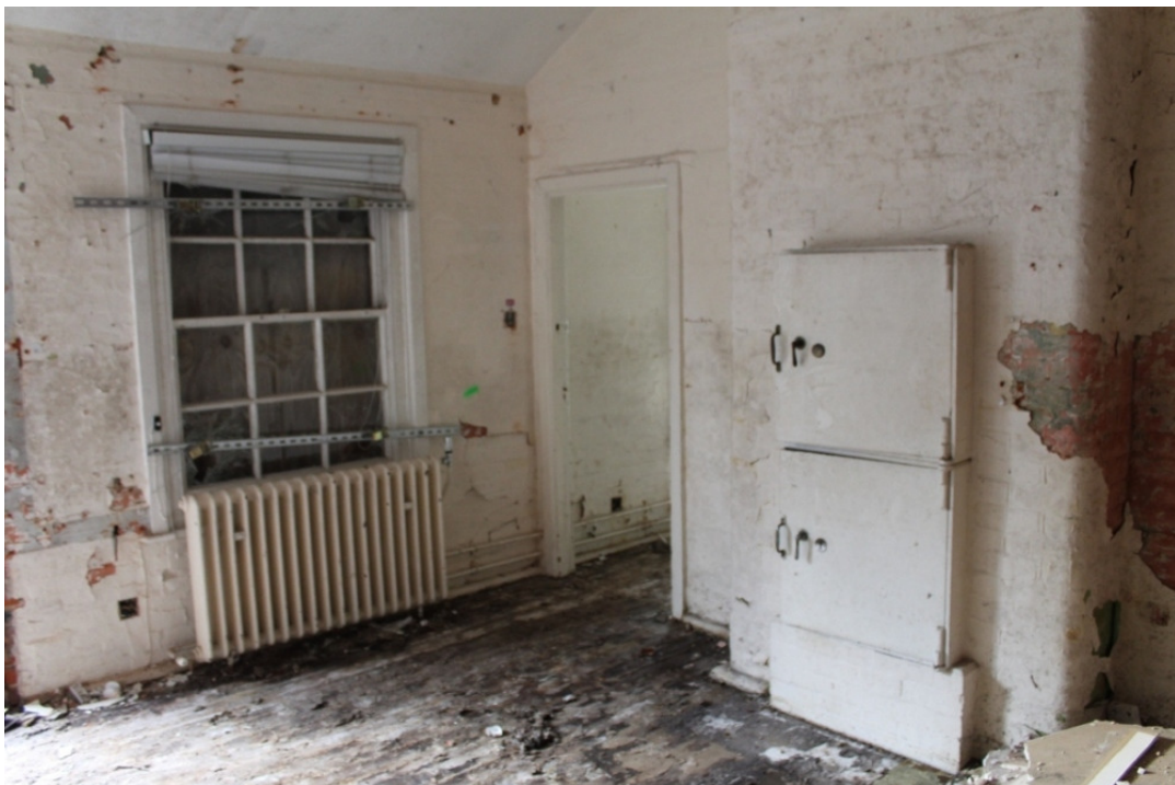
Plate 6 The interior of Room 7 of the Annexe showing the fireplace converted to a double safe – view south-west
