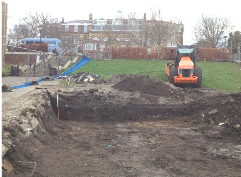
Plate 1: view south towards old College building, showing general level of ground reduction for Student Services building (scale is 1m long)
