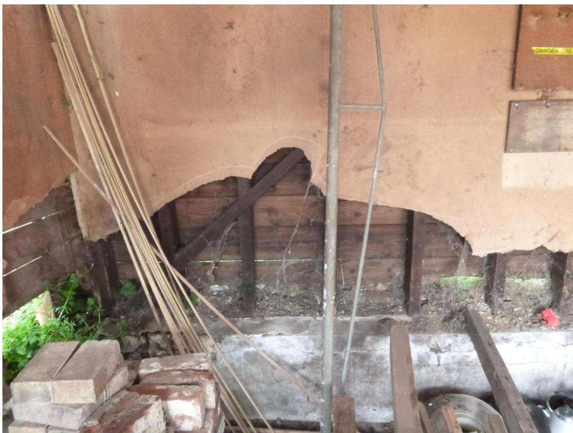
Plate XII Interior shot of outbuilding. Shot taken facing north-west.
