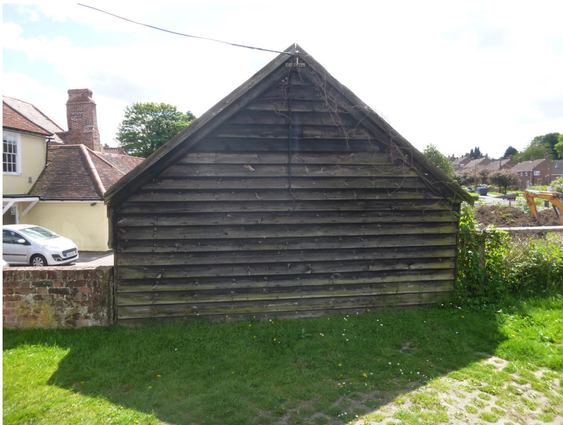
Plate IX North-west elevation of outbuilding. Shot taken facing south-east.
