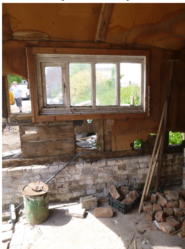
Plate XIII Interior shot of outbuilding. Shot taken facing south-west.
