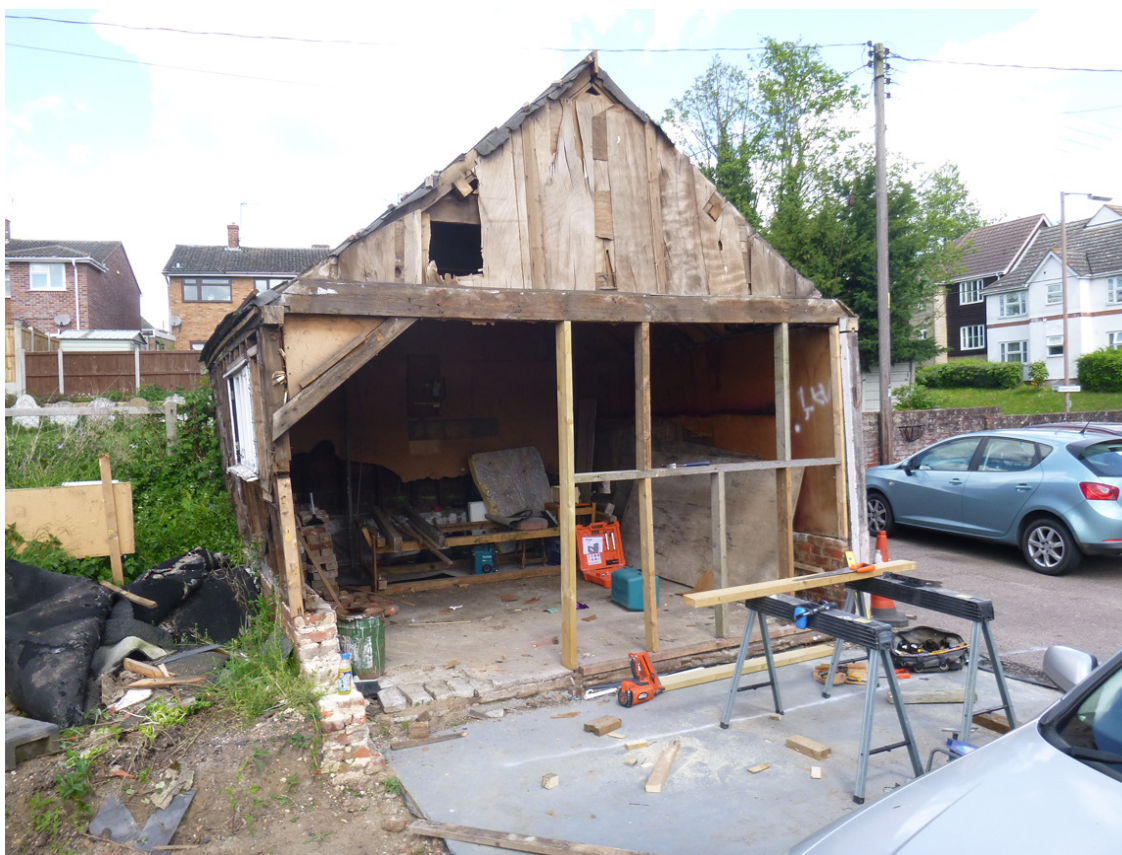
Plate VII South-east elevation of outbuilding. Shot taken facing north-west.
