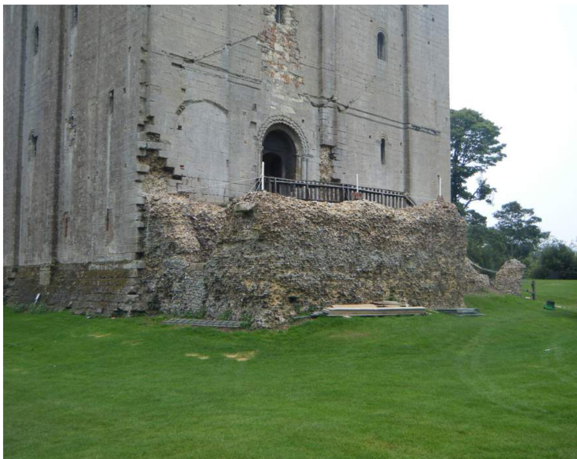
Plate XXXV Fore-building viewed from west. Scars on keep wall show likely height of fore-building when intact.
