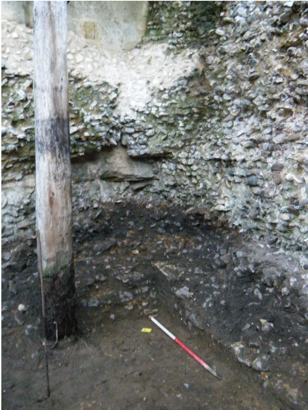
Plate XXX Fore-building interior east corner after lowering of ground level. Small amount of intact facing visible.
