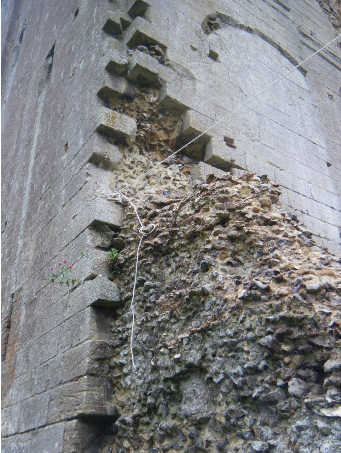
Plate XXXIII North-west corner of keep, showing the removal of ashlar blocks in order to bond the fore-building to the flint and mortar core fabric.
