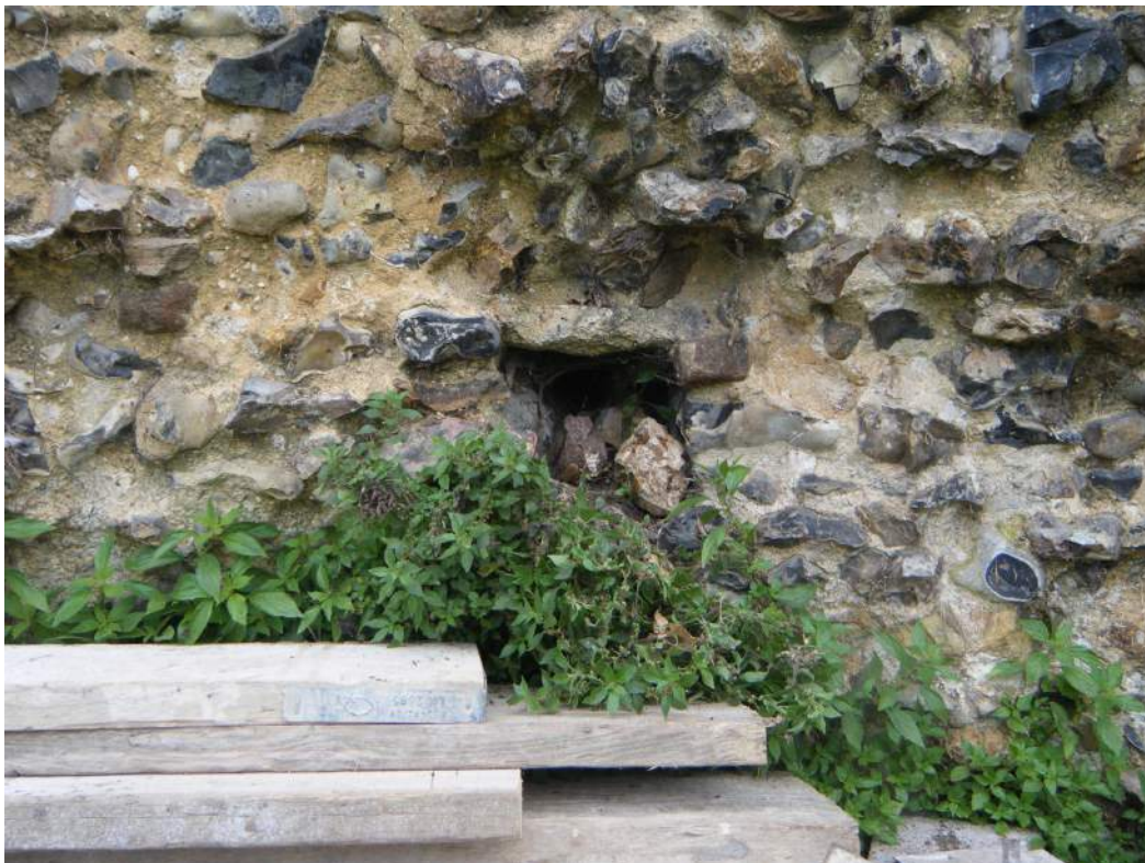
Plate XXIII Close up of putlog hole in south-west elevation.
