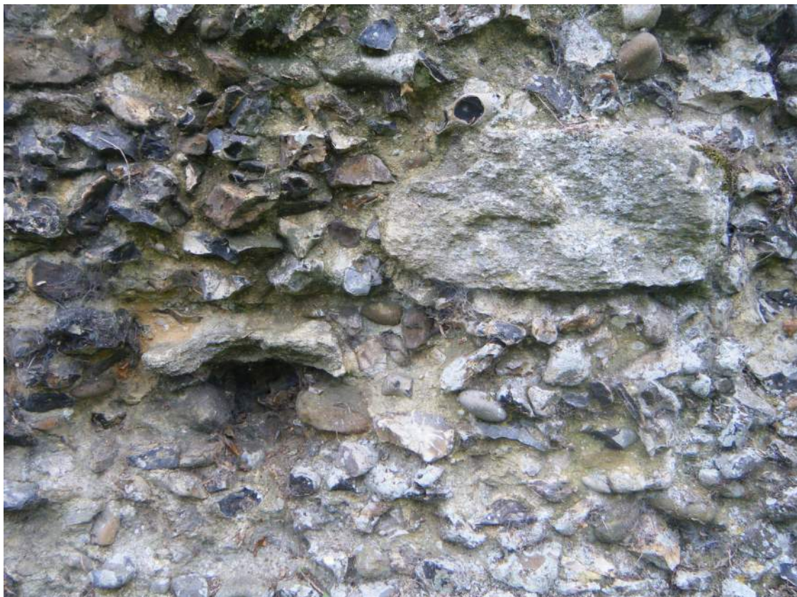
Plate XXI Close up of putlog hole and intact ashlar facing on north-west elevation.
