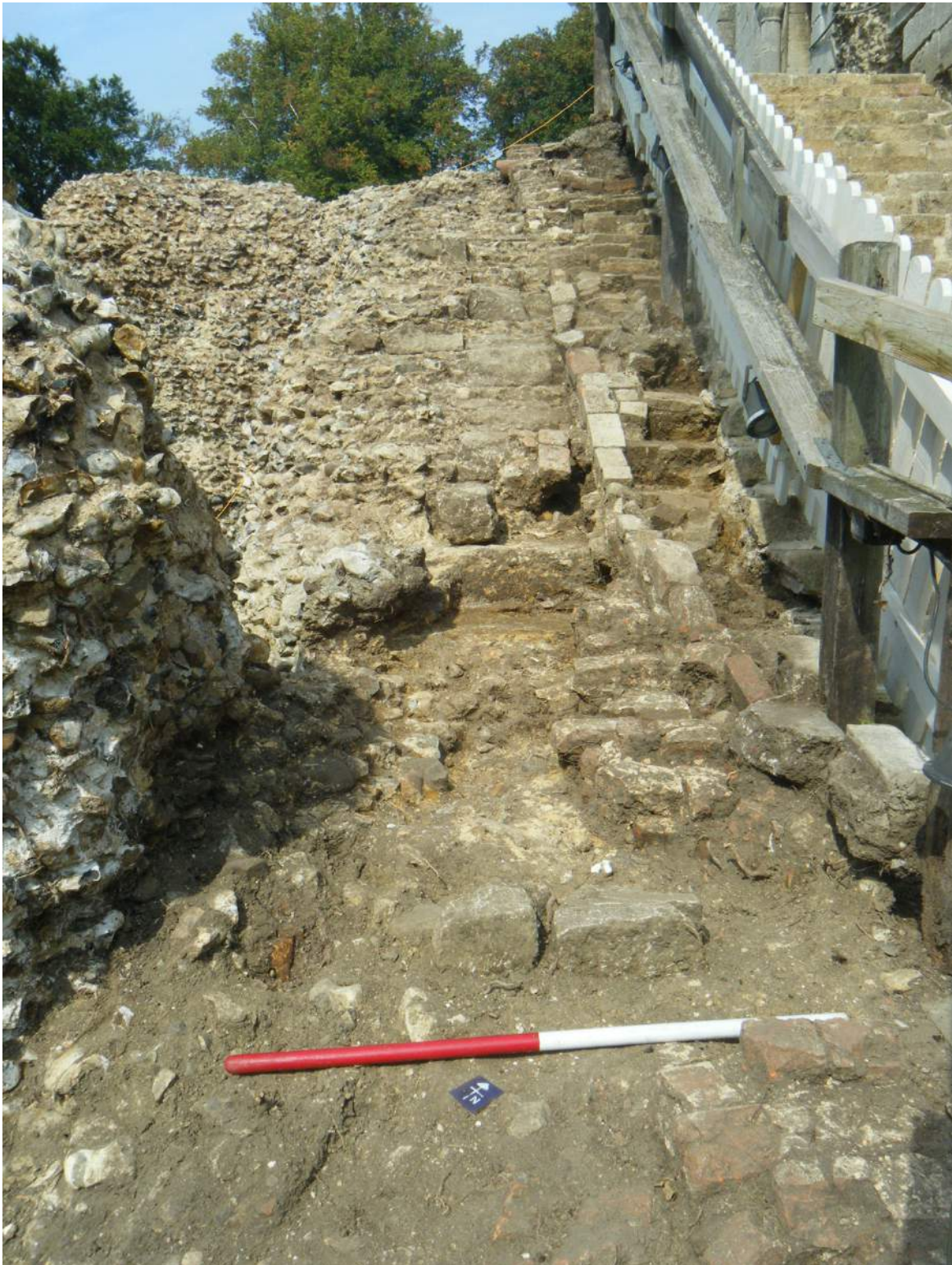
Plate XXXI Stairs fully cleaned and excavated. Original Norman steps visible as well as later post-medieval brickwork. Current stairway to right of frame.
