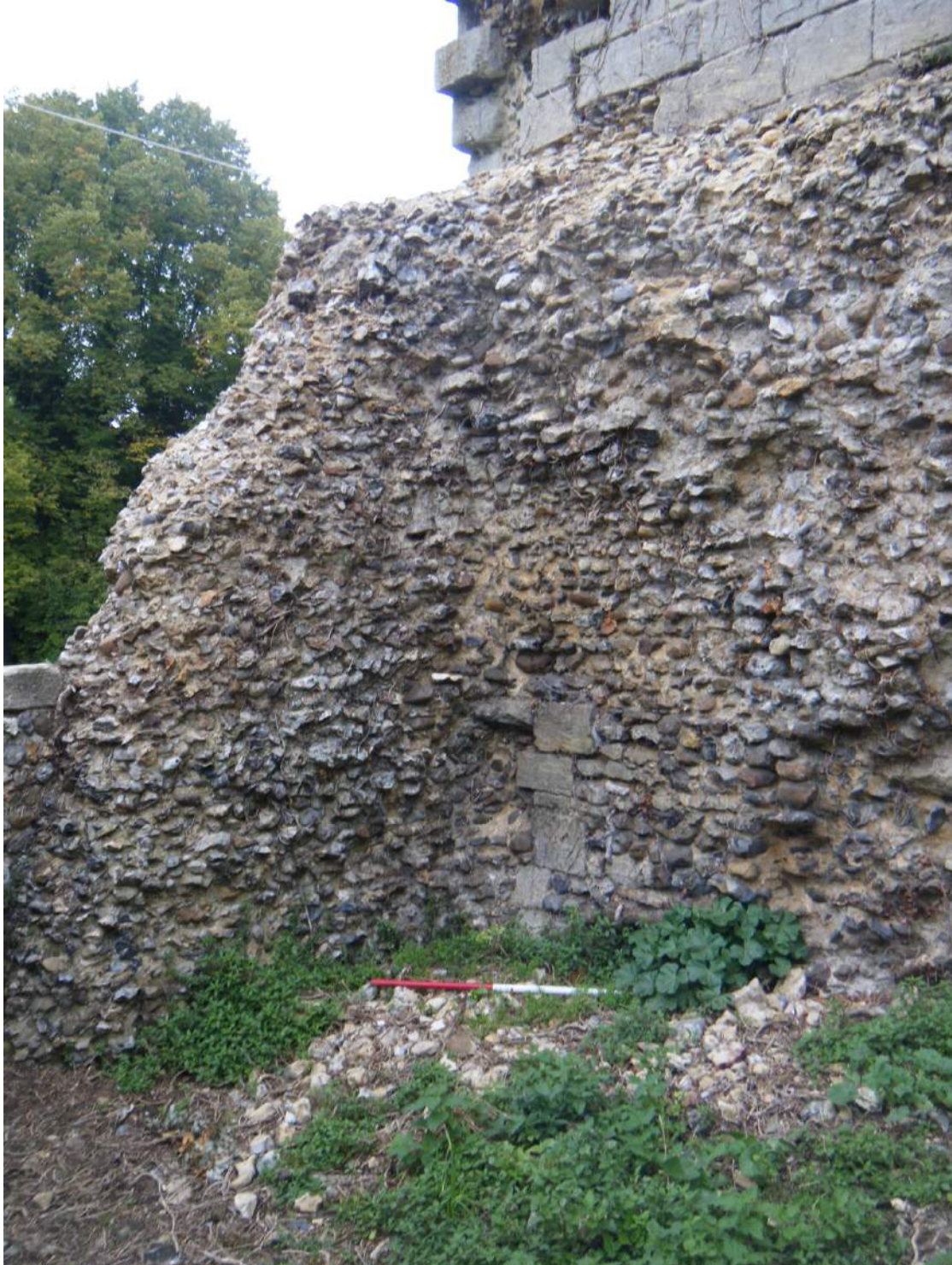
Plate XXIX Interior north-corner of fore-building. Intact facing visible.
