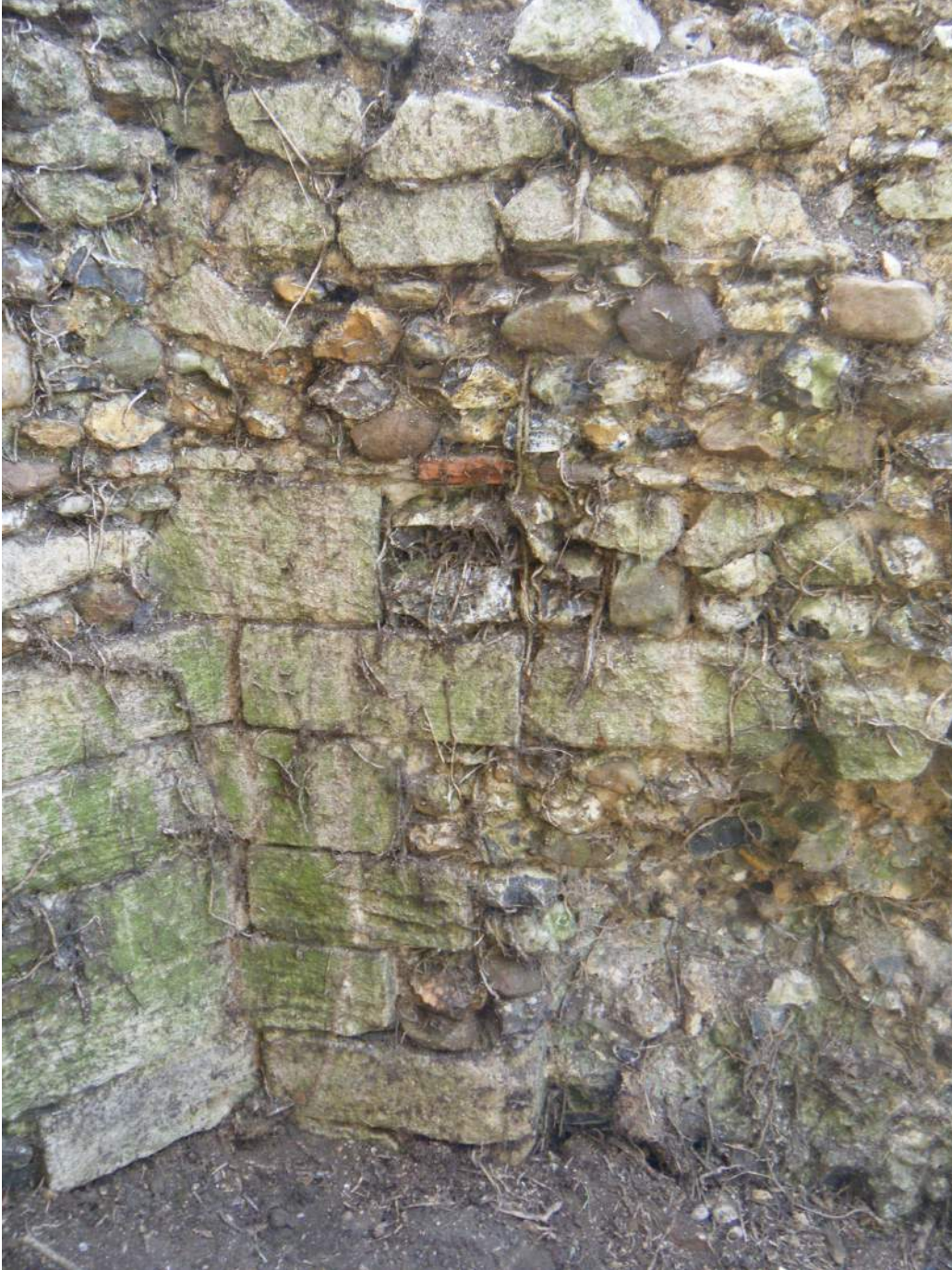
Plate XXVIII Close up of intact facing on south-east interior elevation. Roman tegula visible centre frame.
