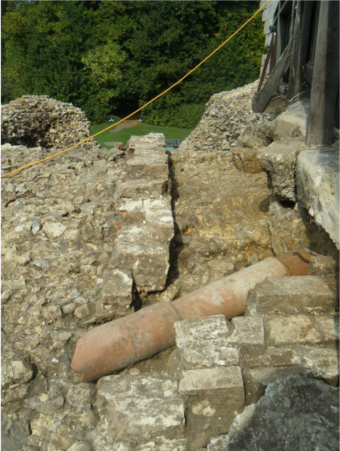
Plate XXXII Drainpipe at top of stairs, with original Norman steps and post-medieval brickwork visible.
