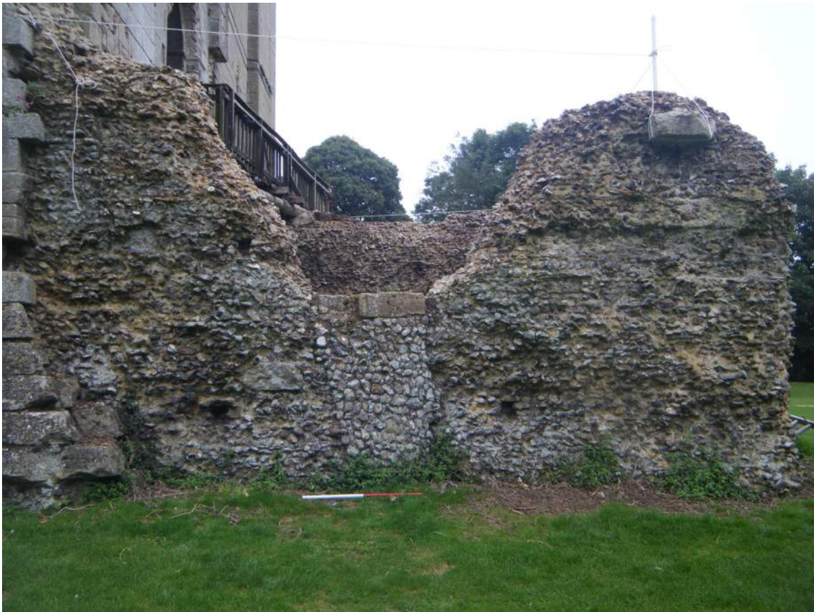
Plate XX North-west elevation of fore-building. Repair visible in centre of wall.
