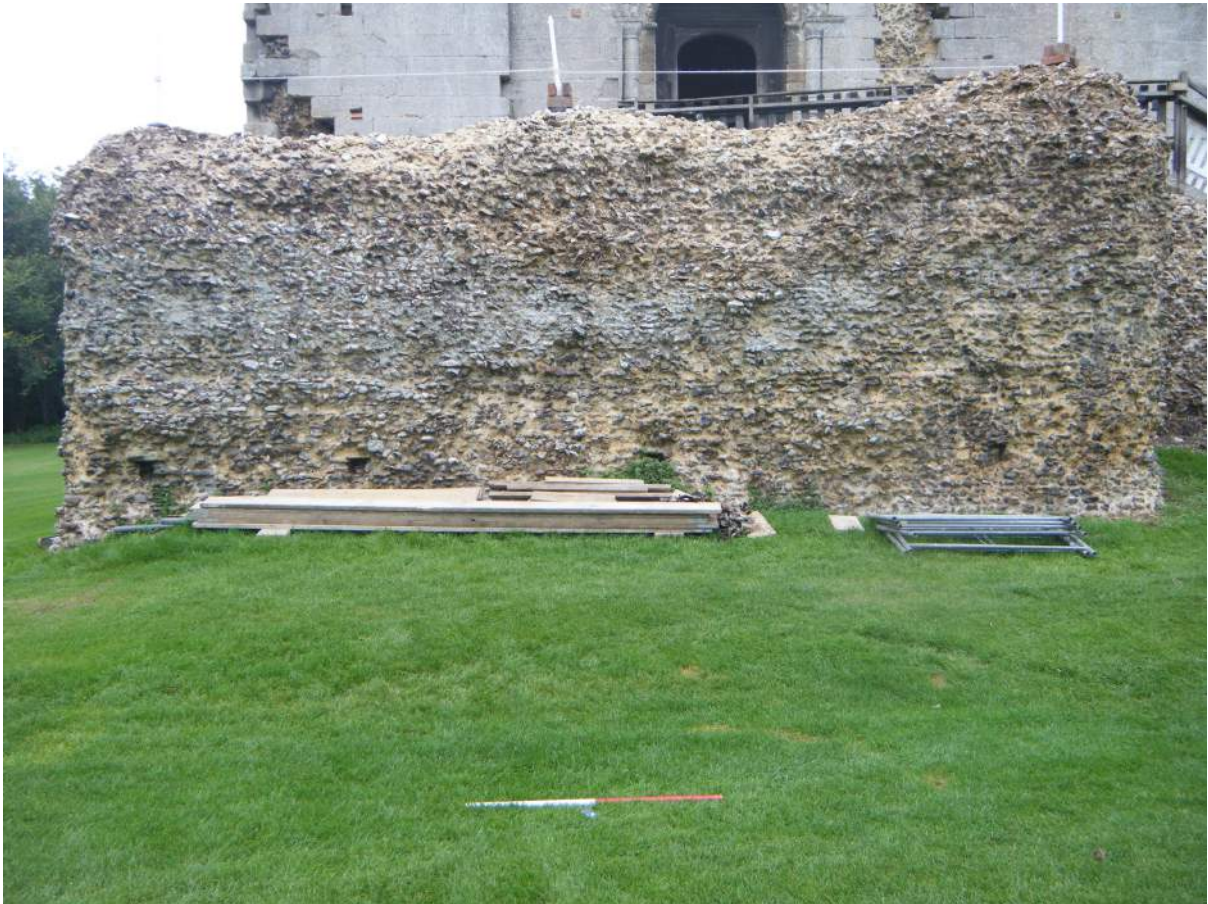
Plate XXII South-west elevation of fore-building.
