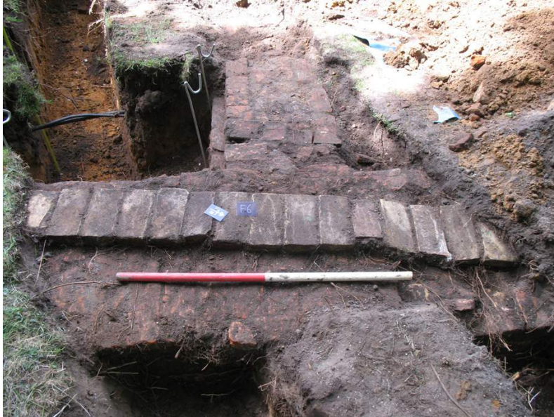
Plate V F6 in T1. View facing south-west. Note the course of lighter pavior bricks.
