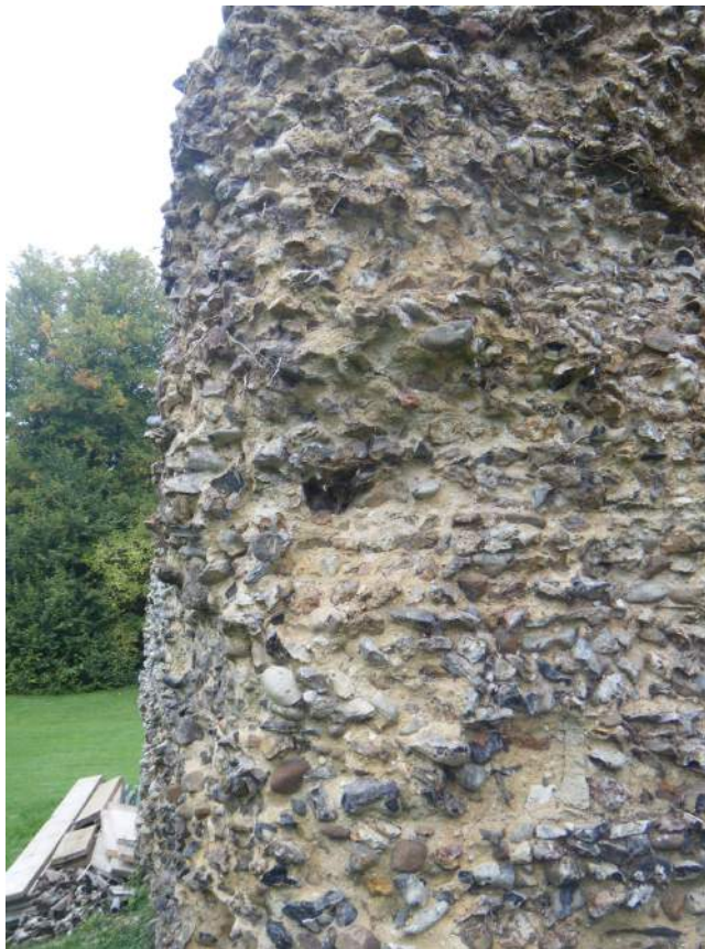
Plate XXV Close up of putlog hole in south-east elevation.
