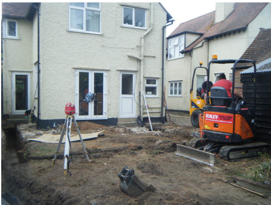
Plate 1: general site show, view NW
