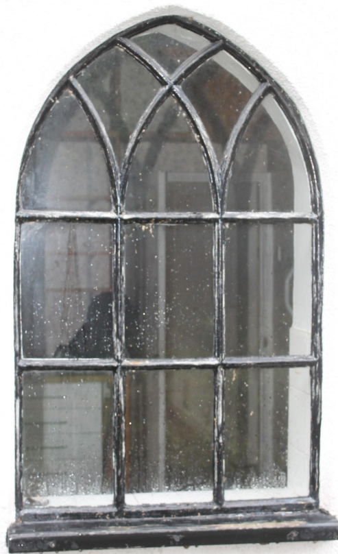
Plate 2 Detail of original timber-framed Gothic Revival window to south-east elevation - view north-west.
