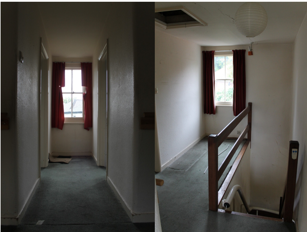
Plate 10 Staggered first floor landings showing 20th-century stairs in reversed position - view north-east and south-west.
