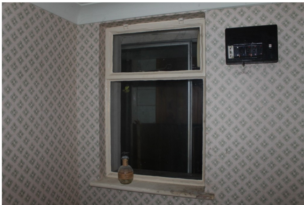
Photograph 15 Replacement Crittall-type metal-framed window to the rear of the main range – view south-west.
