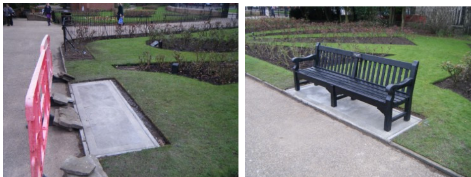
Photograph 5-6 Base slab laid and bench in new position, looking SE
