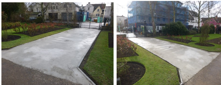
Photograph 11-12 New entrance completed, looking SE and SW
