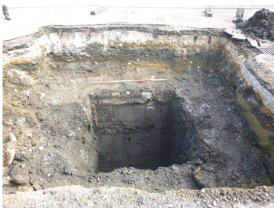
Photograph 3 T1, looking E
