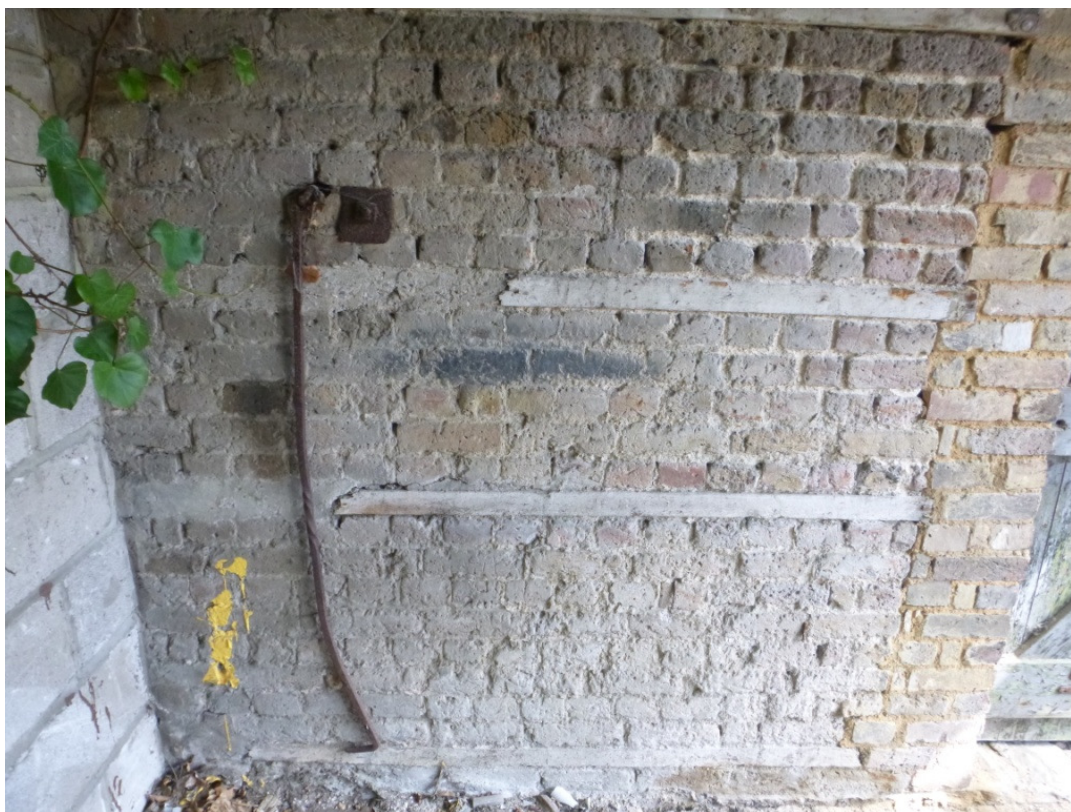
Photograph 12 Original wrought iron cart door retainer mounted on east wall of the west midstrey – view east.
