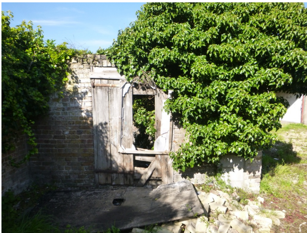
Photograph 10 Original doorway in side wall of east midstrey – view west.
