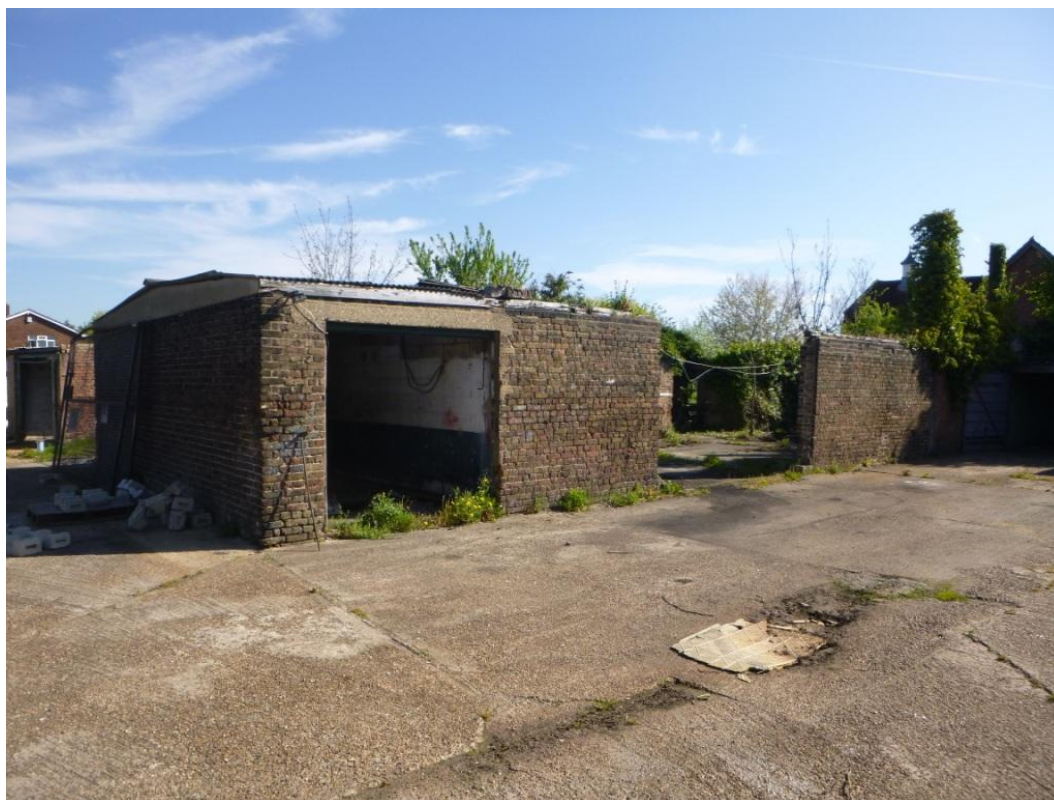
Photograph 8 Building A, west and south elevations with the inserted garage doorway to the left of the shot – view north-east.
