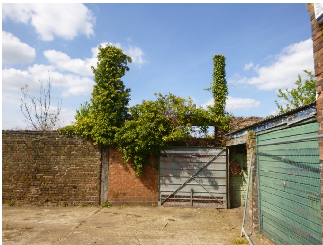
Photograph 9 Infilled cart door opening in south elevation with ivy-covered door posts indicating the original height of the building – view north.
