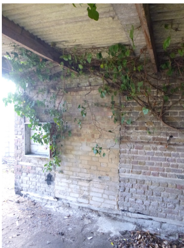
Photograph 11 Infilled original doorway in the west wall of the west midstrey – view south-west.
