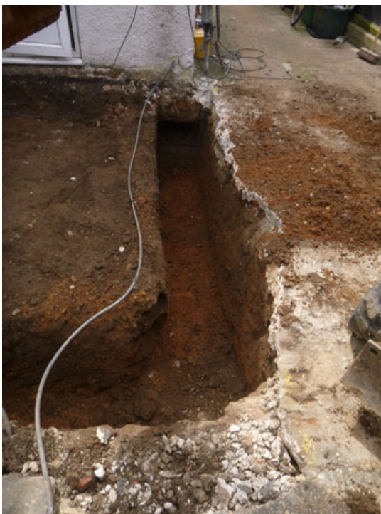
Photograph 2 Foundation trench, looking S
