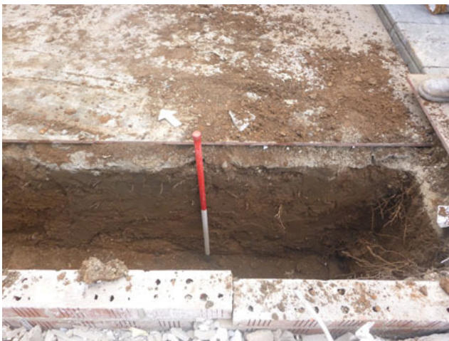
Photograph 2 Foundation trench, looking NE
