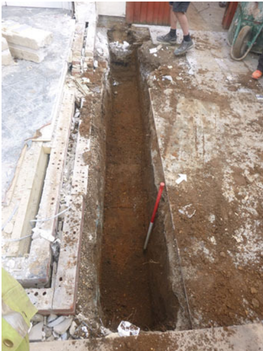
Photograph 1 Foundation trench, looking NW
