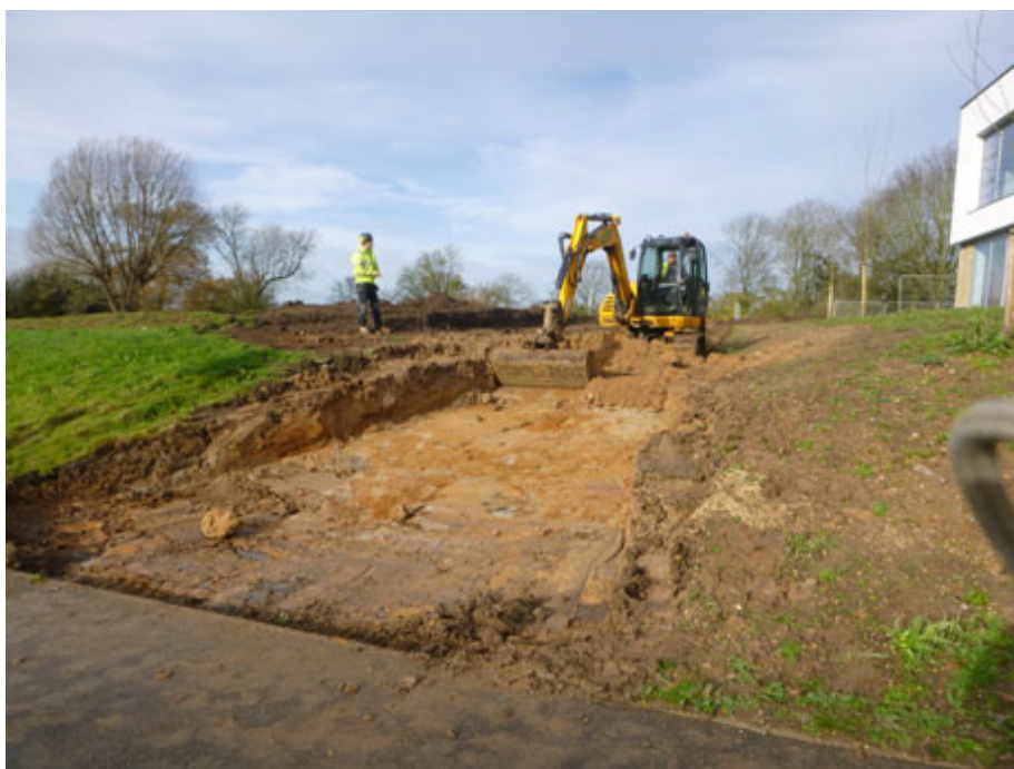
Photograph 1 Excavation of the haul road, looking NW
