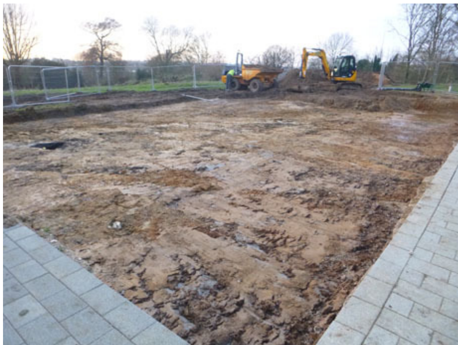
Photograph 2 Area reduction, looking NW
