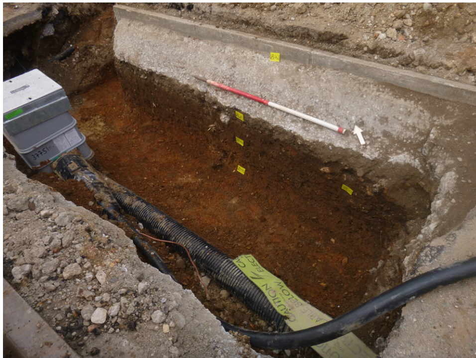
Photograph 1 Service trench, photograph taken facing north.
