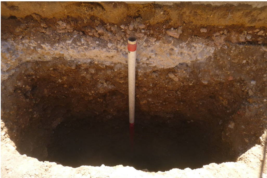
Photograph 4 Test-pit 1, slot through backfill, looking S
