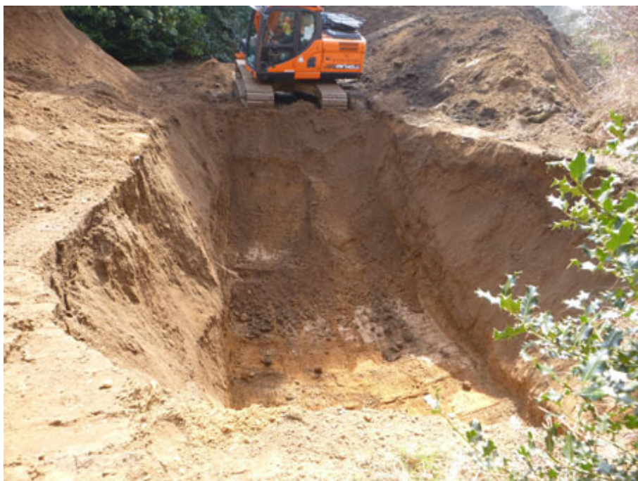
Photograph 5 Soakaway, looking SE
