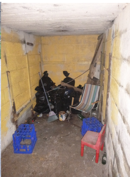
Photograph 12 Interior of the shelter
