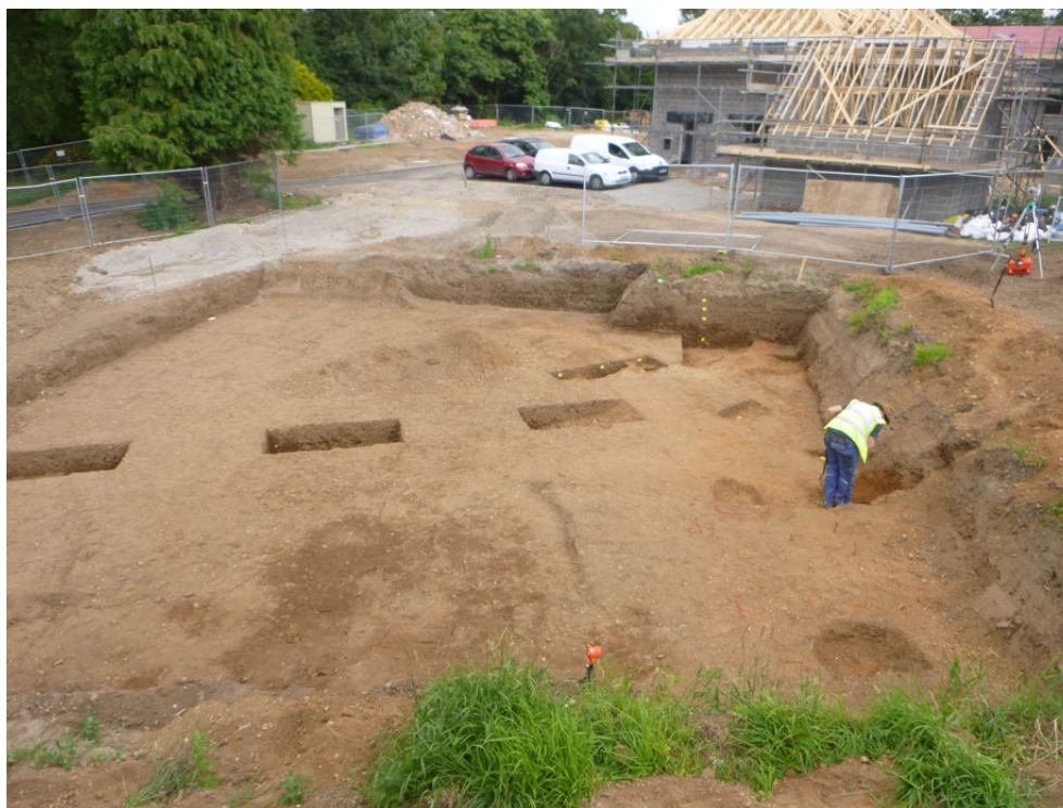
Photograph 3 Plot 3, looking NW
