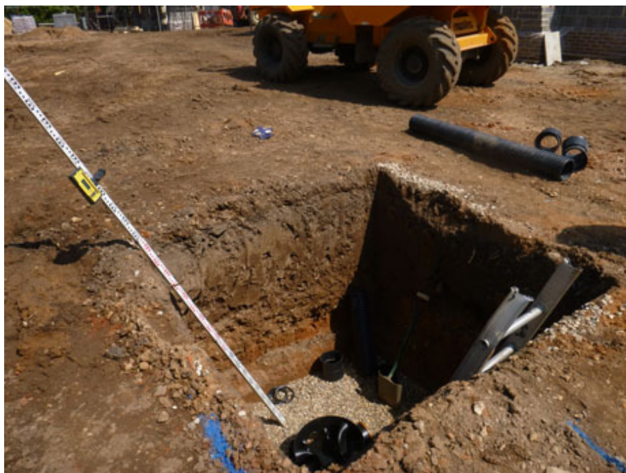
Photograph 6 Manhole 2, looking NE
