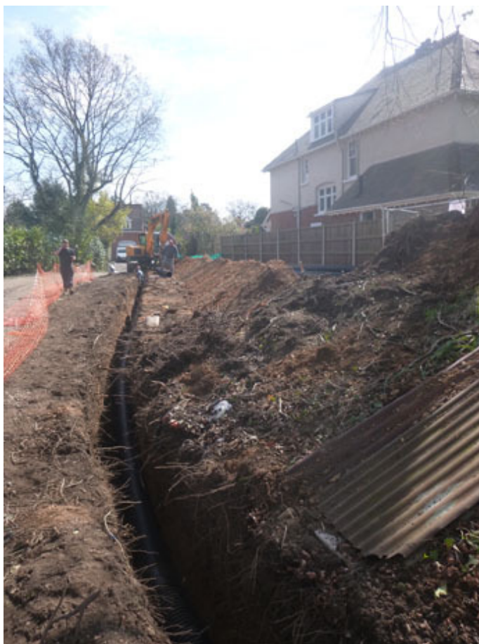
Photograph 4 Service trench, looking E
