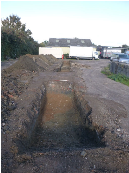
Photograph 1 T1, looking N
